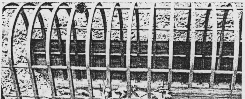
Arches and reject steel mats form tunnel structure.
