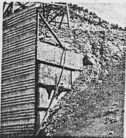
Retaining walls at each end of tunnel were constructed with old mine cars filled with earth material.
