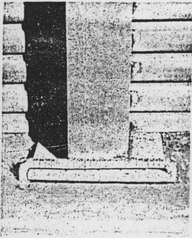
Flanges of arches were slipped under reinforcing bars set in concrete.
