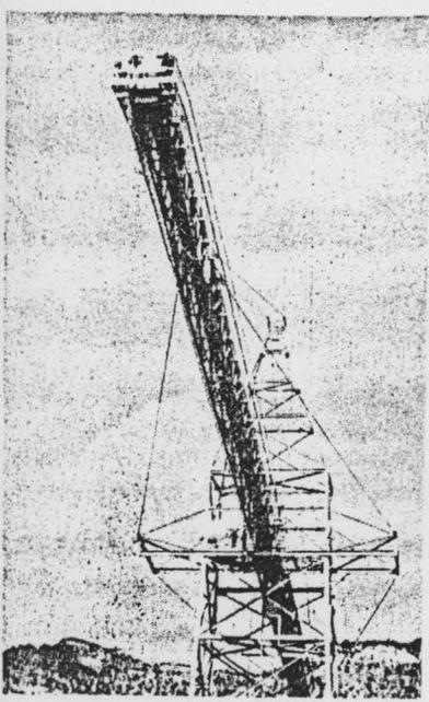
Coal, elevated 120 ft, discharges onto the 456-ft-diameter storage pad.
