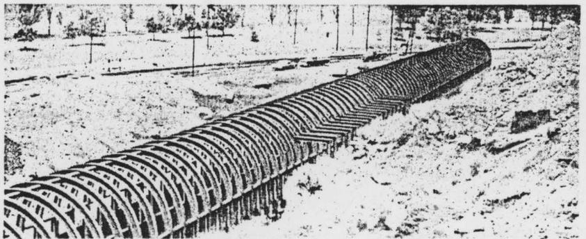
Tunnel is 456 ft long with control room in center. Structure is covered with approximately 10 ft of earth material.
