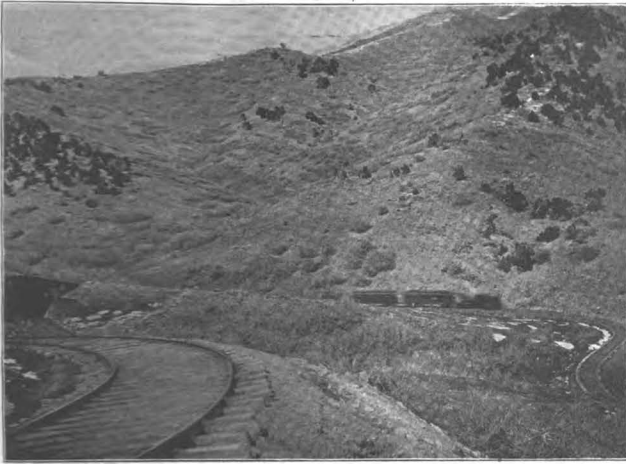
VIEWS ON THE SALT LAKE & MERCUR R. R. IN UTAH. MAXIMUM GRADE, 4.2%; SHARPEST CURVE, 42°. ELEVATION OF 1,986 FT. ATTAINED IN A DISTANCE OF 9.58 MILES.
