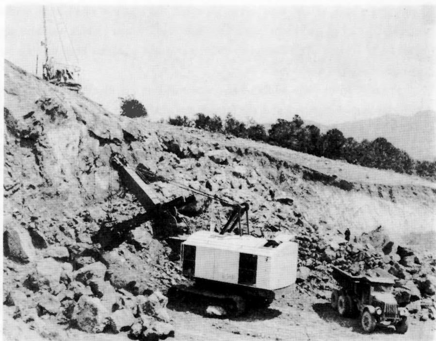
OPEN PIT MINE AT IRON MOUNTAIN, SHOWING SHOVEL AND BLAST HOLE DRILL
