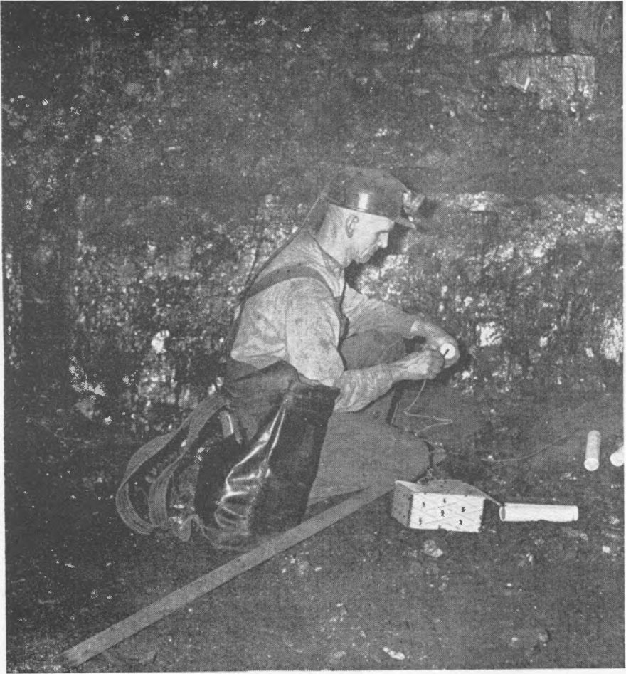
Loading holes with explosives preparatory to blasting. Joe Otterstrom, tamper.
