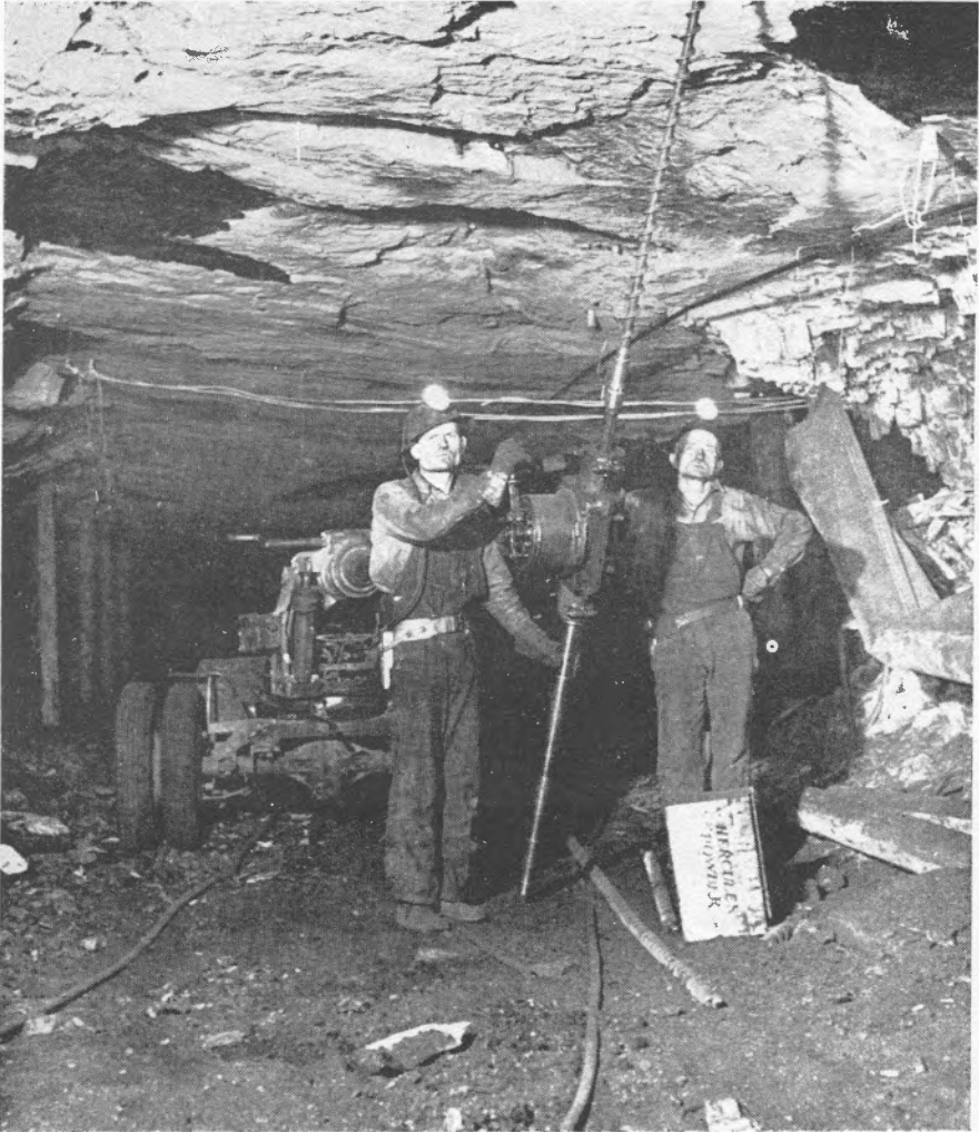
George Rogers and Roy Barkley, drillers, set up to drill top coal.
