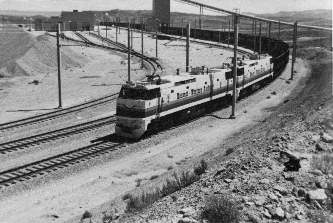
Top, loading operations at Deserado. Both E60's pull the unit train under the coal silo as the coal pours aboard for its 37 1/2-mile train ride. The engine-house can be seen at the left. The lower picture shows the sweeping curve of the conveyor to the top of the silo, as the train approaches. The author rode this trip in August 1984.
