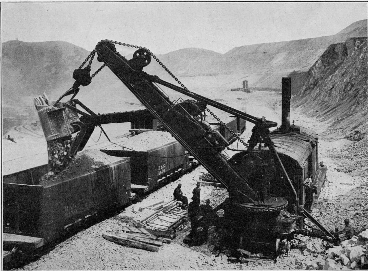
STEAM-SHOVEL LOADING ORE INTO RAILROAD-CARS
