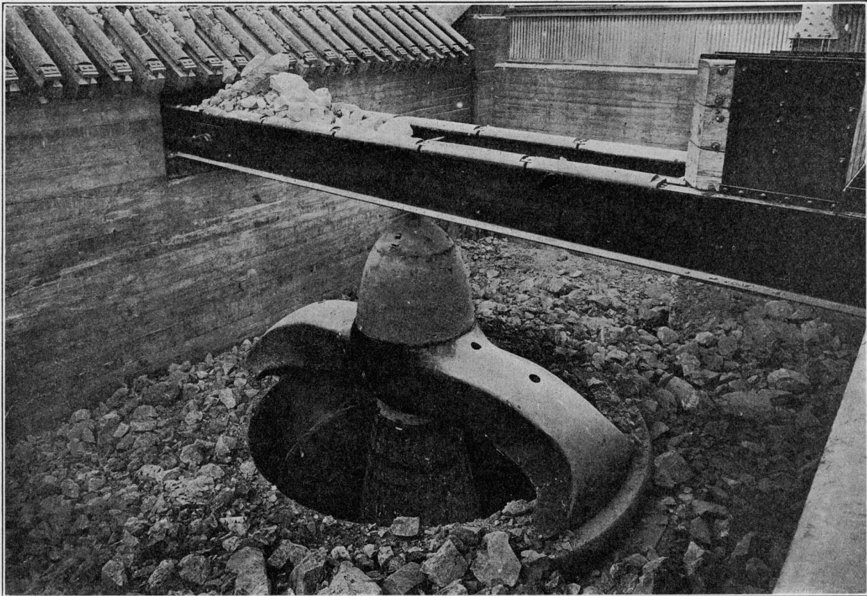
FIG. 5. GYRATORY CRUSHER, AND LOWER END OF GRIZZLEY
