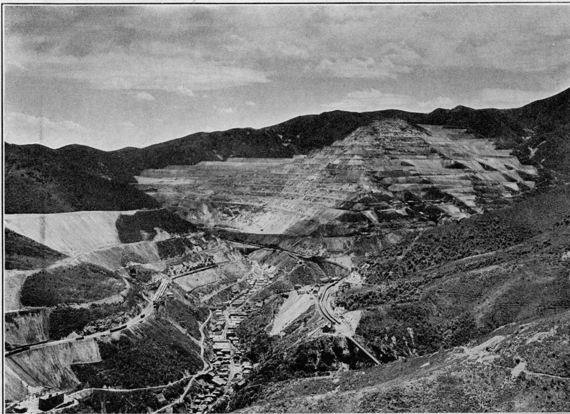
GENERAL VIEW, SHOWING THE TOWN OF BINGHAM IN THE FOREGROUND, THE UTAH COPPER MINE IN THE BACKGROUND, AND THE BINGHAM & GARFIELD RAILROAD IN THE CENTRE. THE WHITE DUMP ON THE LEFT IS PART OF THE OXIDIZED ORE OF THE 'CAP'; THE TERRACES EXTENDING AWAY FROM THE MINE WORKINGS ARE DUMPS OF 'STRIPPING', OR WASTE ROCK, IN GALENA GULCH, ON THE LEFT, AND IN INGERSOLL GULCH, ON THE RIGHT.
