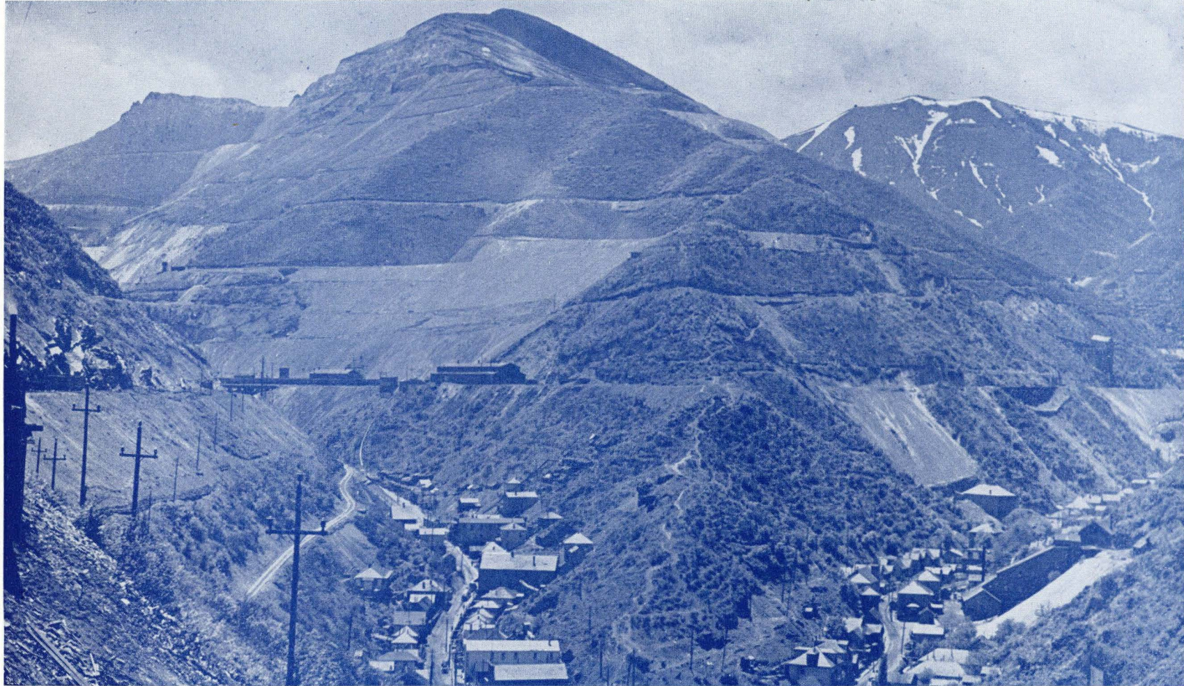
By 1909, the pattern of the first few levels on the mountain had been established. Utah Copper operations are the lower ones; the levels near the top of the mountain were cut by the old Boston Consolidated Mining Company.
