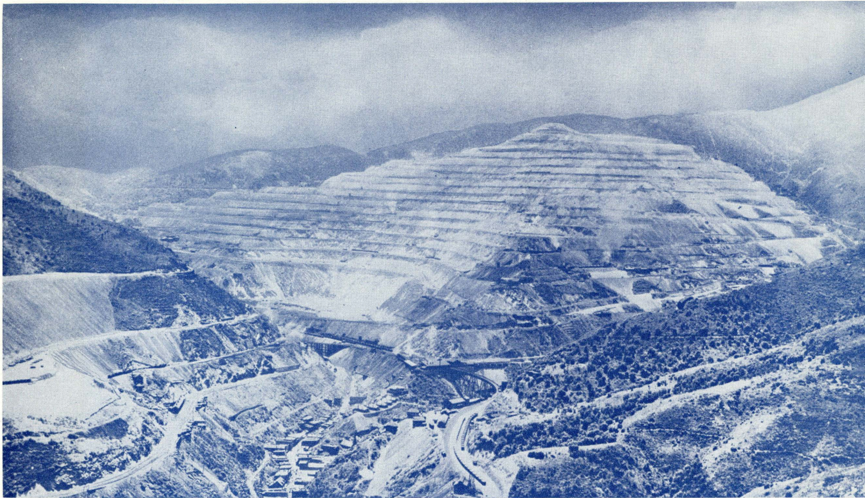
By 1919, the entire face of the mountain was cut into benches. Underground mining had ceased by this time, and all ore was being obtained from surface operations. Waste dumps were located on both sides of the mine.
