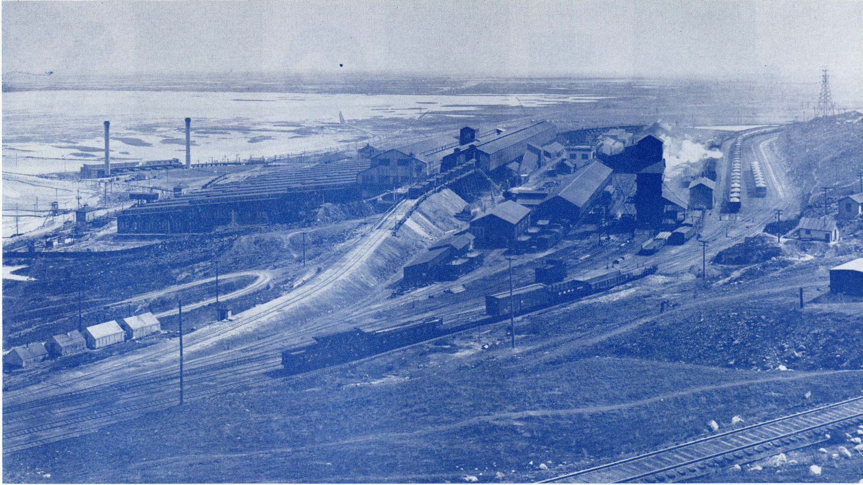
Utah Copper's Magna ore concentrating mill about 1915. At this time, experiments with the flotation process of metal recovery were being conducted. These and other experiments resulted in a far greater percentage of metal recovery.
