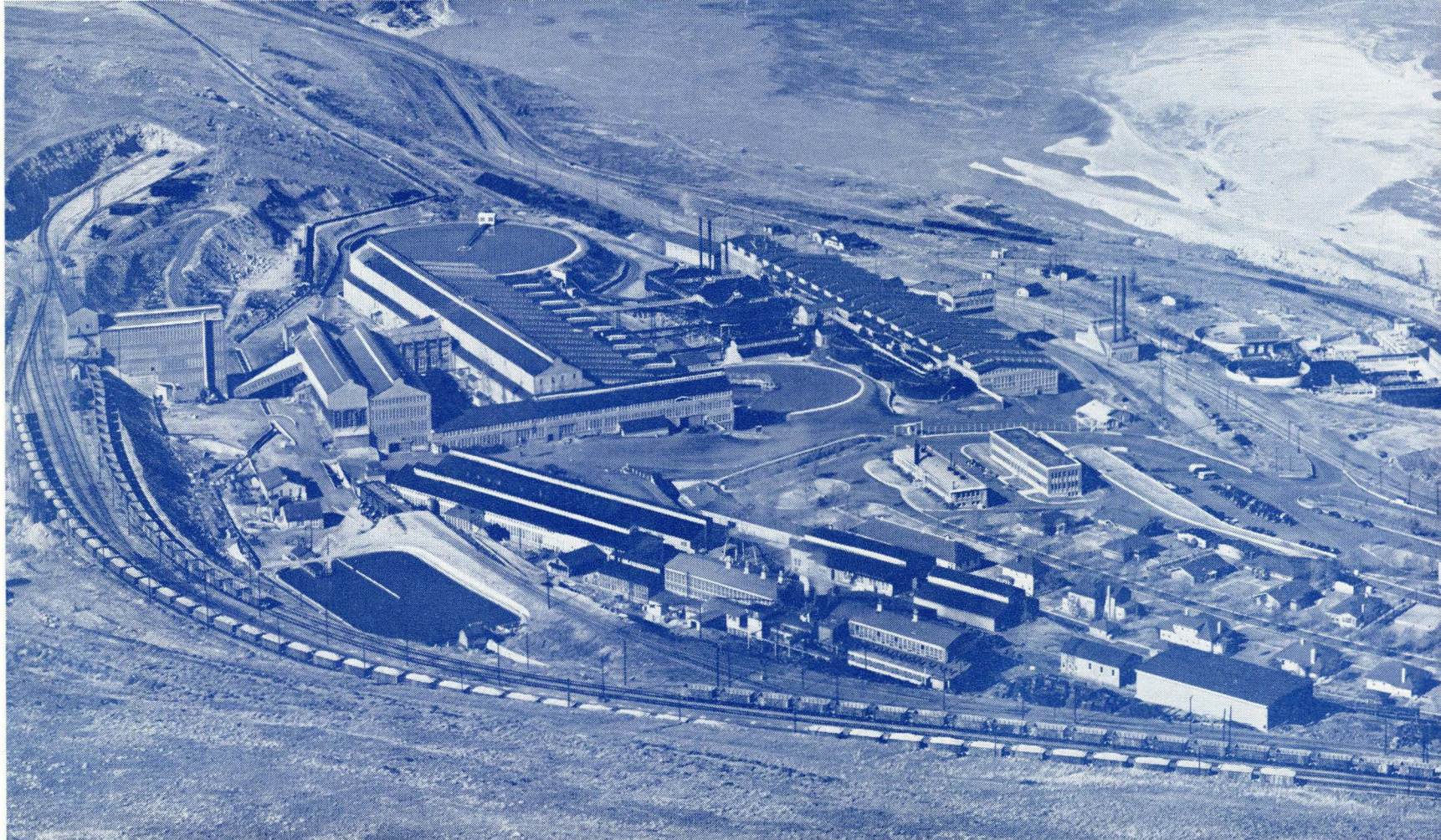
A recent view of the same mill. It has a normal capacity of 40,000 tons of ore per day. Both the Arthur and Magna mills exceeded this tonnage during World War II and again during the fighting in Korea.
