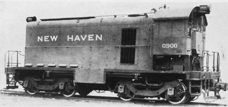
Left: The first Alco shunter to be equipped with the then new 600 b.h.p. Alco/McIntosh & Seymour engine with six 12½ in. by 13 in. cylinders, 1931
