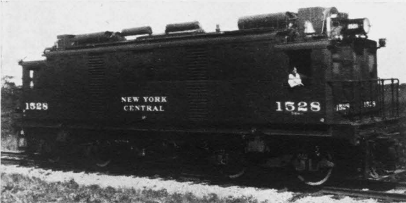
Above: Two - power diesel-battery locomotive of the New York Central; the N.Y.C. also had 35 three-power units with third-rail shoes for 600-volt d.c. (1931)
