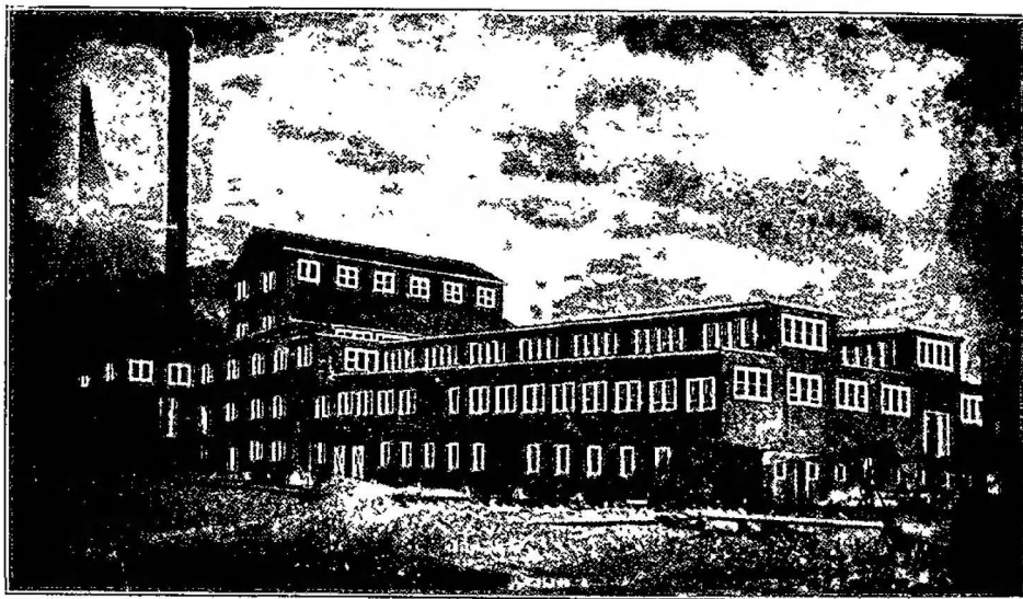
View of Newhouse Mill from the Northwest
