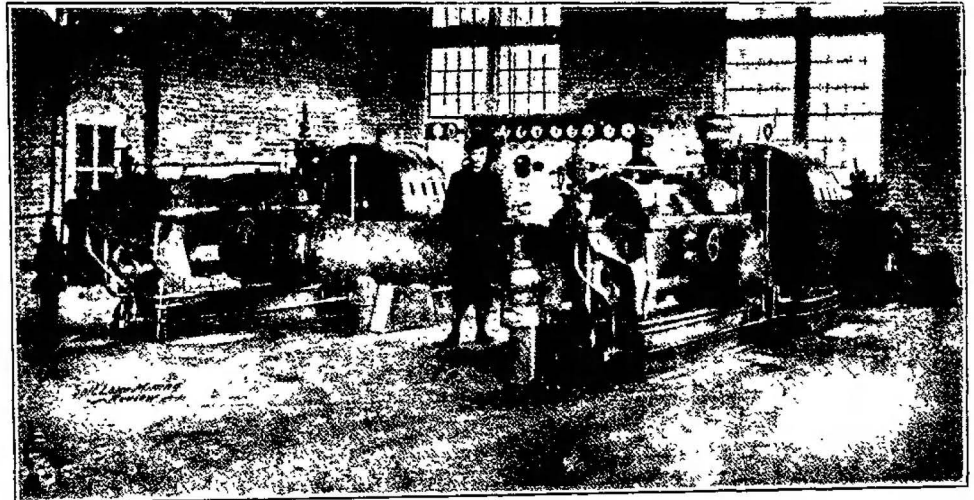
View of Turbine Units and Switchboard
