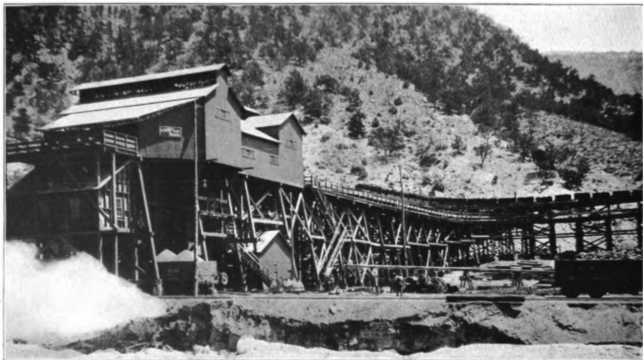
Sunnyside Crusher Plant and Bridge.
