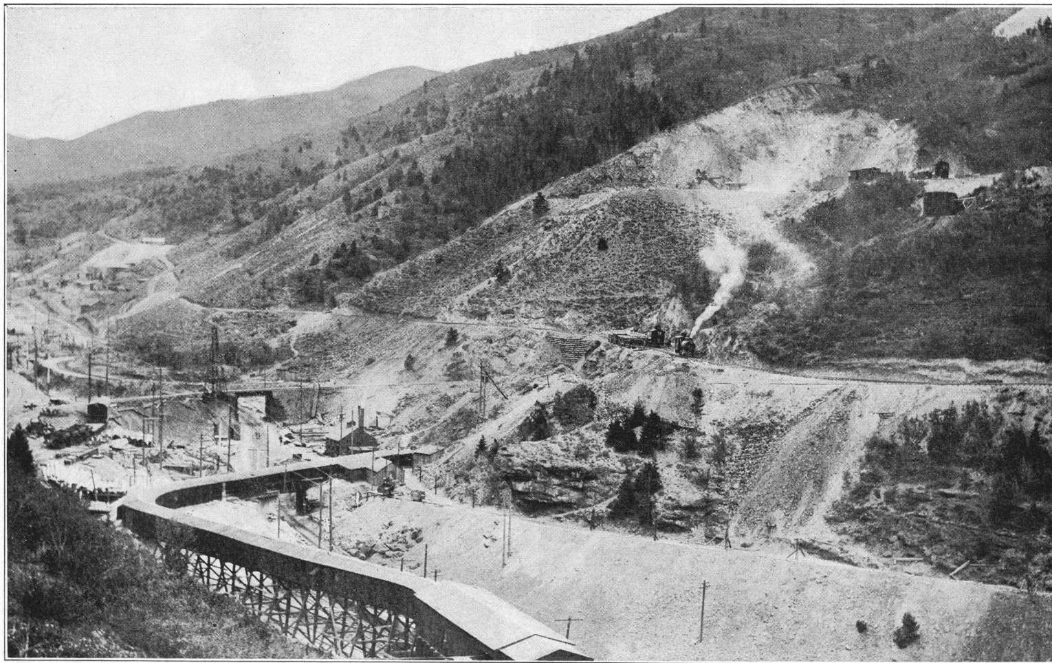
View of Utah Copper in August, 1906, When First Steam Shovel Was Started.
