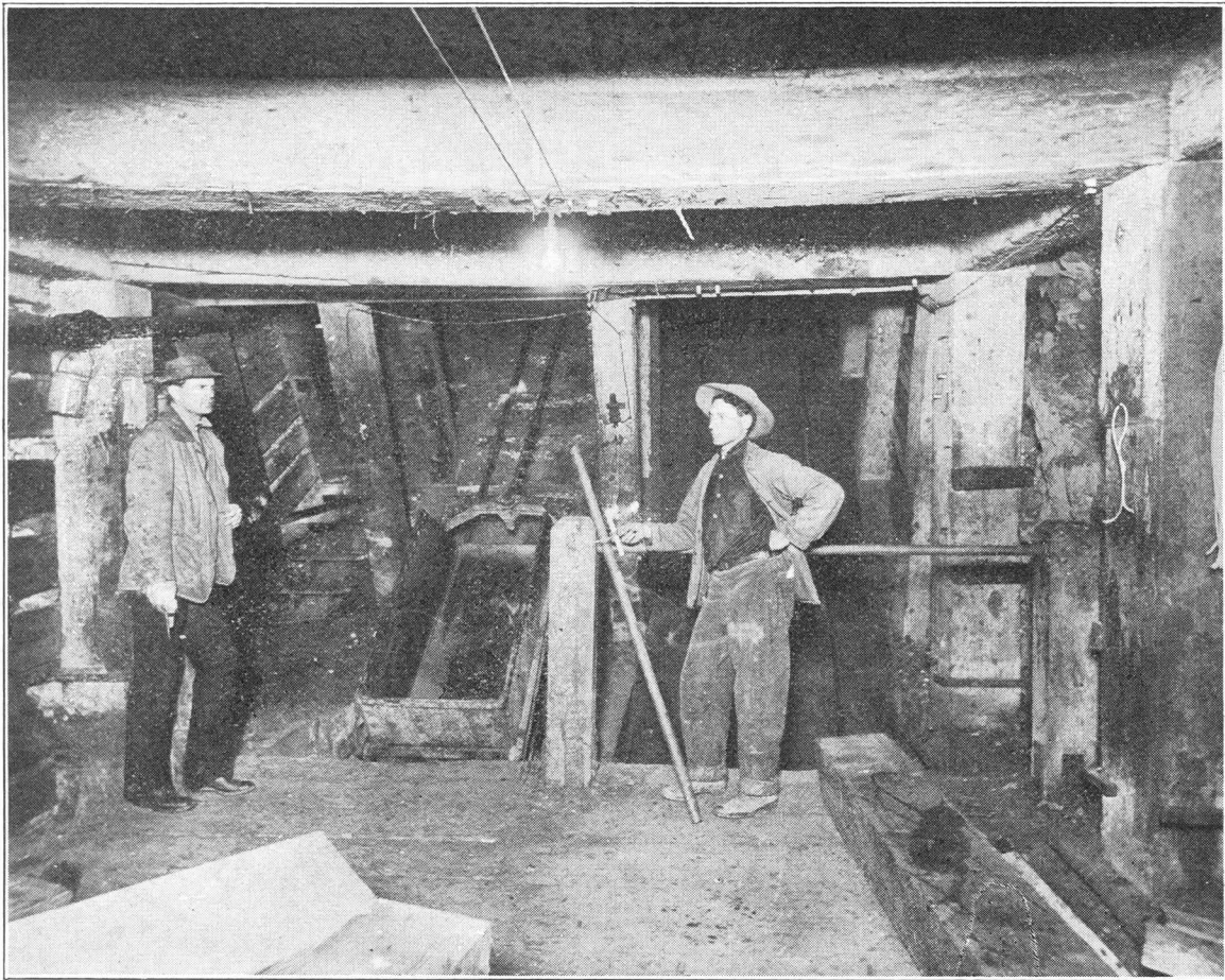
Station at Twelfth Level. Yampa Mine.
