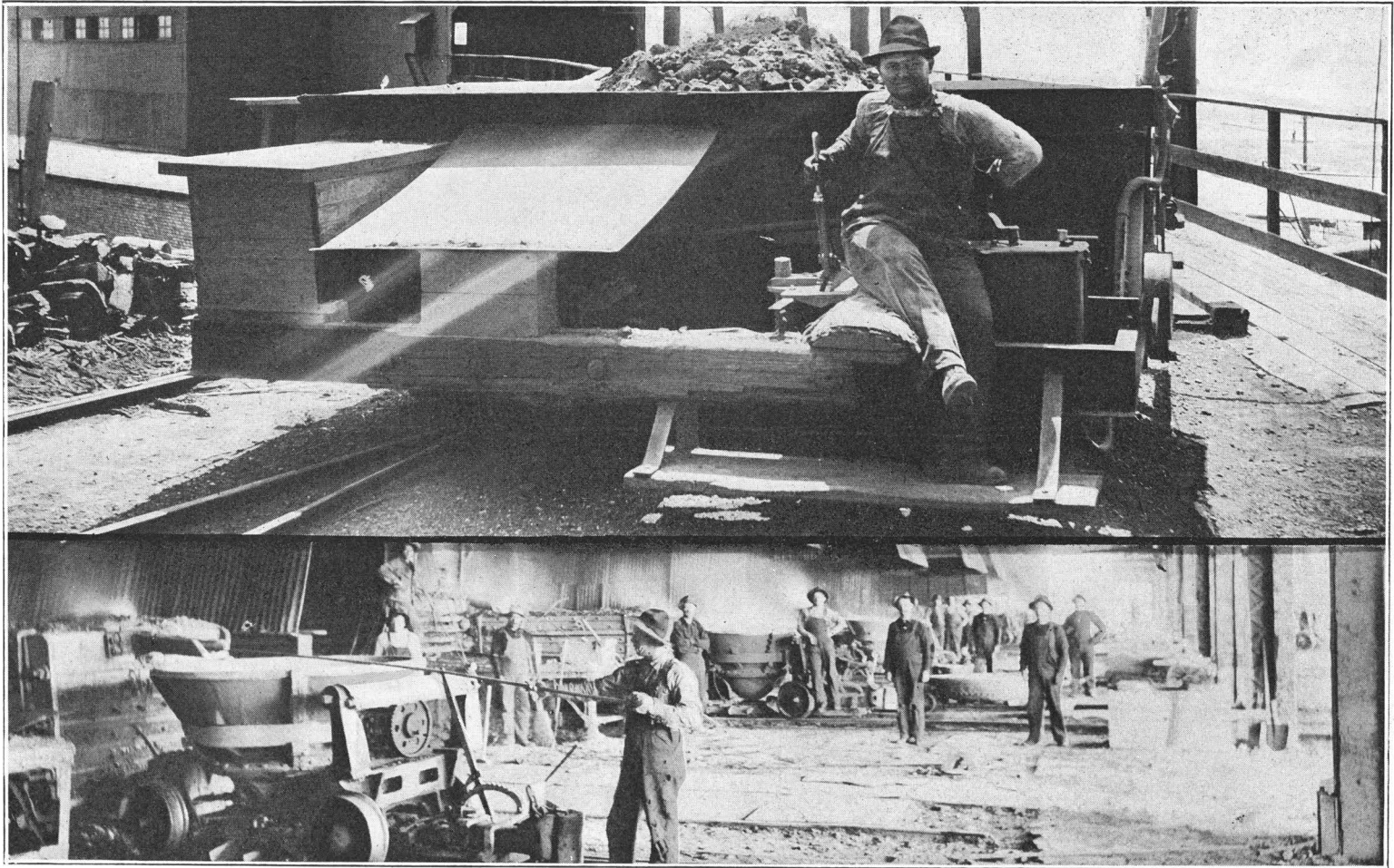
View of a charge car at the U. S. Smelter, with its load of miscellaneous ores, on its way to the feed floor where it is discharged into the blast furnaces. Tapping the lead furnaces in the blast furnace building of the U. S. Company's mammoth smelter. The slag is being tapped into cars and hauled to the slag dumps. The metal is tapped from the sides of the furnaces and settlers and is cast into bullion in an adjoining building.
