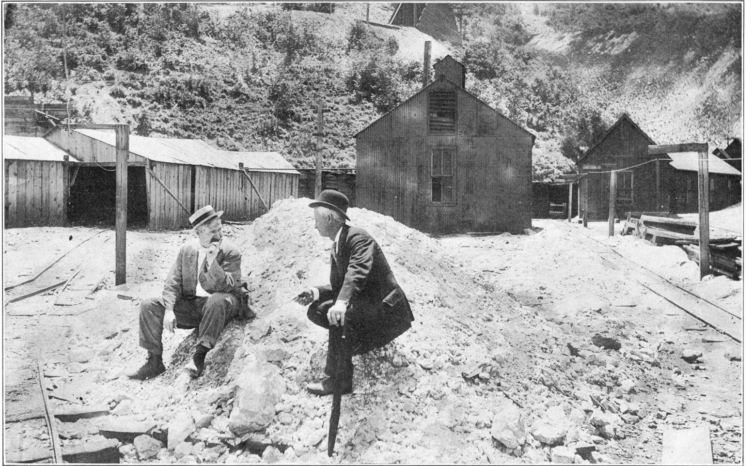
Tunnel Entrance—Silver Shield Mining Company.
