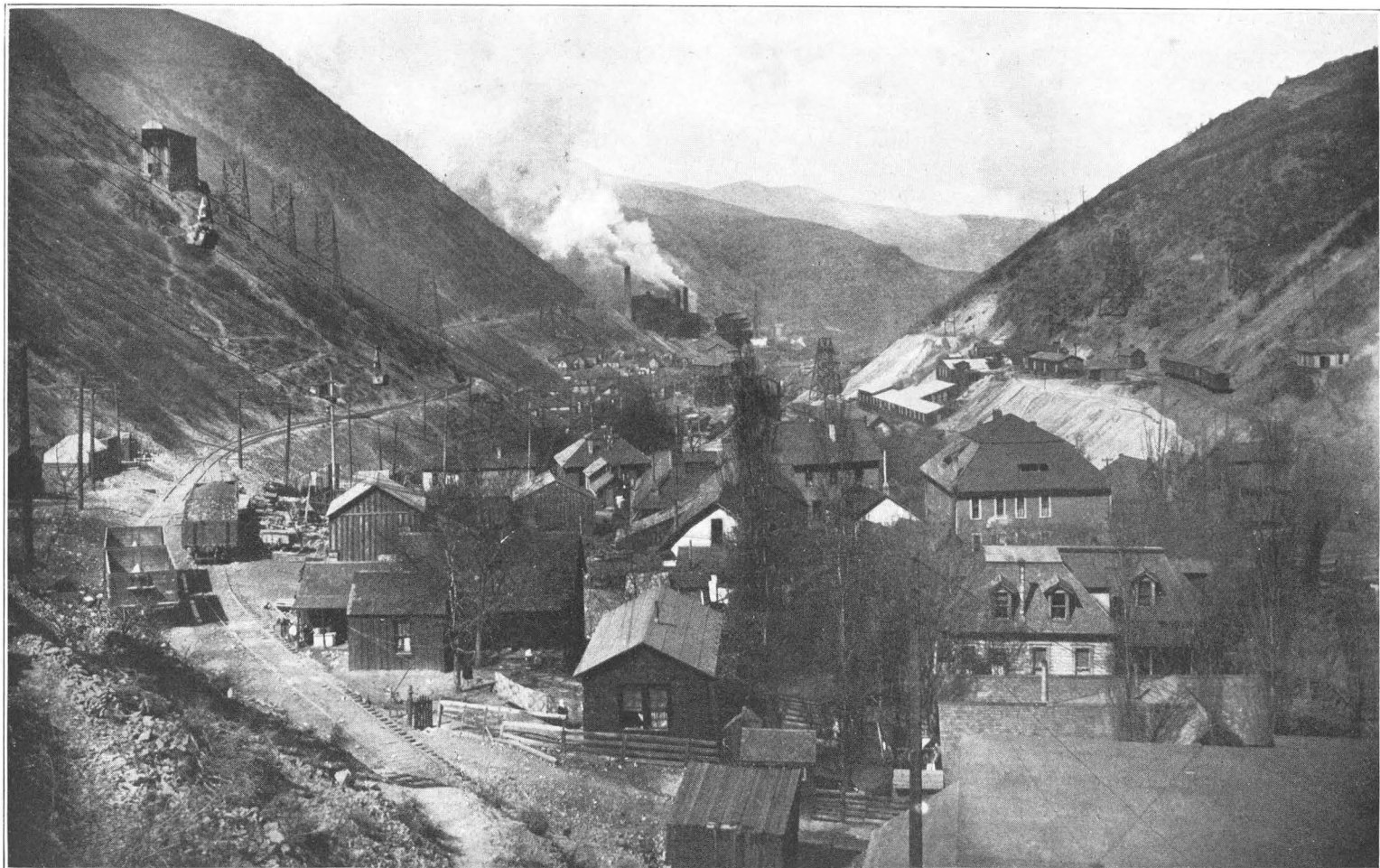
Bingham Canyon, looking down from Copper Belt Trestle at Bingham Butte Mine. Showing Yampa Smelter and Winnamuck Mill
