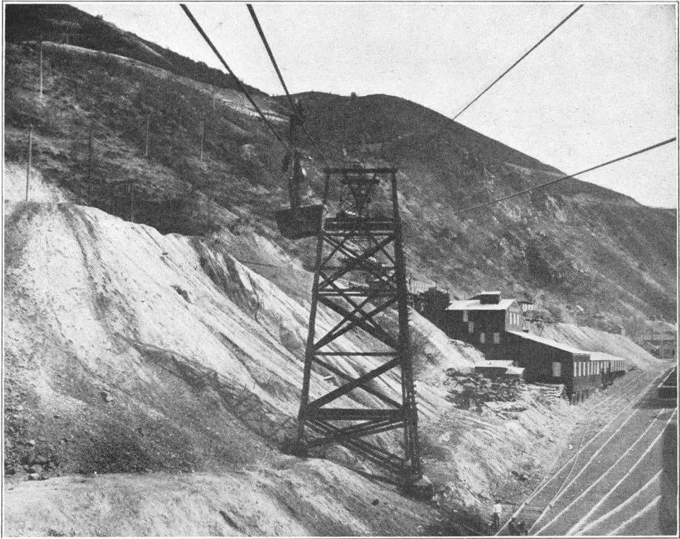
Section view of United States Co.'s aerial tramway on which the ore is conveyed in buckets to the railway station at Bingham, where it is loaded into cars for the company's smelter in the valley. Hundreds of tons of ore are daily forwarded over this line.
