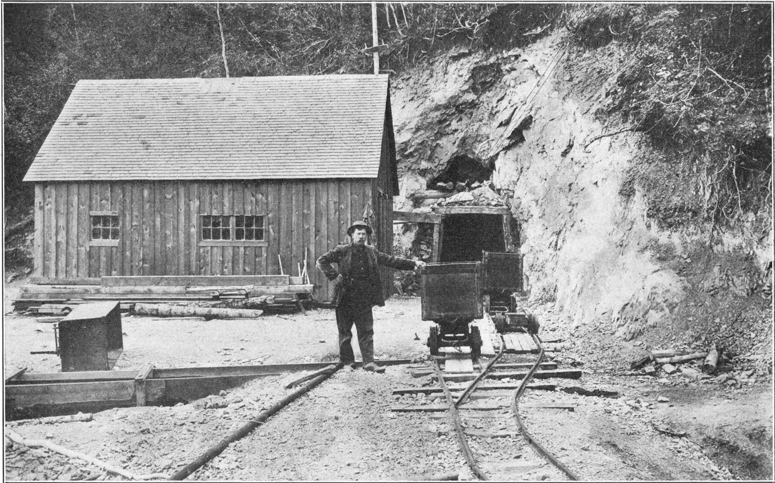
Tunnel Entrance—Utah Metal Property.
