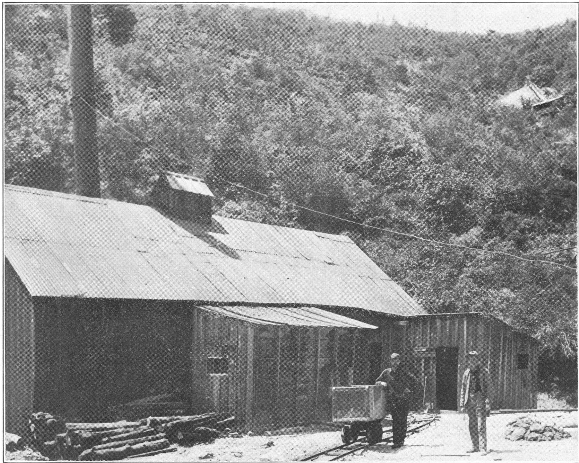
Giant Chief Shaft House—Utah-Bingham Co.
