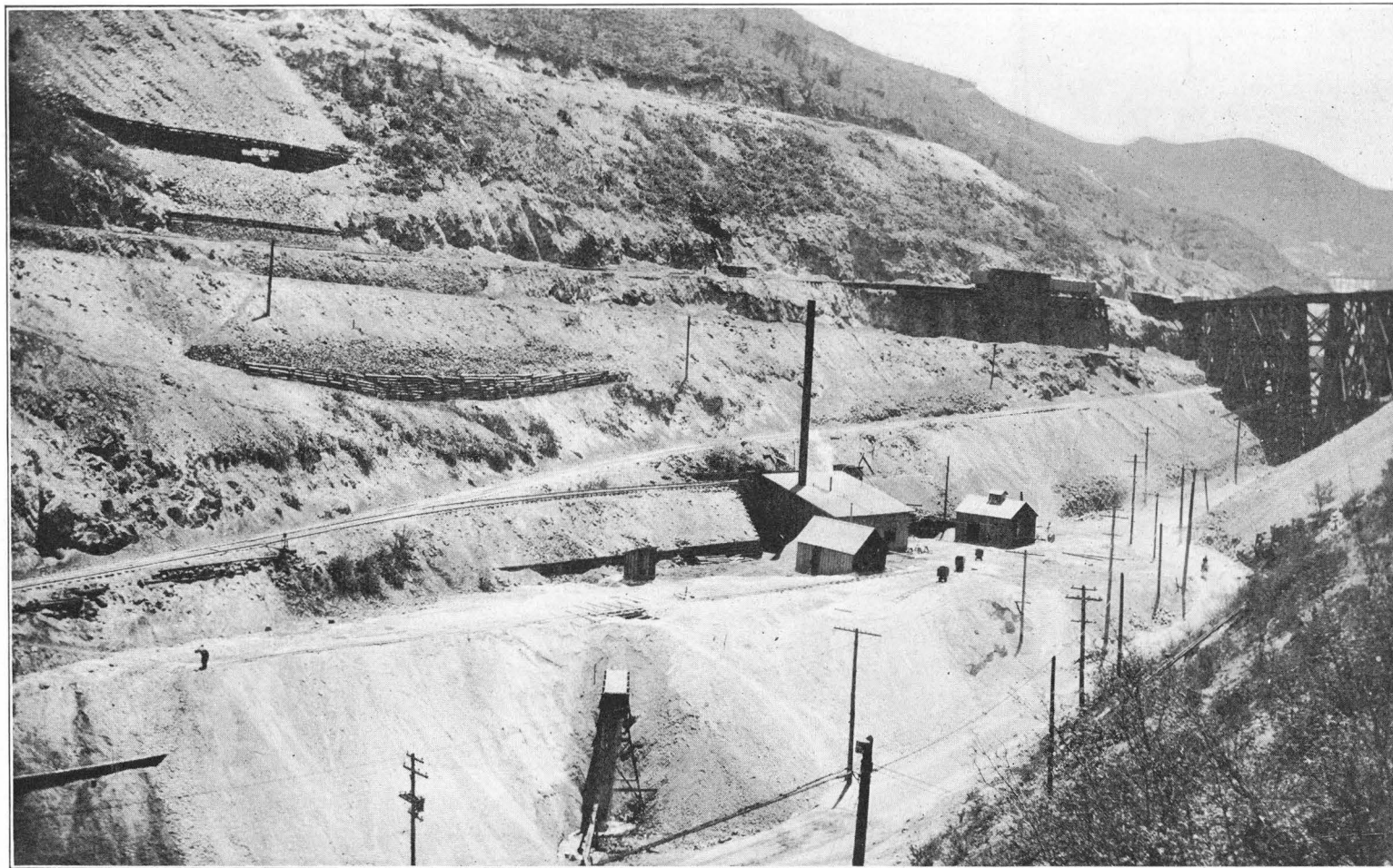
The Starless Group—Air Compressor and Tunnel Entrance. R. G. W. Trestle at Utah Copper Mine.
