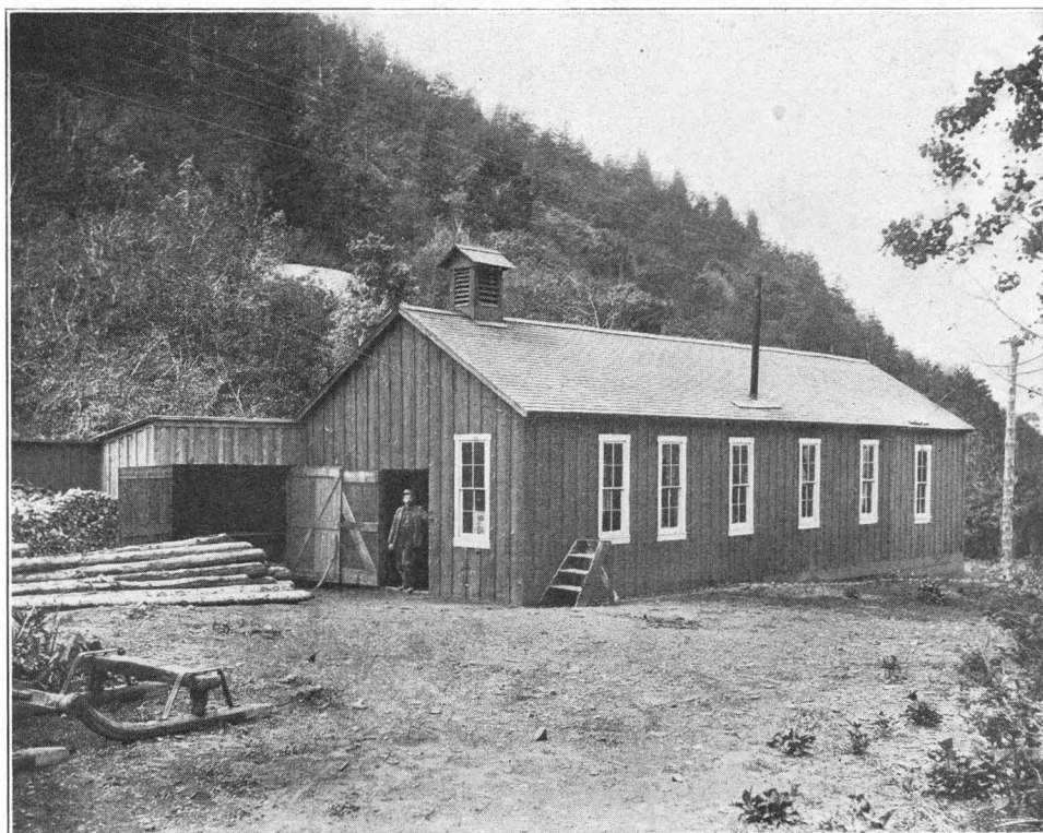
Interior and Exterior Views of Utah Metal Compressor Building.
