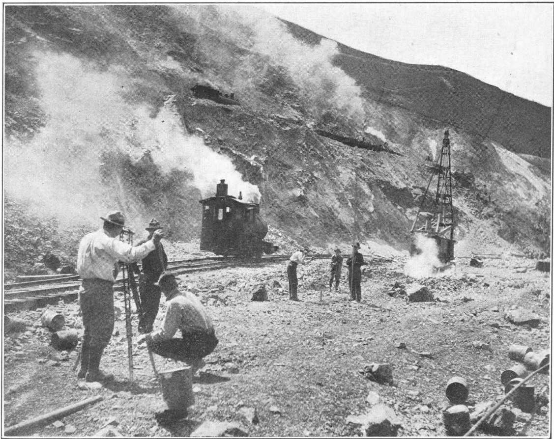
Views at the Utah Copper Mine.
