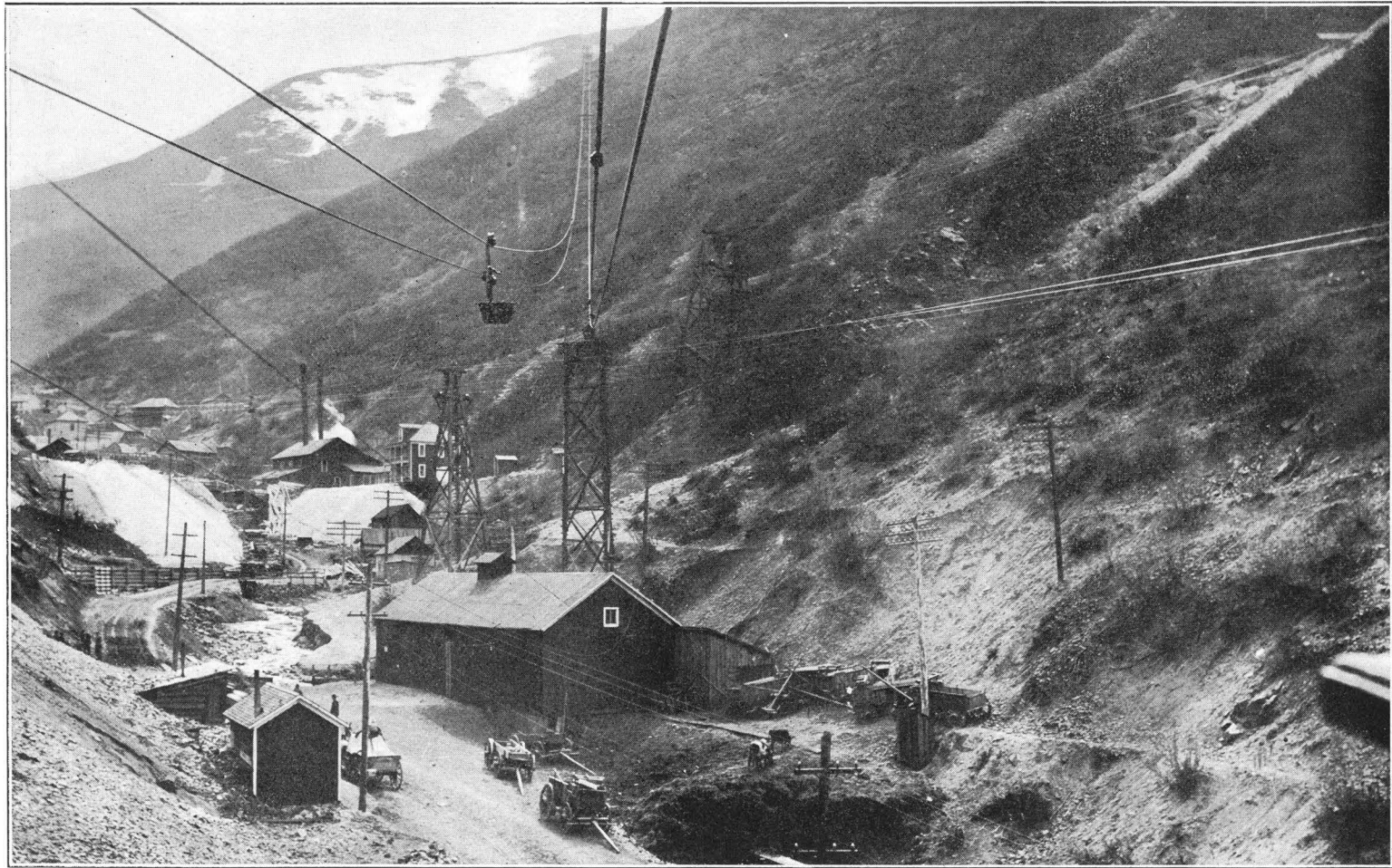
General View of the Utah-Apex Properties. Utah-Apex Tramway crossing Utah-Con. and Yampa Tramways.
