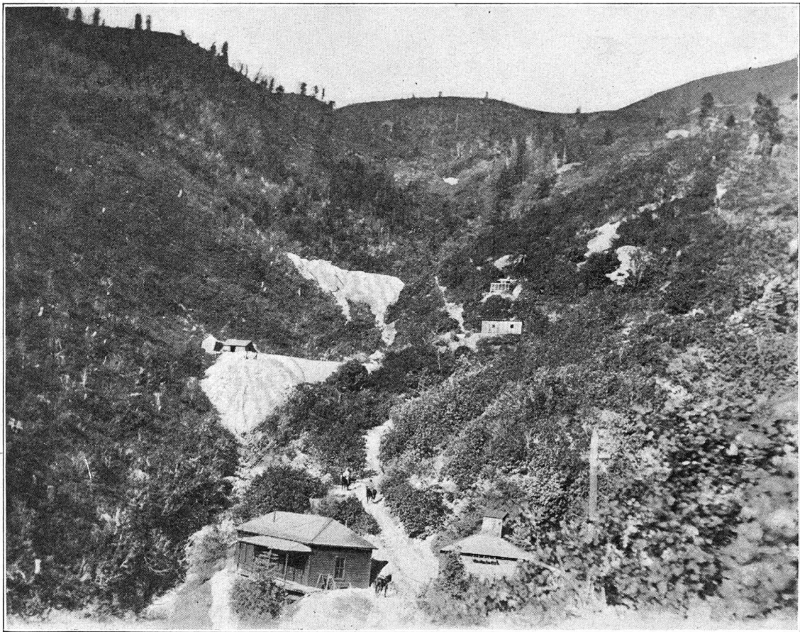
Cottonwood Gulch, Compressor and Office Building of Bingham Copper Company and Dumps of the Caromondel and the Petro Tunnels (now Utah Apex).
