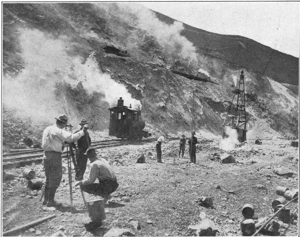
Views at the Utah Copper Mine.
