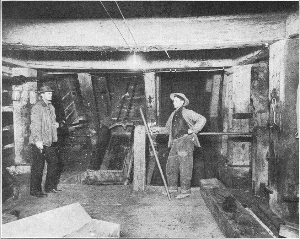
Station at Twelfth Level, Yampa Mine.
