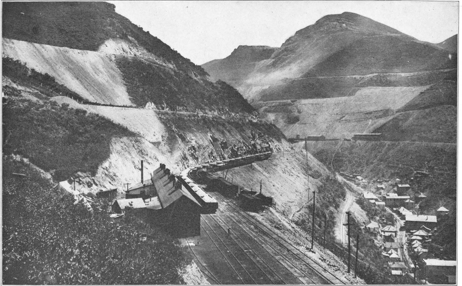
Cuprum—R. G. W. assembly yards and round house on High Line above the town. Utah Copper lines farther up the mountain—Utah Copper and Boston Con. properties in the distance.
