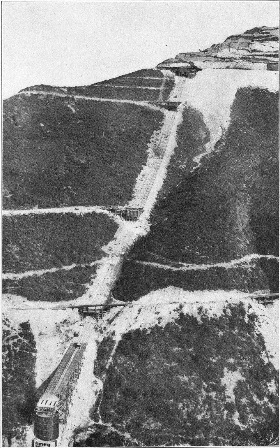
Boston Consolidated Gravity Tramway—Ore Bin at the Base.
