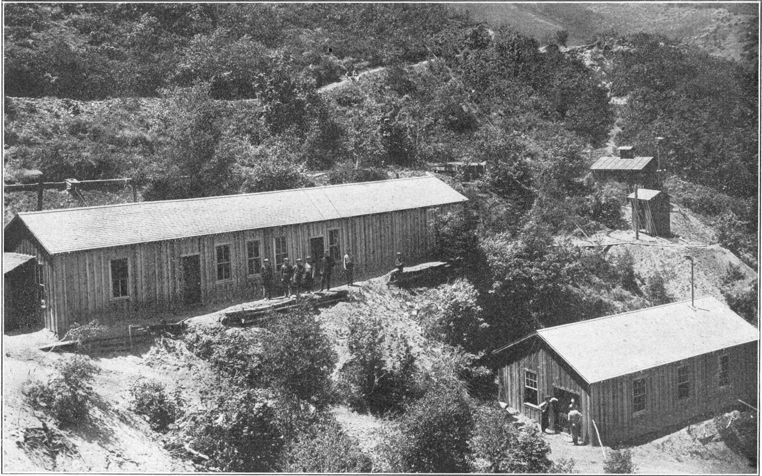
Utah-Bingham Compressor and Boarding House.
