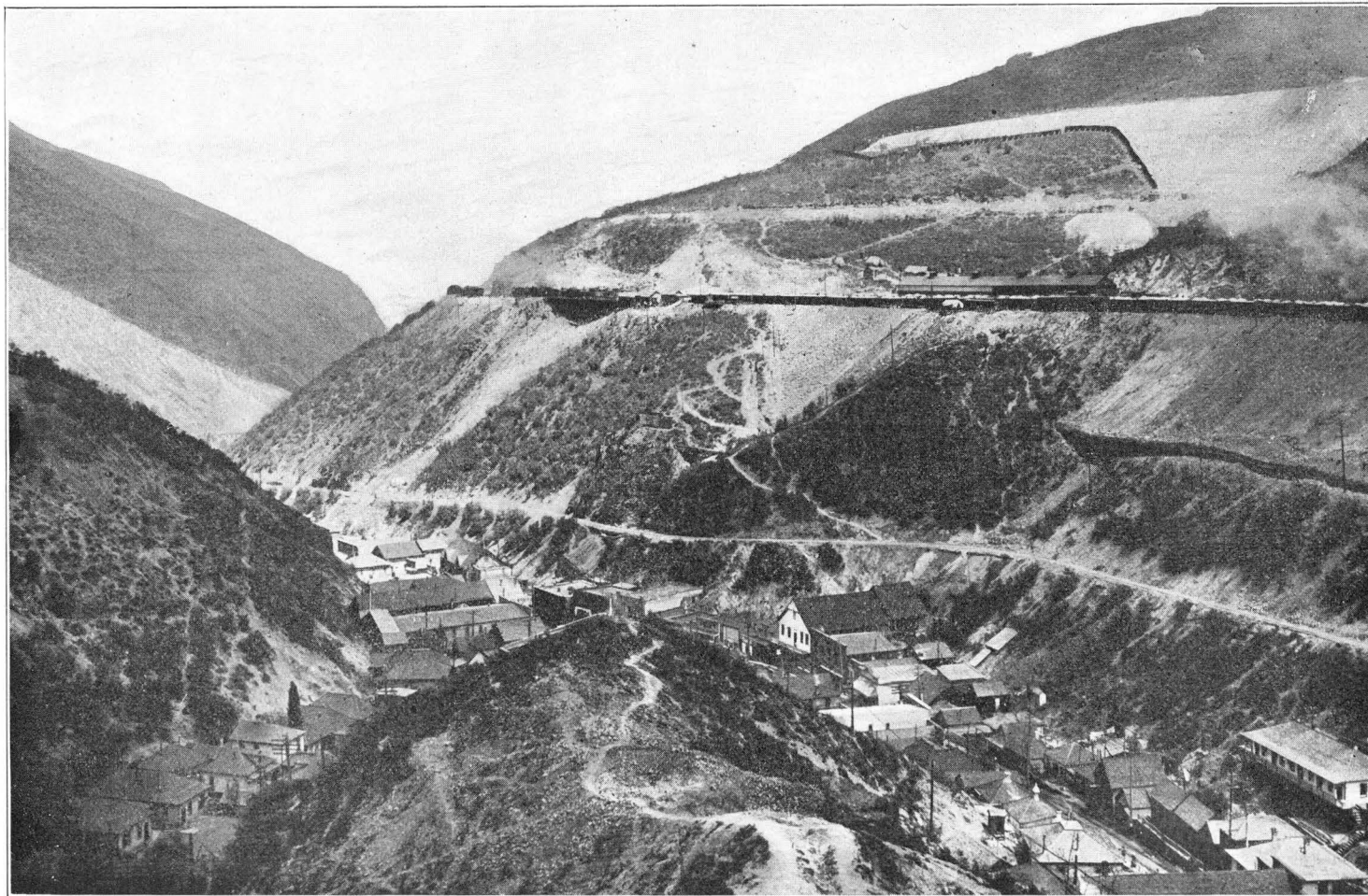
Looking down Bingham Canyon, Copper Belt R.R. just above buildings, R.G. W. High Line above, and two lines of Utah Copper Co.
