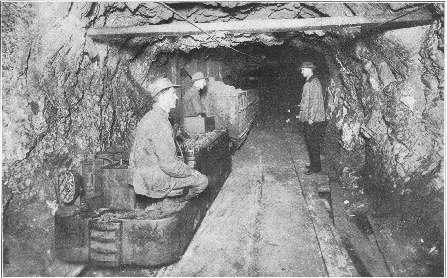
Electric locomotive with six three-ton cars, loading from No. 2 chute, 2,700 feet from surface. From this chute 600 tons of sulphide is loaded daily—Yampa mine.
