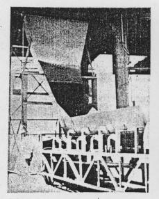
Chute at preparation plant discharges 6x0 clean coal onto conveyorway.
