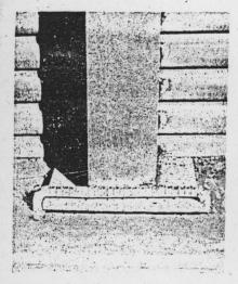
Flanges of arches were slipped under reinforcing bars set in concrete.
