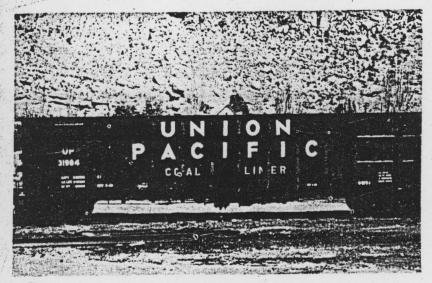
One-hundred 100-ton, specially-designed high-side gondola cars will haul more than 700,000 tons of coal annually in 8,400-ton unit trains.
