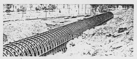
**Tunnel** is 456 ft long with control room in center. Structure is covered with approximately 10 ft of earth material.
