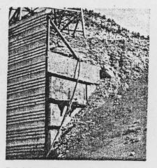
**Retaining walls** at each end of tunnel were constructed with old mine cars filled with earth material.
