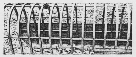
Arches and reject steel mats form tunnel structure.
