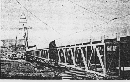
Conveyorway and tower move coal to the 70,000-ton stockpile area. Coal is elevated 120 ft in 1,250 ft, horizontal distance.
