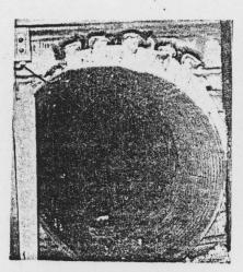
Escapeway and ventilation tube for control room is approximately 228 ft long and 42 in in diameter.
