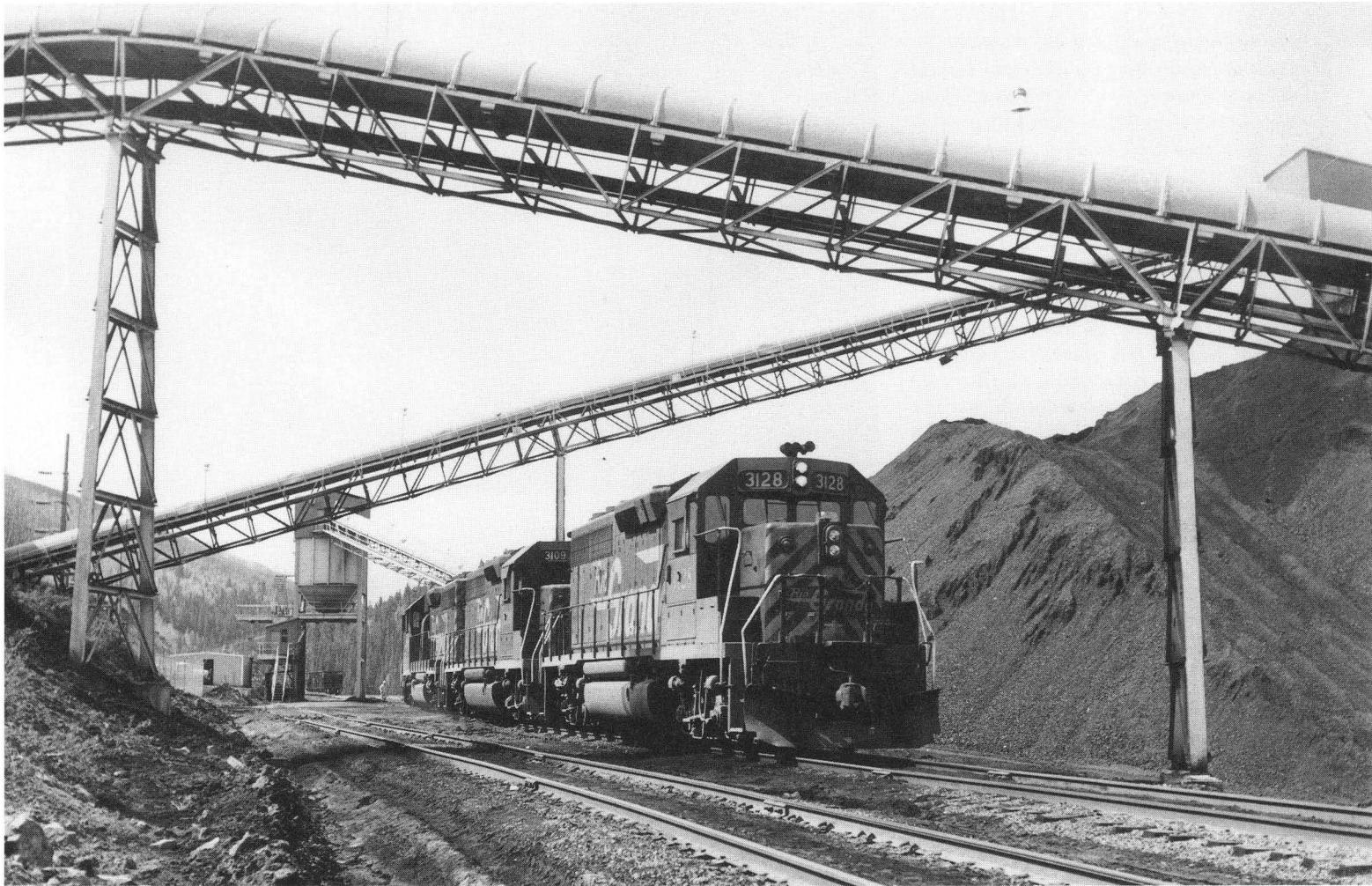
The belt conveyors of the Valley Camp Coal Company form a frame for the three D&RGW units running around their train preparing to load 8400 tons of coal. Long the mainstay of Pleasant Valley, coal is still king there on June 7, 1982. (J.L. Ozment photo)
