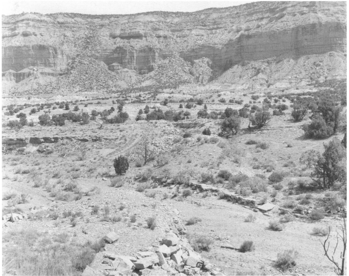
An abandoned narrow gauge grade on which rails were never laid curves from the left foreground across this scene looking downgrade at the base of Cedar Mountain between Green River and Castle Valley (Jackson Thode photo). The carefully laid stone box culvert is still functioning, with no maintenance done in 100 years. It will no doubt still remain a century and more from now as a monument to this railroad building endeavor. (J.L. Ozment photo)
