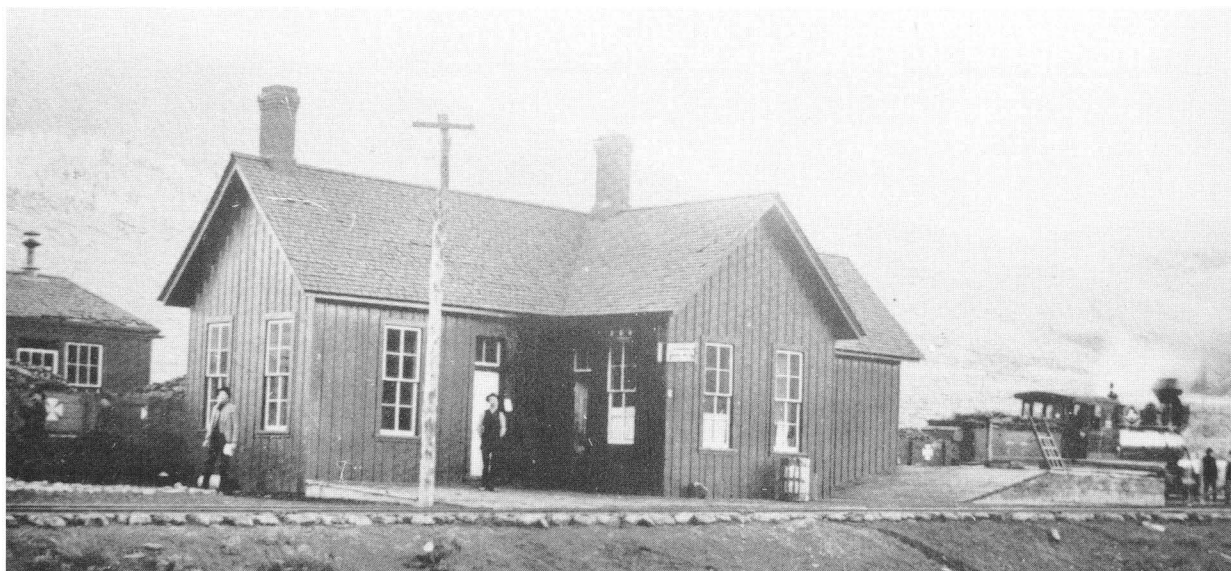
D&RGW Railway locomotive 77 is on the house track at the original Scofield board and batten depot. The maltese crosses on the narrow gauge gondolas indicate that the picture was probably taken in 1889. (Museum collection)
