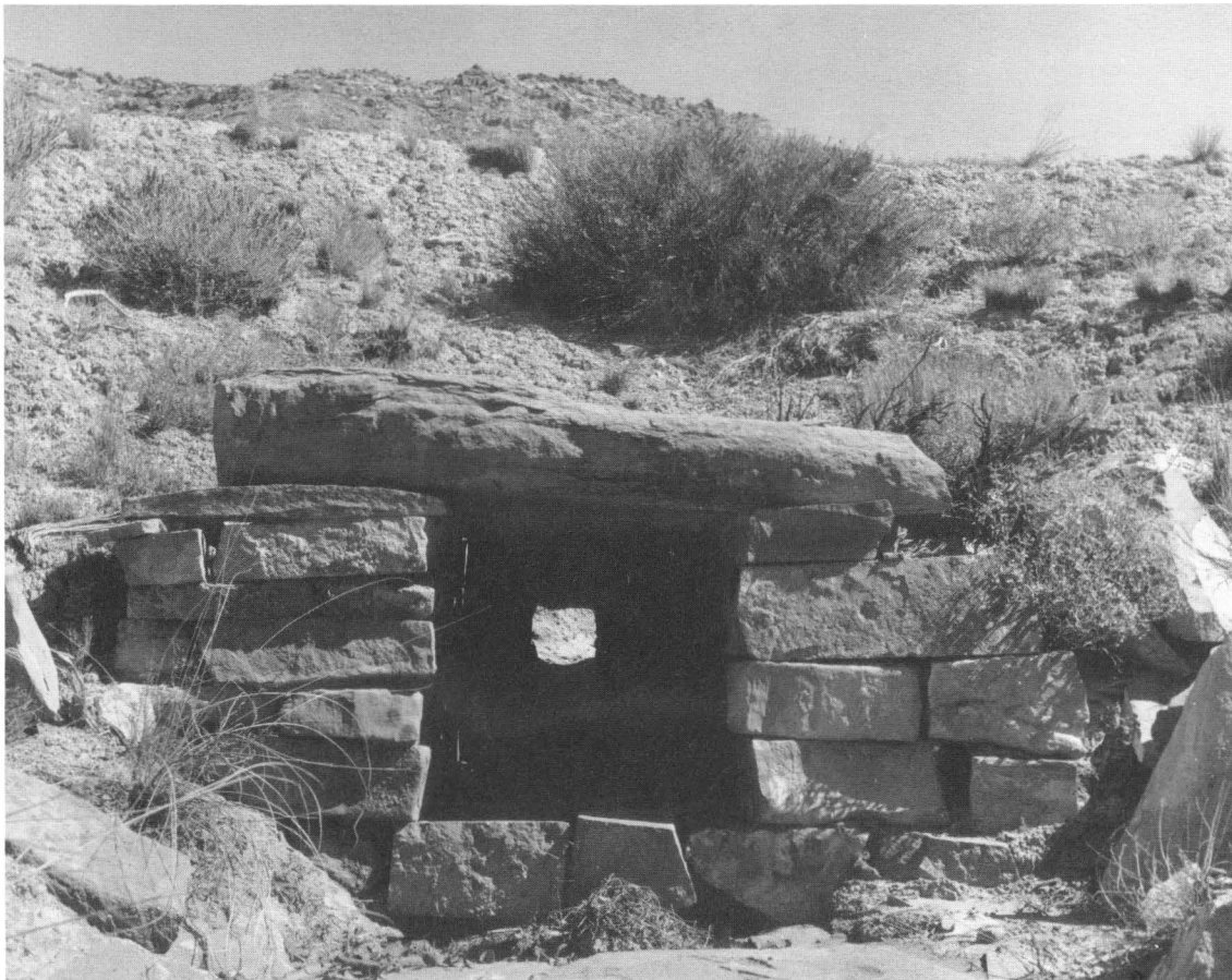
An abandoned narrow gauge grade on which rails were never laid curves from the left foreground across this scene looking downgrade at the base of Cedar Mountain between Green River and Castle Valley (Jackson Thode photo). The carefully laid stone box culvert is still functioning, with no maintenance done in 100 years. It will no doubt still remain a century and more from now as a monument to this railroad building endeavor. (J.L. Ozment photo)
