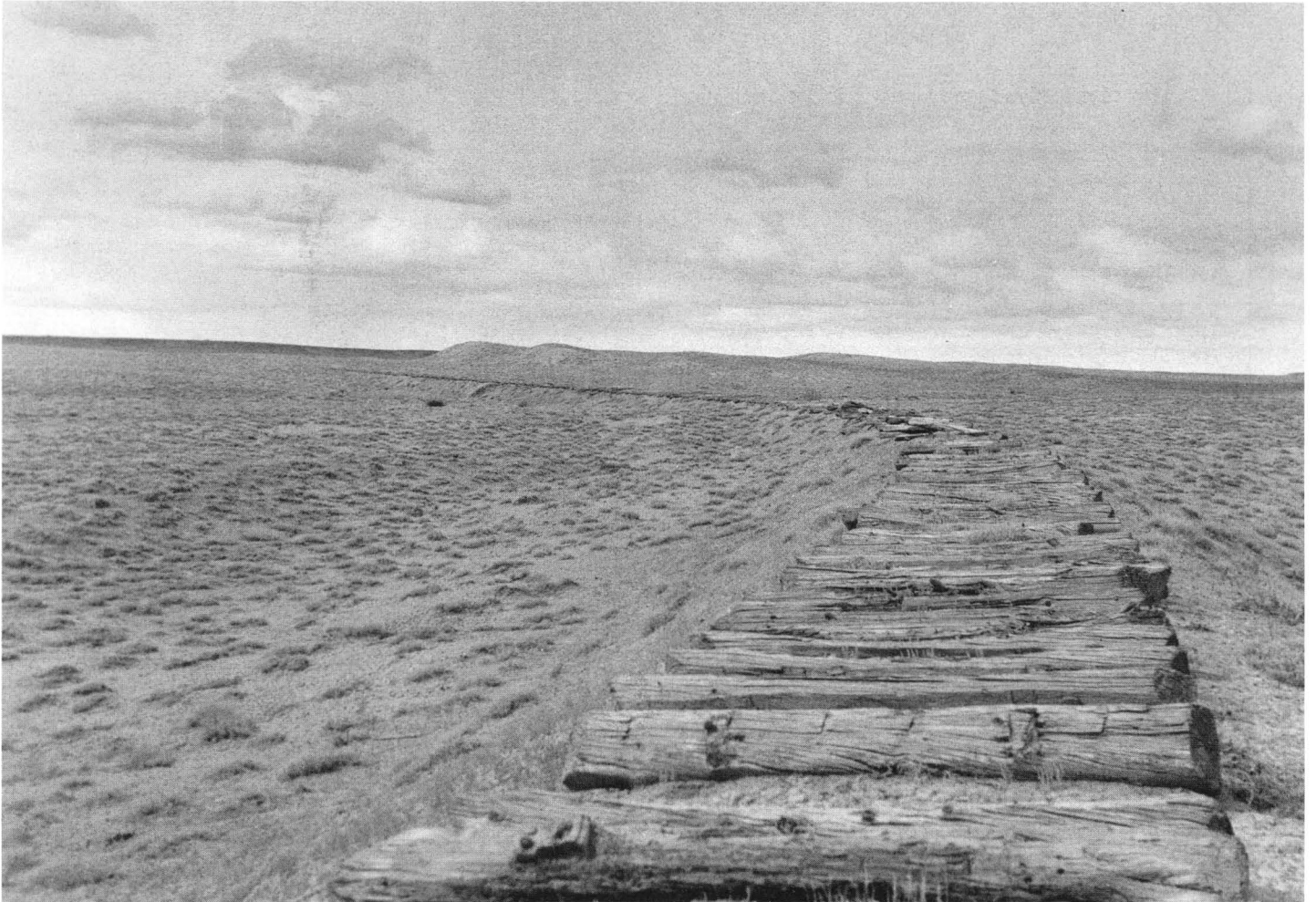
Unseen by travelers speeding along nearby Interstate 70 or on Amtrak's California Zephyr, a long line of hand-hewn narrow gauge pole ties laid down in the winter of 1883, some still with spikes and 30-pound rail braces, marches to the horizon across an eastern Utah desert landscape that still would be recognized by Hodgman and his colleagues from that long-ago surveying party (Robert W. Richardson photo)
