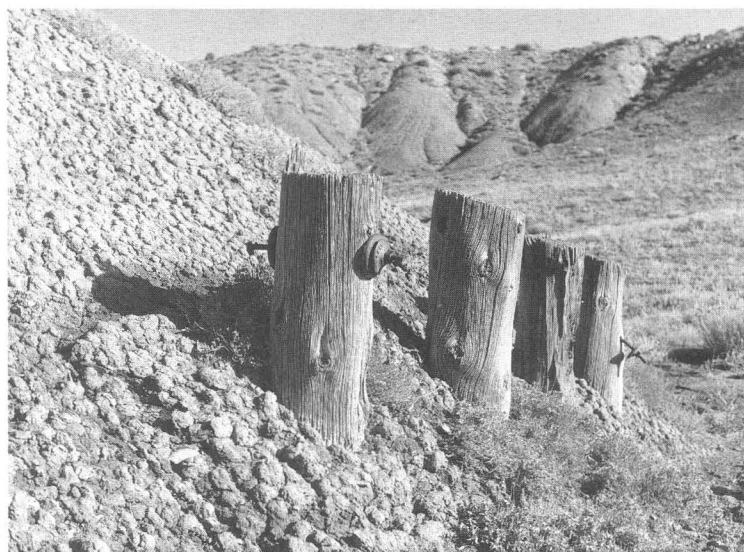
Evidence of the desert grade alignment can be found here and there, if one takes the time to look. A set of saved-off bents from an abandoned trestle near Floy slowly decomposes into the dry desert "popcorn" soil.
