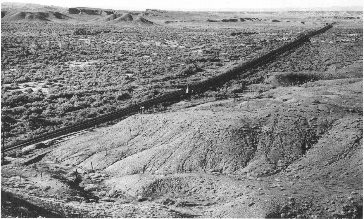
The late afternoon sun of October 2, 1978 highlights the present standard gauge alignment west of Woodside. Near the signal case at center, the original narrow gauge veered left, barely seen in the photograph, and followed the Price River upstream to a junction of Grassy Trail Creek, thence up to near the old siding of Verde. The present alignment was constructed in 1890 to eliminate the severe flooding problems along the original route. (J.L. Ozment photo) The poem is from an 1895 Rio Grande Western promotional booklet titled Utah. (Museum collection)
