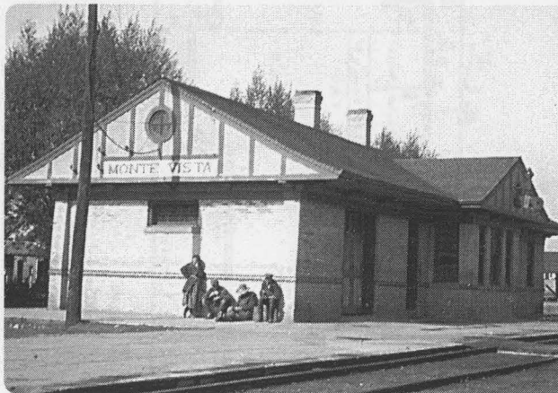
Second Depot-Front View.
