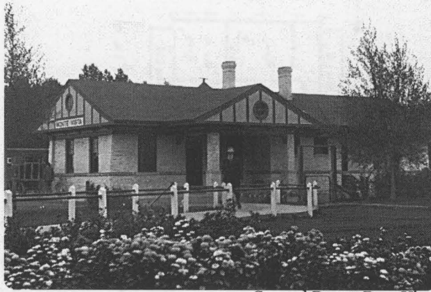
Second Depot-Rear View.
