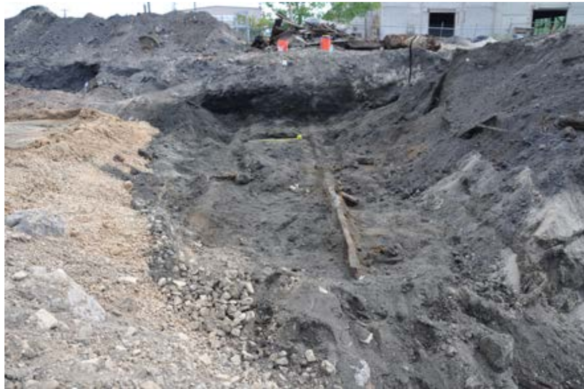
Figure 15. In situ metal rails and wood ties with chains attached, measuring tape at 3 feet.
