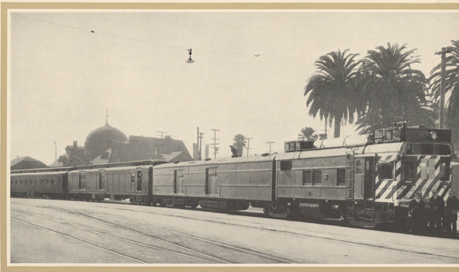
The Sante Fe 900 Horsepower Locomotive unit, articulated with a baggage car. This was one of the forerunners of the "Streamlined Trains" of the modern era.
