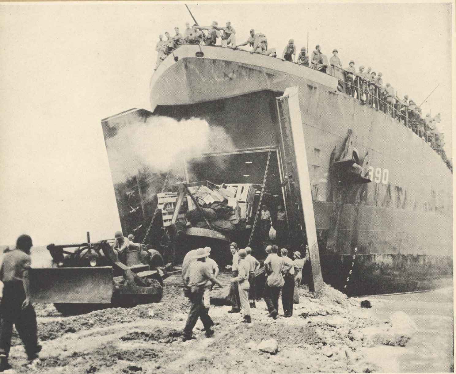
The Mighty Bulldozer comes out of the nose of an LST.
