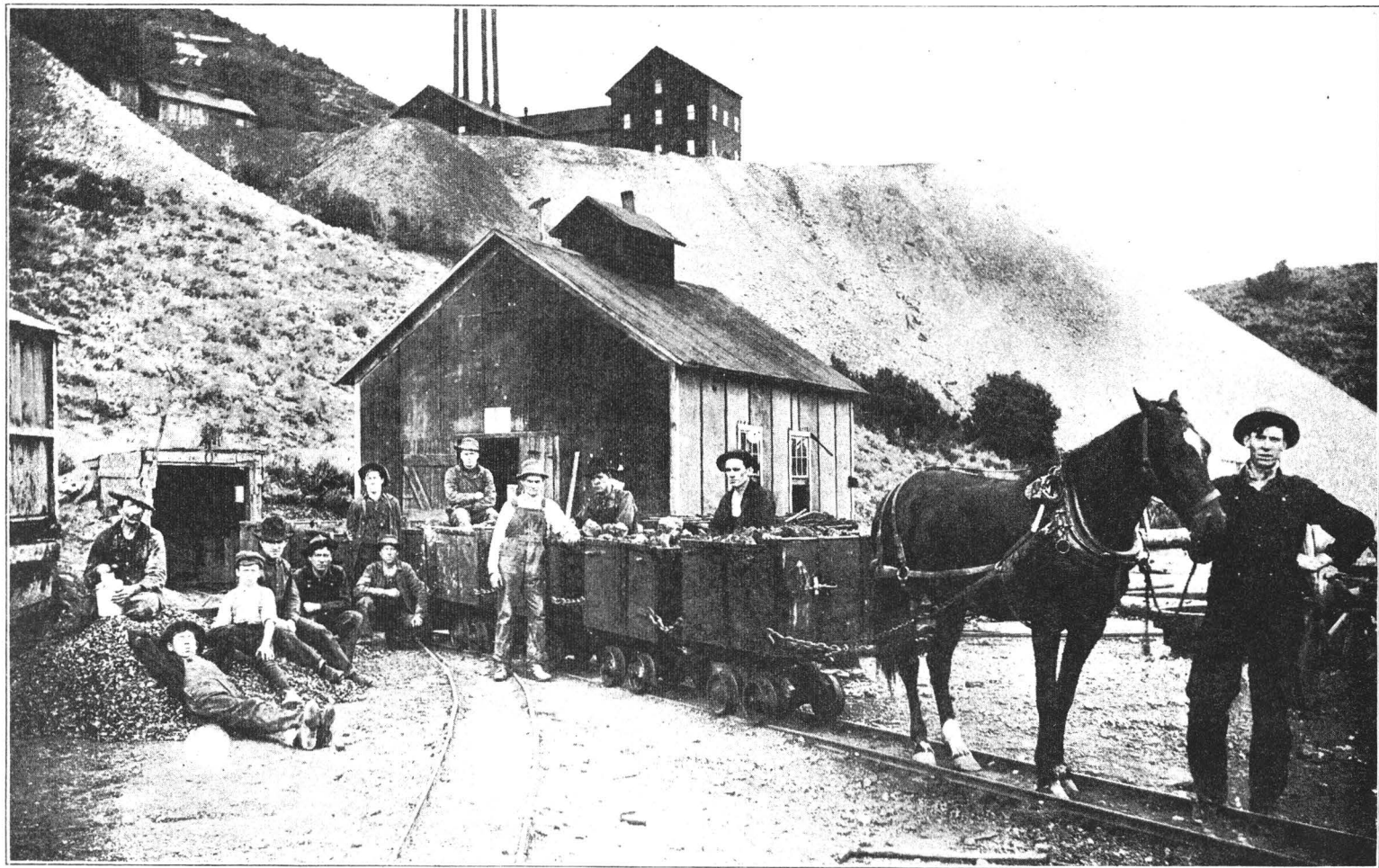
No. 3. Showing "Mule," Horse Train, delivering ore from the Mine to the Mill at the May Day Mining & Milling Company, at Main Entrance of Mine. Owing to the steep grades found in the mine, a horse has proved more successful than a mule.
