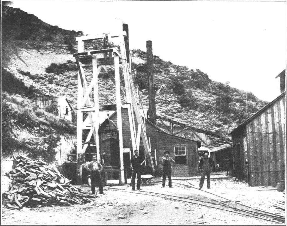
Sioux Consolidated Hoisting Works.
