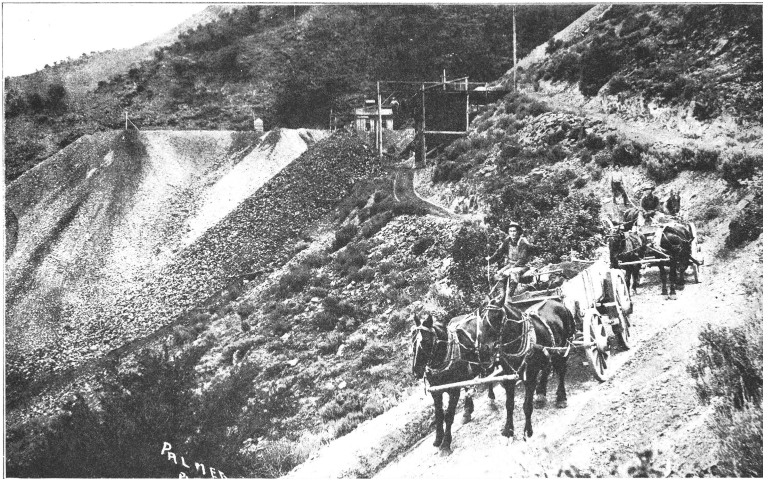
No. 4. Ore transportation at the Humbug Mine of the Uncle Sam Cons. Mining Co. In this manner over one million dollars in ore has been hauled down the mountain side, down a road so steep that the teamsters depend for safety entirely on the brake of the wagon. Should the brake give loose, it would almost certainly mean the killing of the team, possible injury to the teamster, and complete demolishing of the wagon and outfit, besides loss of ore. Very heavy wagons are used, handling over four tons to the load, and particular attention is given to keeping the wagons in good repair.
