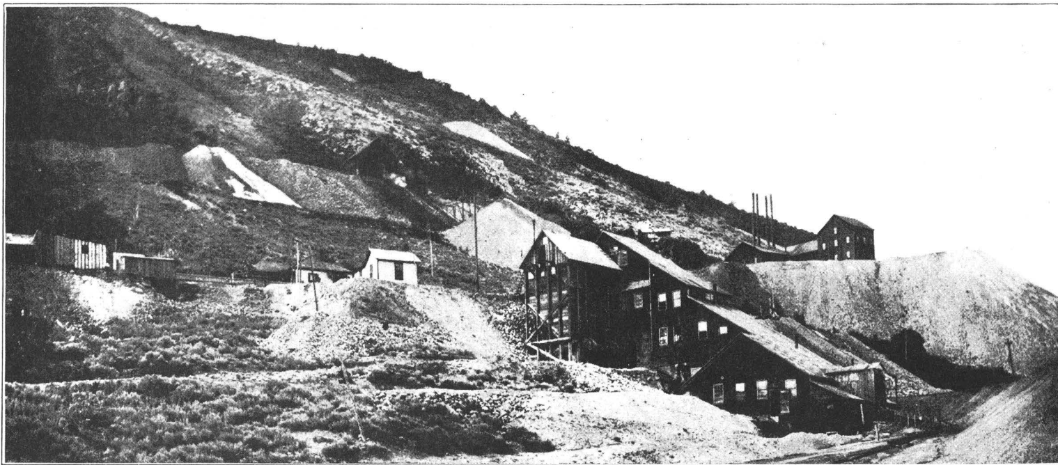
No. 1 May Day Mining & Milling Co., showing hoist, superintendent's residence, office and mill. This mill has been running on low grade ores from the mine for six years. The only successful concentrating mill in the district that has run for anything like this length of time. Treats the low grade ores made in extracting shipping ores from the mine that would otherwise be placed on the waste dump. As a by-product addition to the mine is very successful.
