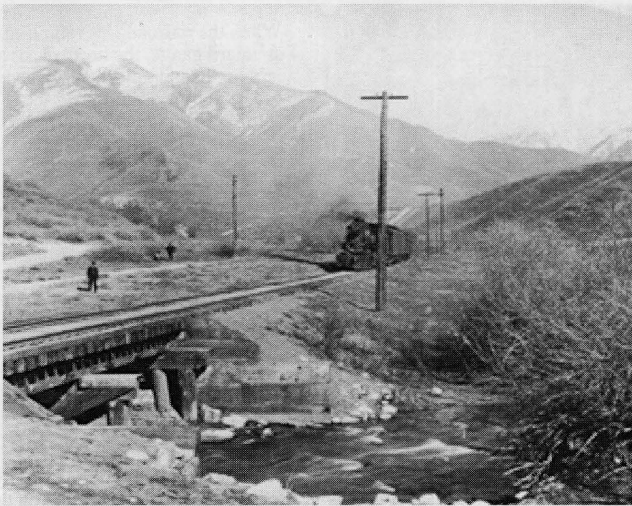
Bridge and road crossing at 27th East. One piling of the bridge still stands. Photo taken from 27th East looking east. Trees around Dudler's Inn can just be seen in the distance beyond the men standing on the other side of the tracks.
