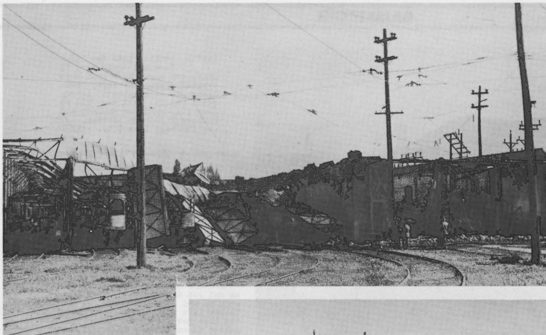
General view of the destroyed car house, substation, and cars. Note to the right center the horn gaps of the lightning arrestors which exploded through the window directly beneath them. Had the window been bricked up, the entire loss would have been only a few hundred dollars. All of the destroyed buildings were constructed of steel frames, brick walls, sheet metal fronts and wooden roofs.
