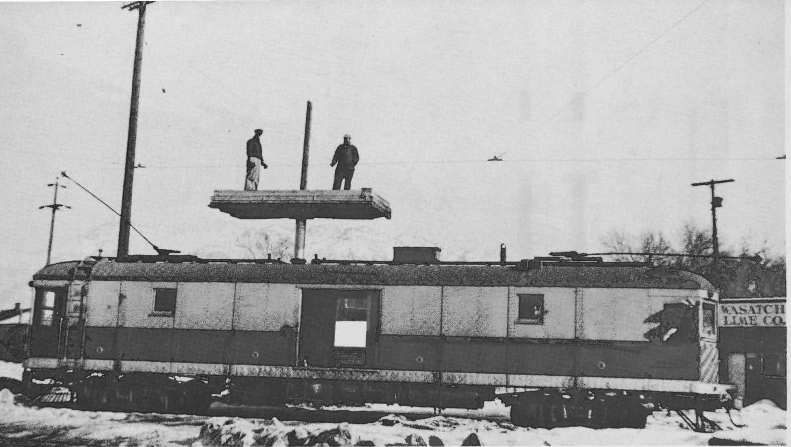
Two camera studies of Bamberger Railroad's line car 05. In upper photo, the unusually deluxe tower car is seen working in Ogden on January 30, 1949. In photo below, the car is in the hole awaiting a regular train's passing so it can resume its task of keeping the overhead wire in excellent condition. (Both, FF)
