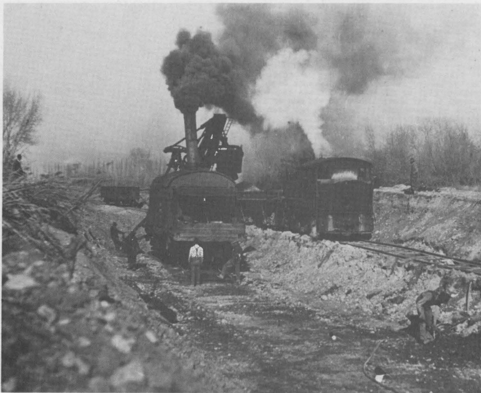
Heavy construction was necessary to carry the OL&I's interurban line north to Preston. In the above photo, a steam shovel is seen hard at work in the "big mud cut" just over the Idaho border. (FF)
