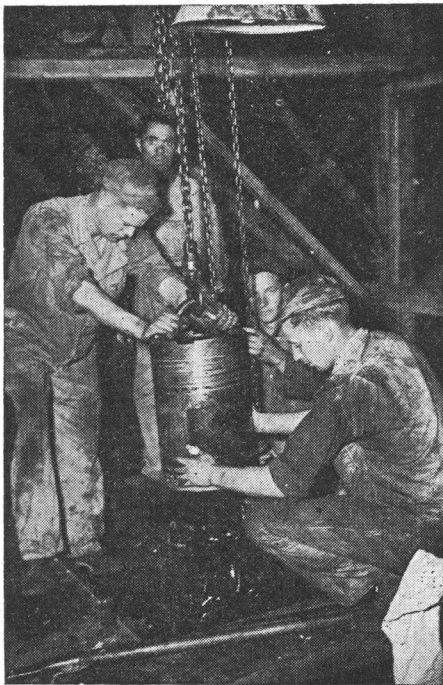
Dropping a Piston Into a Cylinder of an American-Built 1,000-hp. Diesel-Electric Locomotive
