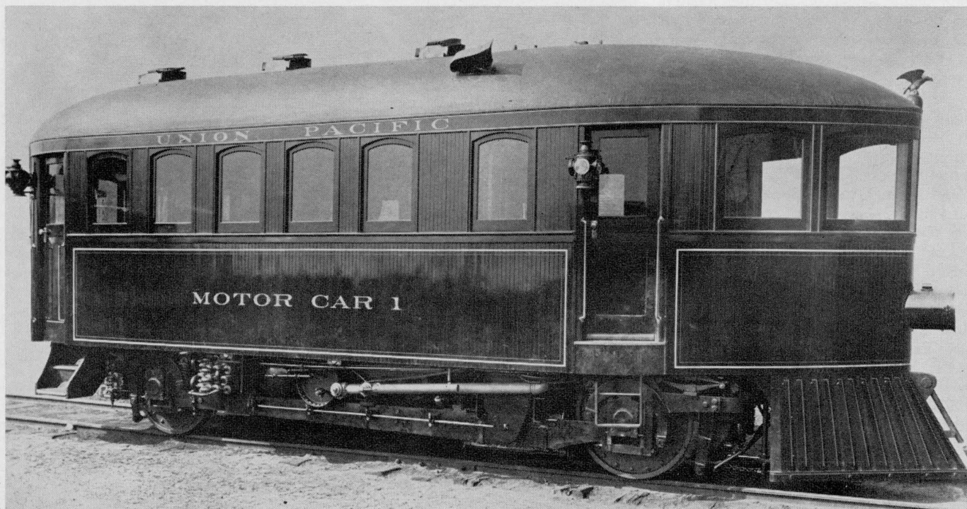
ORIGINAL McKeen car of 1905 featured what developed to be wrong-way streamlining, and an automatic streetcar-type rear door.
