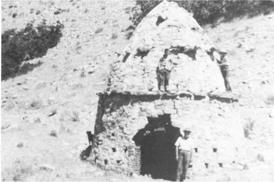
This charcoal kiln was in Soldier Canyon in 1962. The kiln has evenly spaced openings to control the air in making a high carbon fuel from pine logs. Charcoal was used in smelter furnaces in the Stockton area. Other kilns were located in Vernon, Pine Canyon, Tooele City, and Settlement Canyon. When coal became available the use of kilns was discontinued.
