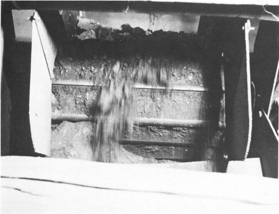
Pan Feeder/Conveyor from Hopper to Jaw Crusher
