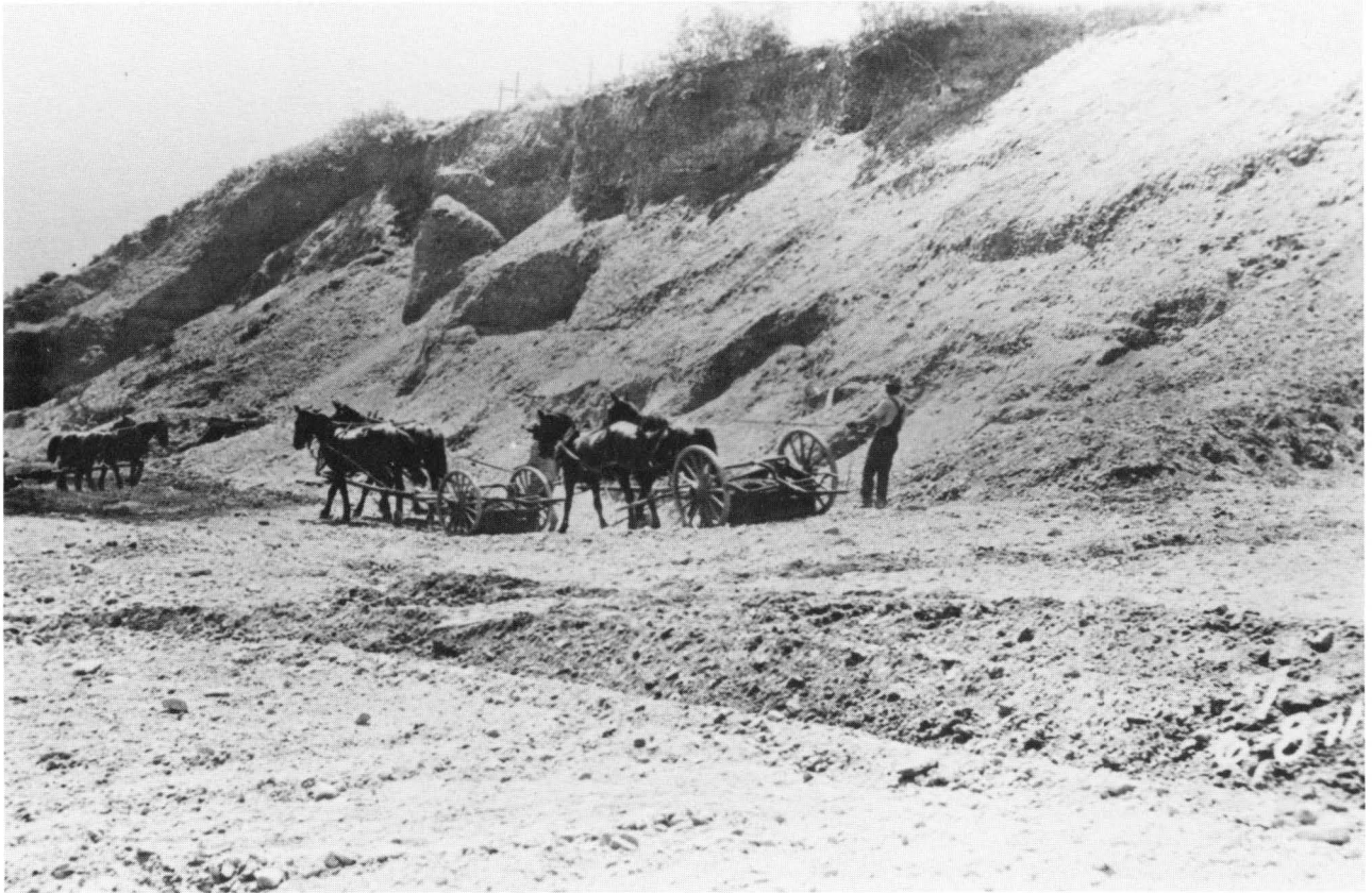
Initial construction stage Tooele Smelter.
