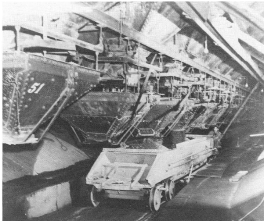
Scale Room — Blast Furnace Charge Floor. Sinter, other ores, fluxes and coke are proportioned by weight and hauled to the blast furnace.
