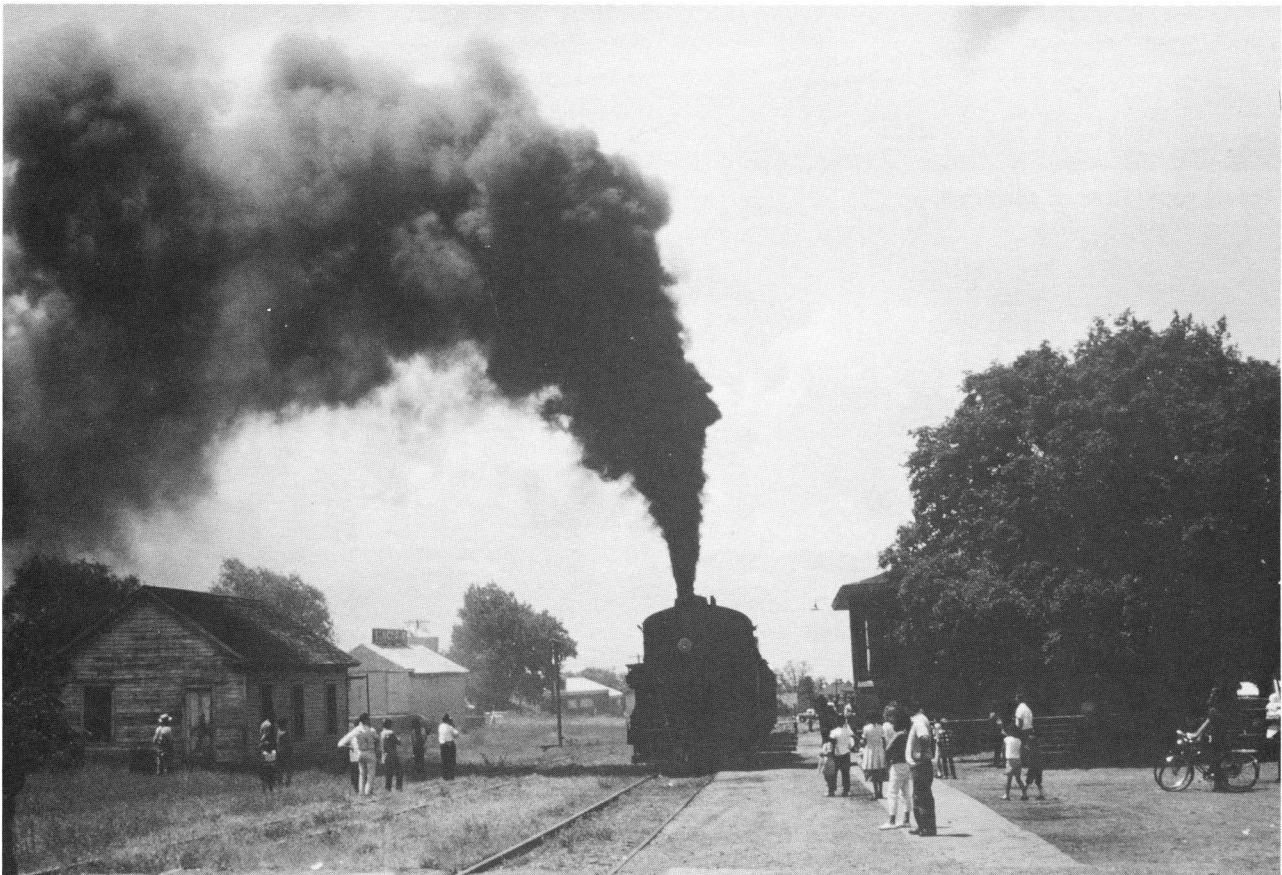
Last run of the steam locomotive pulling freight cars 30 May, 1963. Depot building behind trees at right.
