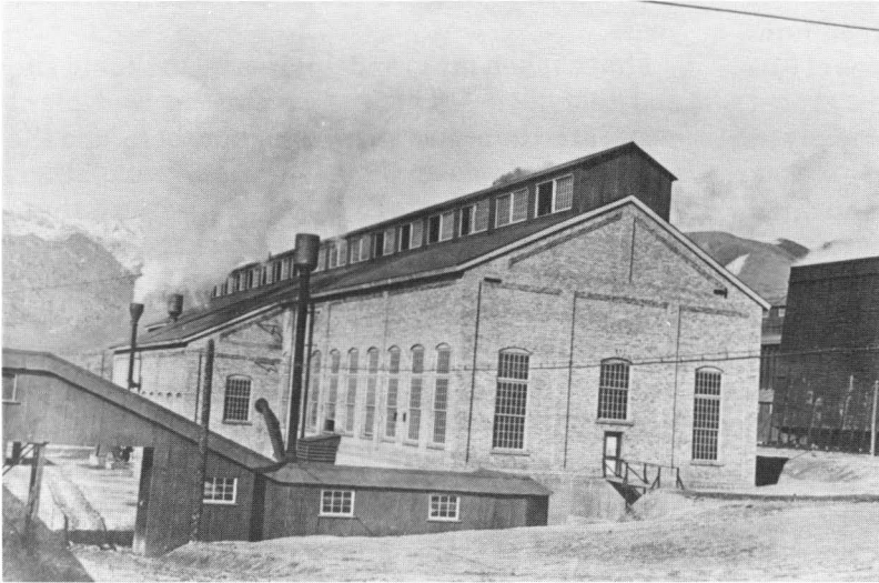
Tooele Smelter powerhouse produced AC and DC electricity and compressed air.
