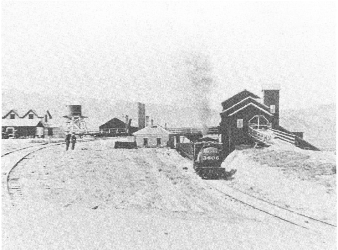
Gravity Mill Ore Concentrater built by Bullion Coalition Co. 1910. Later redesigned for flotation process of sulphide ores in 1927.
