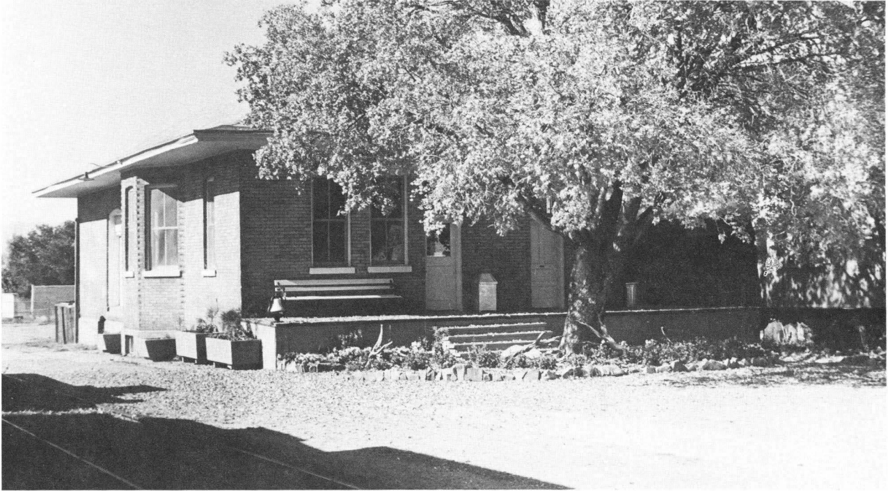
Tooele Valley Railroad Depot and operations office. As of 1983 a museum and registered as a historical site.
