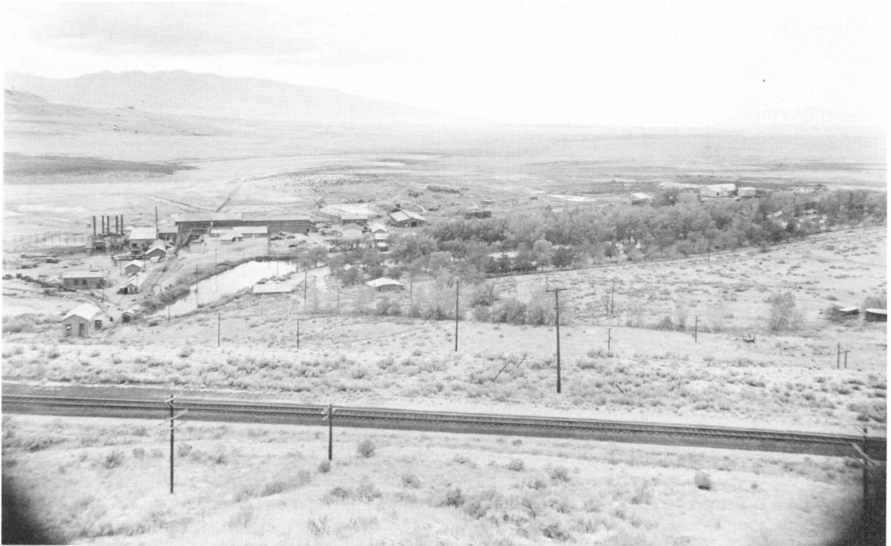
Bauer 1954 (approx) mine portal and change room left center, Mill upper left. Resin Plant near dikes and black coal piles. Remains of orchard upper far right. Dwellings center and right. Union Pacific Railroad Trailer foreground.
