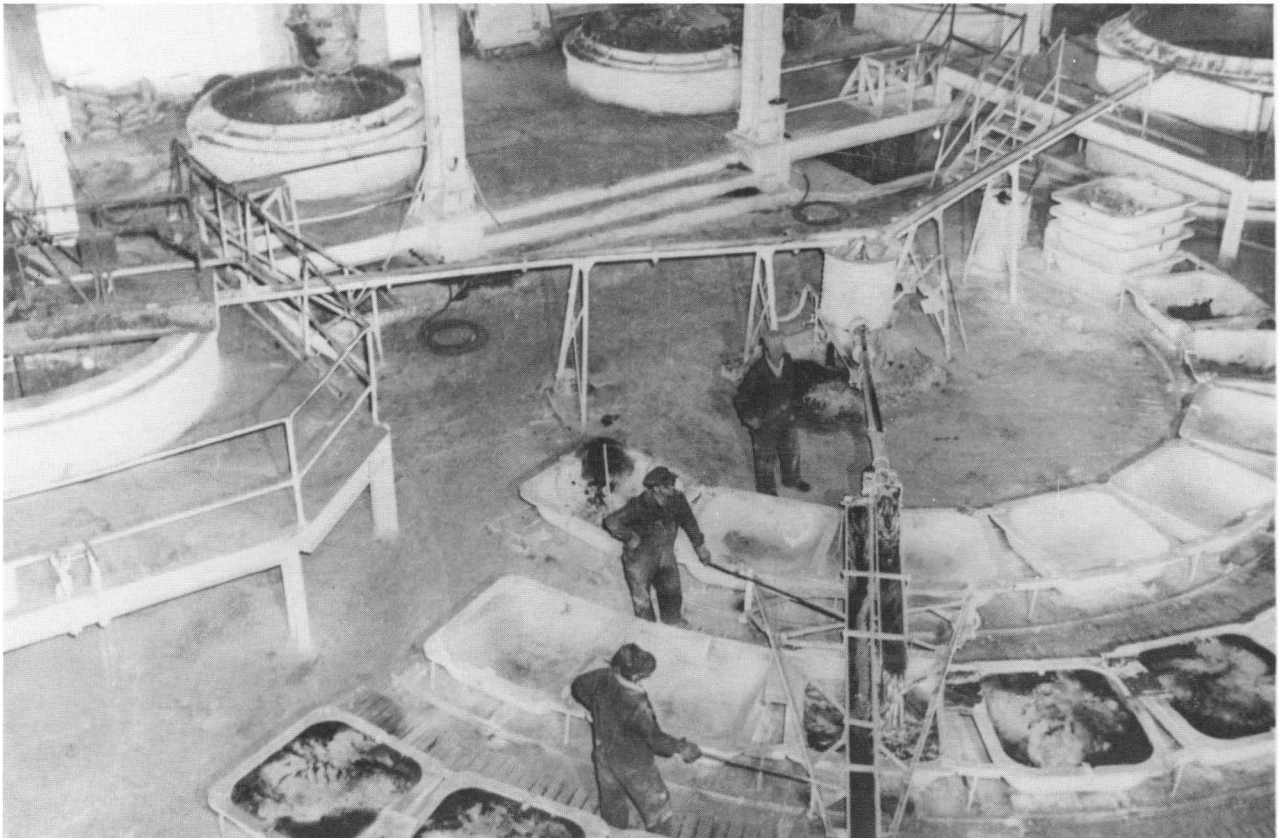
Blast Furnace Dressing plant, lead ingots weight 4 tons each.
