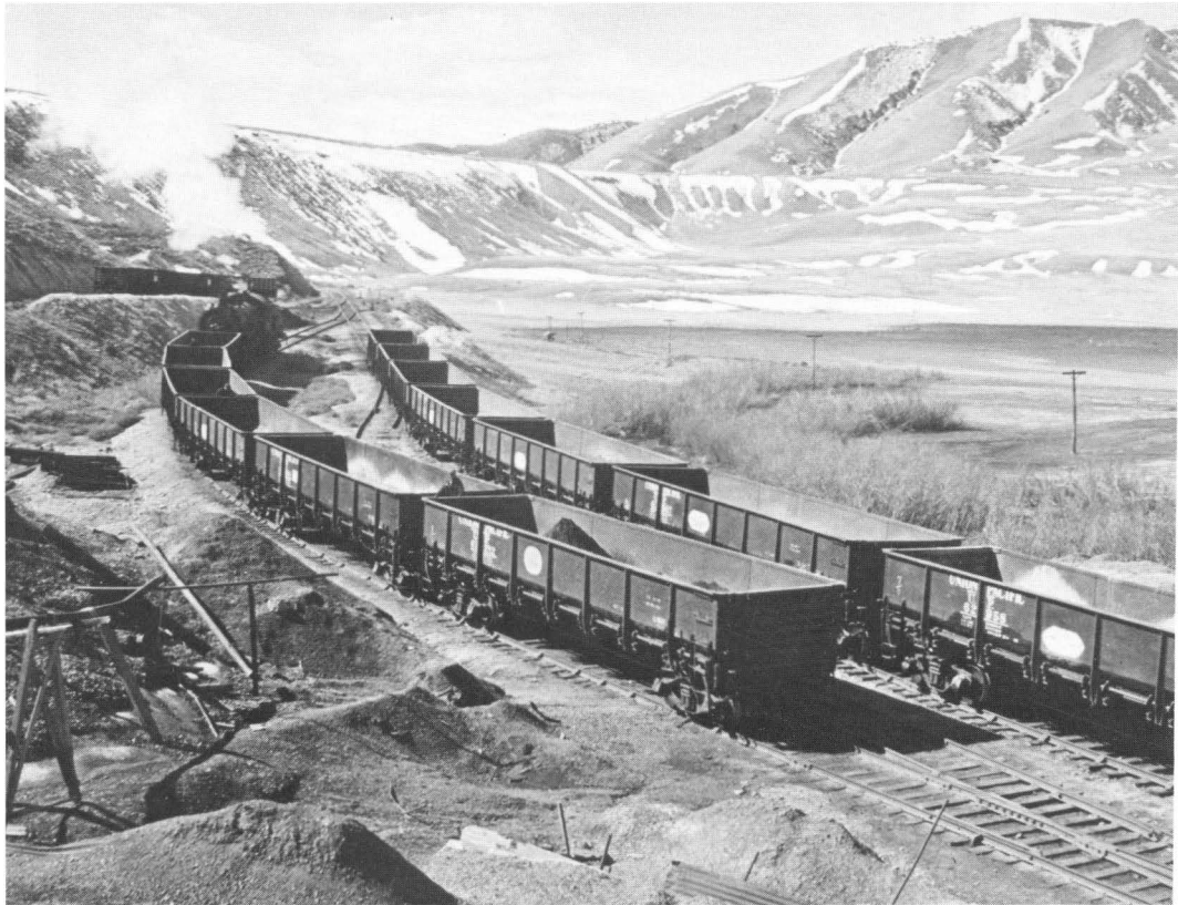
Rail Switching Yard
