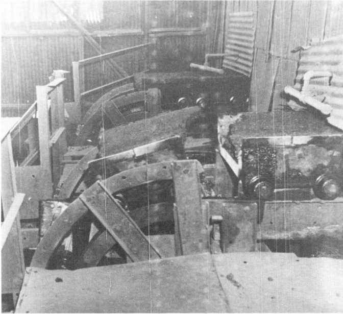
Discharge end of D&L Sintering Machine. Most of the sulphur has been burned out and the ore is agglomerated. The sinter is sent to the lead blast furnace.
