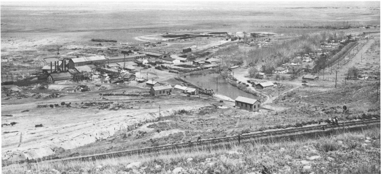
Bauer Plant Operations Circa 1954. Looking NW mine portal East of change room and pond. Large building is mill. East of mill maintenance shops, NE of mill laboratories, assay office and storage building, Panacalite plant and resin plant top right. Boarding house and scale house center. Dwellings right center.
