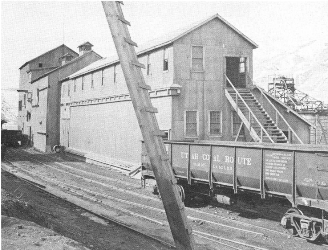
Mill Ore Bin Building
