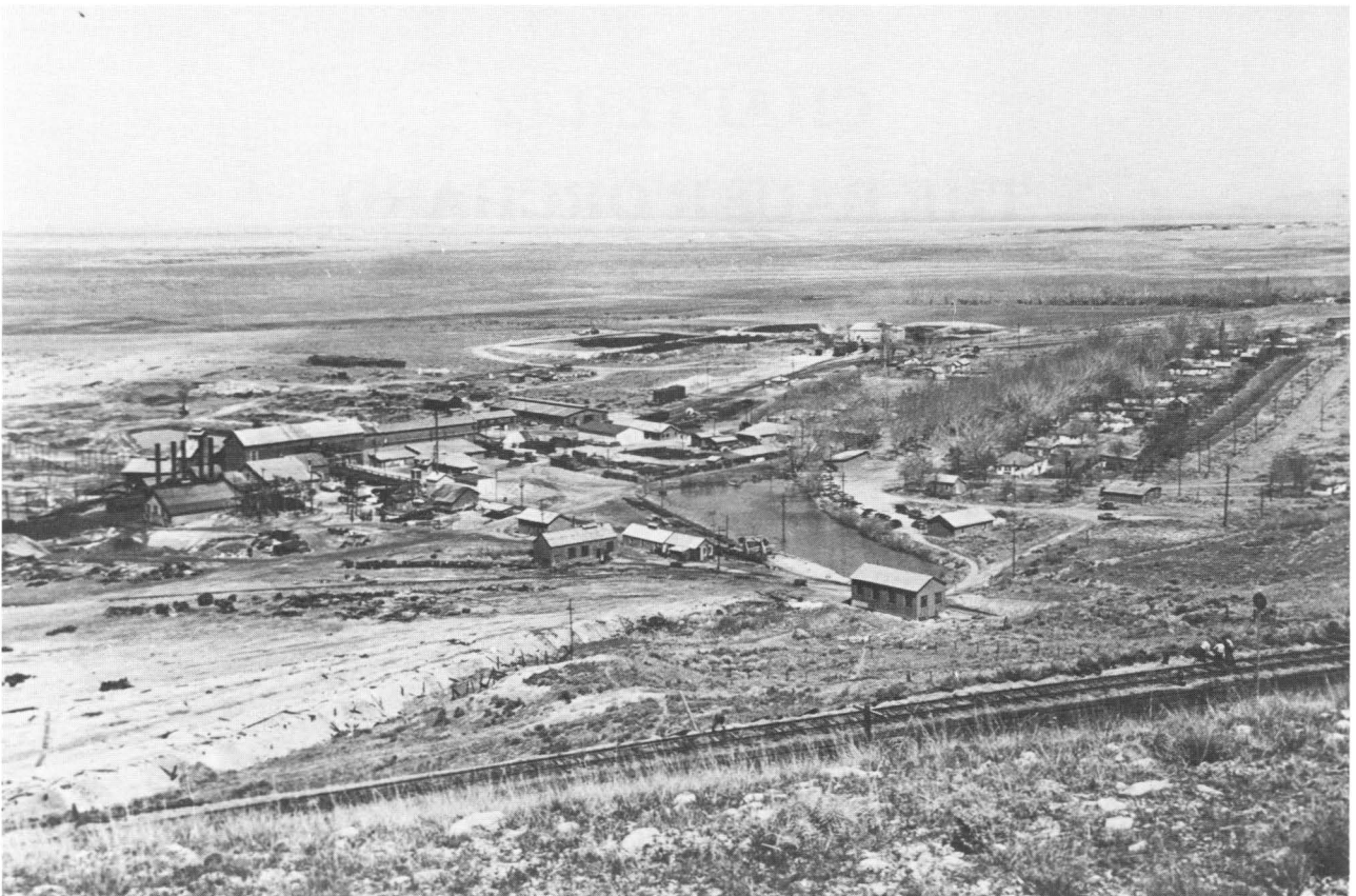
Bauer Plant foreground. Union Pacific Railroad, mine portal and change rooms.
