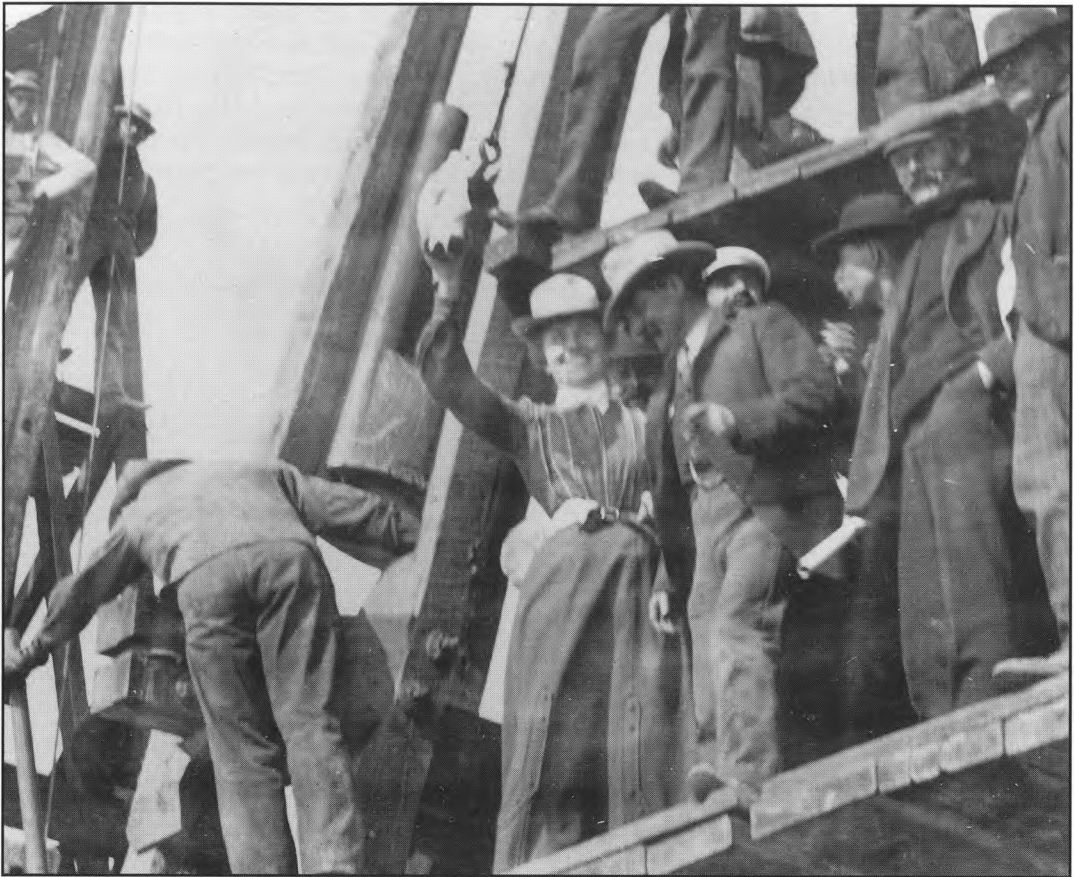
Mrs. Ogden holds up the bottle of champagne that she will place atop the last pile, so that when the 3,200 pound hammer delivers the last blow, the bottle will be crushed. Standing beside her is William E. Marsh, engineer in charge of construction.
