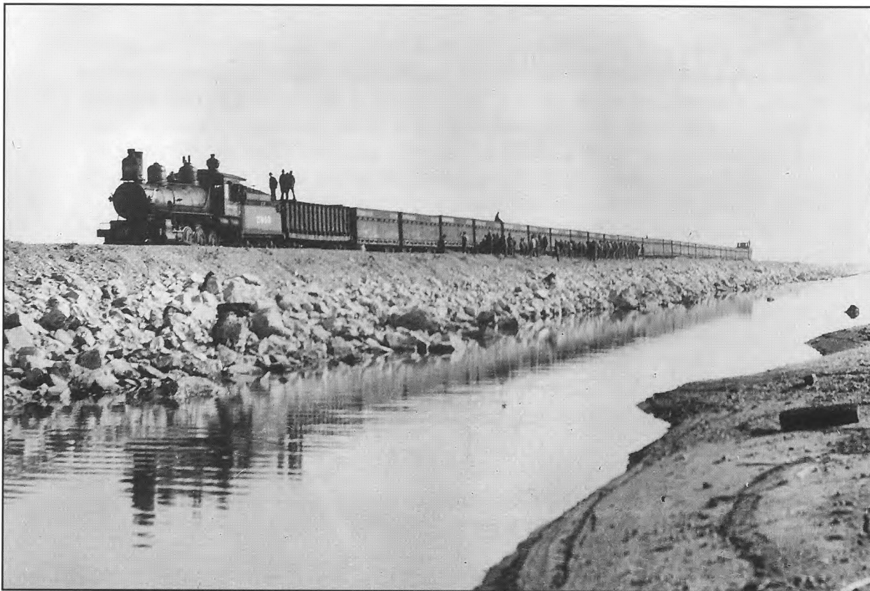
Here the track has been raised. The only sign of the sinking grade is the uplifts from which the photographer took the picture. To the right of the dump cars are some of the 3000 workers employed on the Lucin Cutoff. California State Railroad Museum, Collection:387-253 No.16981
