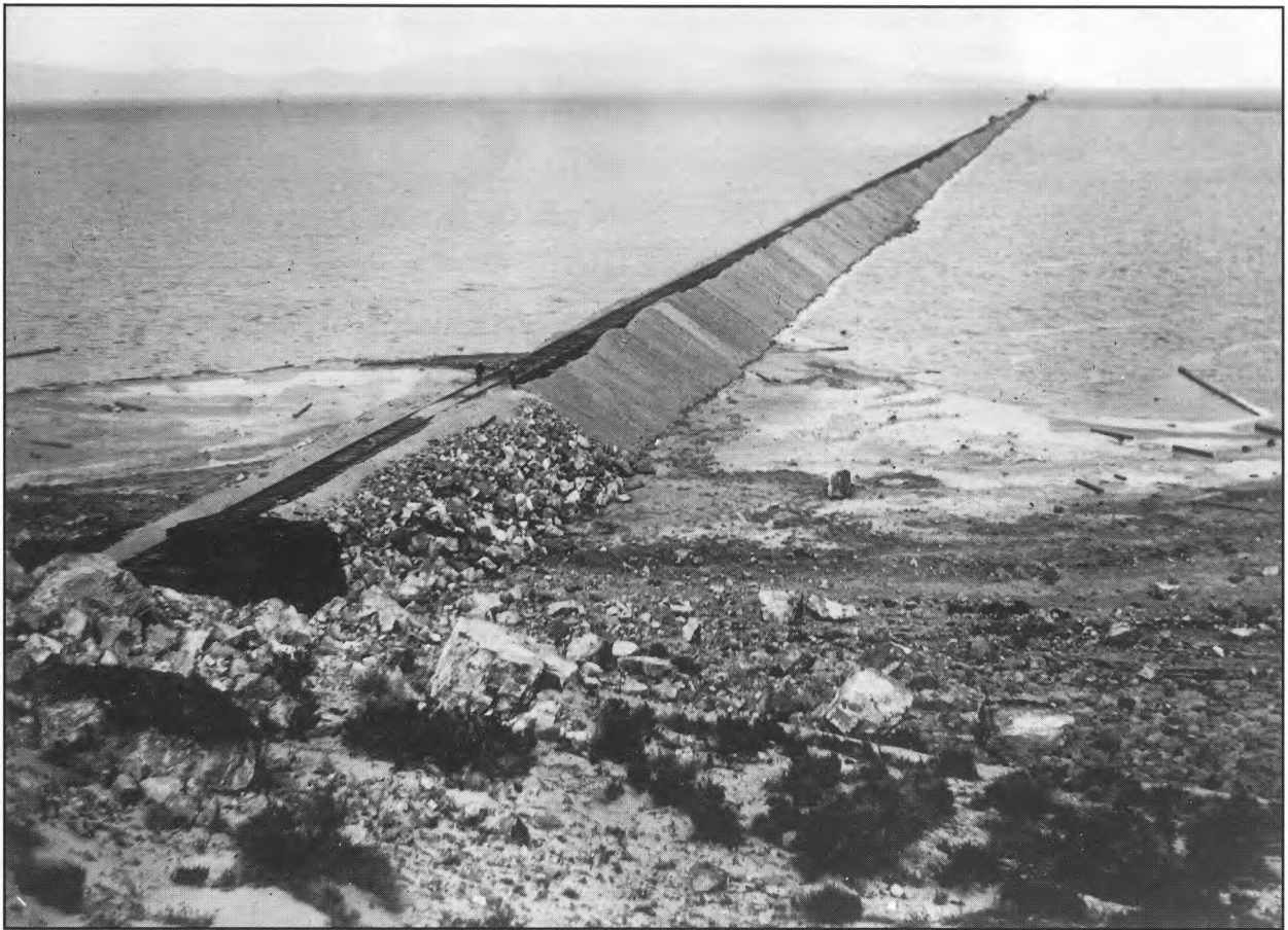
Temporary trestle after being filled in. Looking east from Lakeside toward Promontory. California State Railroad Museum, Collection:387-253 No.16982
