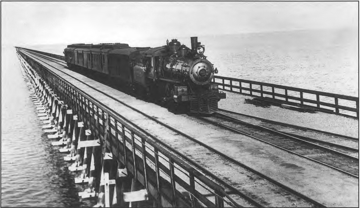
The newly completed trestle was single tracked, but had a siding at Midlake for trains to pass each other. Used by permission, Utah State Historical Society, all rights reserved Photo no. 763
