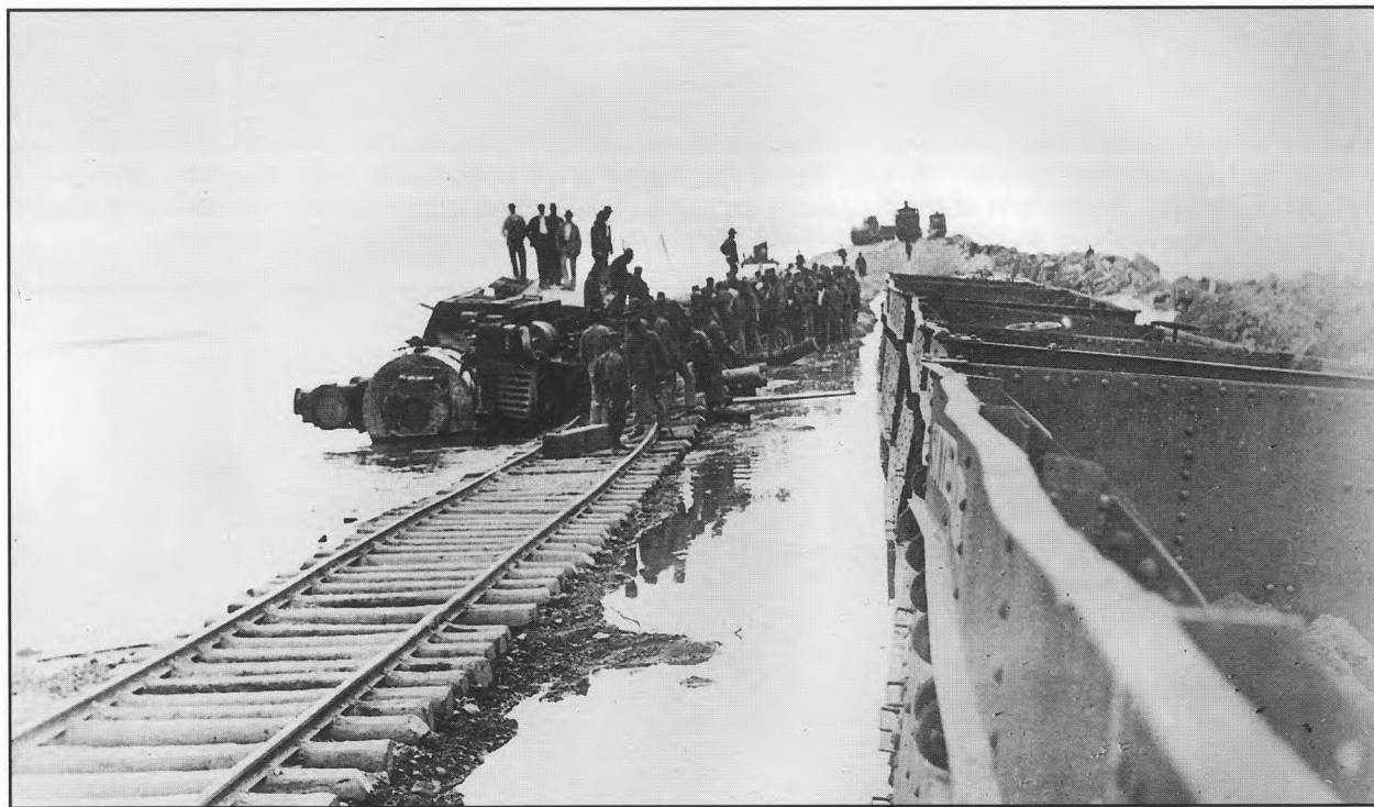
The famous pilot engine for the Harriman Special lies mired on its side at Rambo sink. In the background can be seen the height of the grade before it failed. The actual sinking of this particular section took approximately twelve minutes. Some of the uplifts were so extreme at Rambo that they stretched out 300 feet on either side of the fill.
