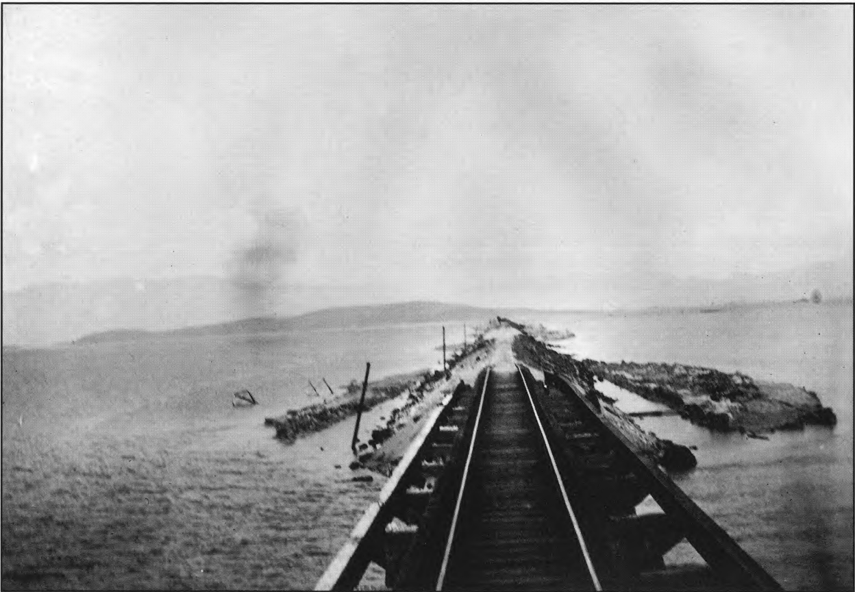
From atop the trestle, a view of the mess faced by Southern Pacific's engineers. Note the uplifts on both sides of the track. So extreme were some that the piling inside the embankment was forced out and to the surface more than 100 feet from the tracks.
