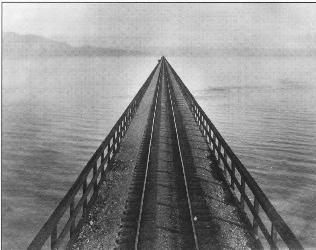
Three inches of asphalt roofing was laid down over the trestle's heavy decking, and then ballasted with fourteen inches of gravel and rock.
