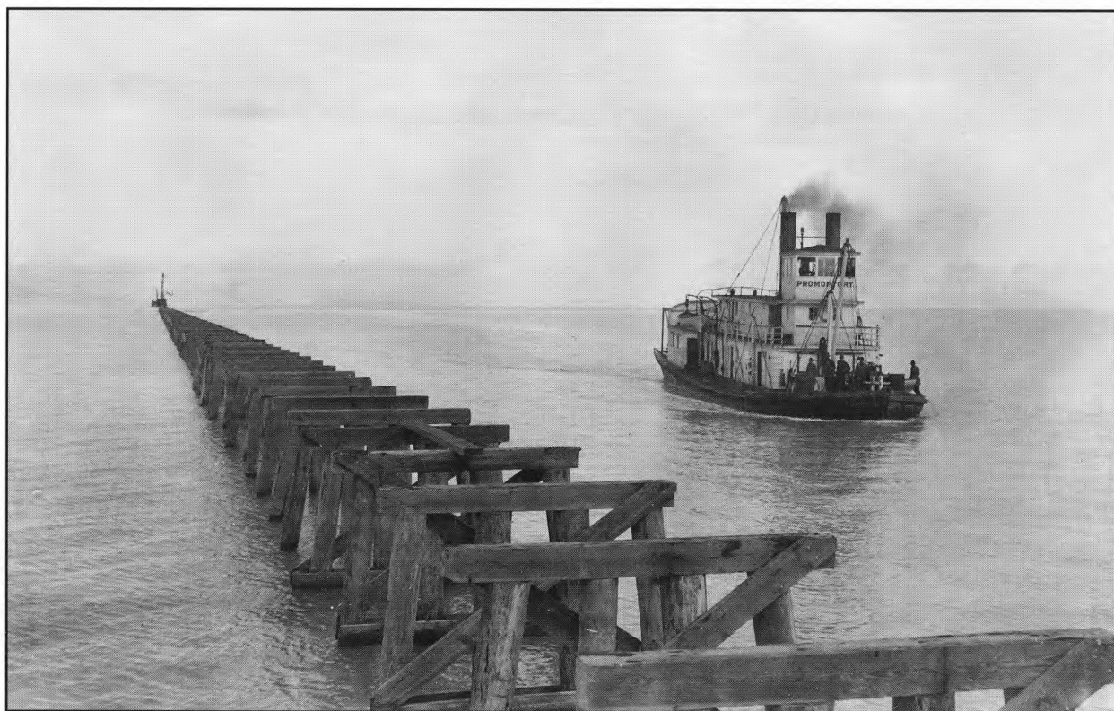
Four piling per bent, each bent 15 feet apart, was the specification of the temporary trestle. The steamer, Promontory is on the right.
