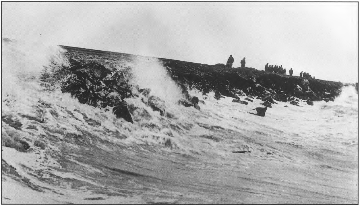
Huge waves batter the side of the Lucin Cutoff embankment. Note the large rocks used to keep smaller material from washing away.
