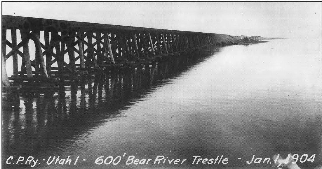
C.P.Ry. - Utah I - 600' Bear River Trestle - Jan. 1, 1904 The only opening between the eastern shore and Promontory was this 600' section of permanent trestle, called the Bear River trestle, which still exists today.
