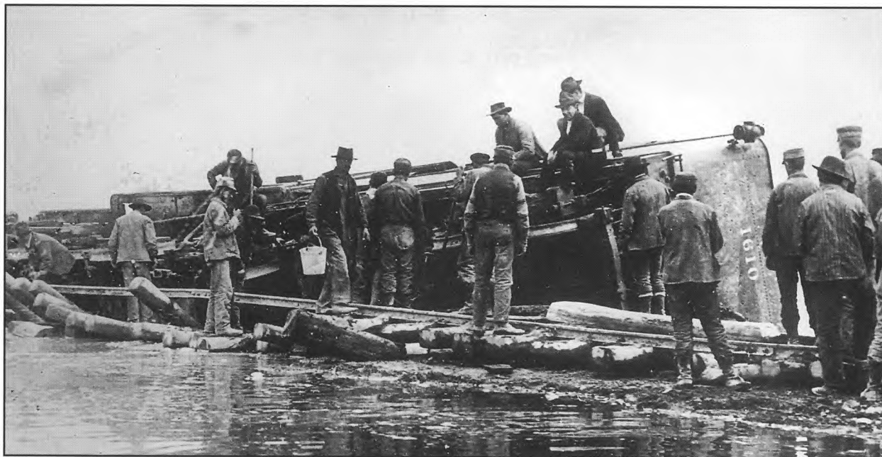
Workers mill about near an overturned locomotive at Rambo sink, yet another failure of the grade. Used by permission, Utah State Historical Society, all rights reserved Photo no. C-525 #38
