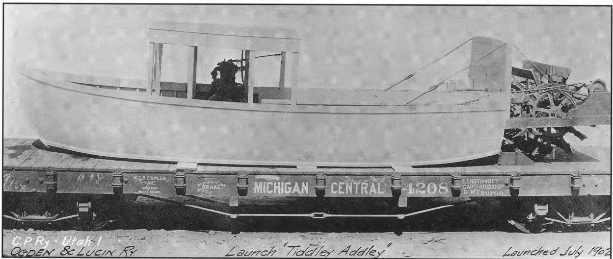
Southern Pacific's Pioneer vessel on the Great Salt Lake, the 30-foot gas-powered paddle wheel Tiddley Addley . Although beneficial to the railroad to facilitate a roadway in the extreme shallows of the lake, the Tiddley Addley was said to be "more of a whining, grinding failure than a howling success".
