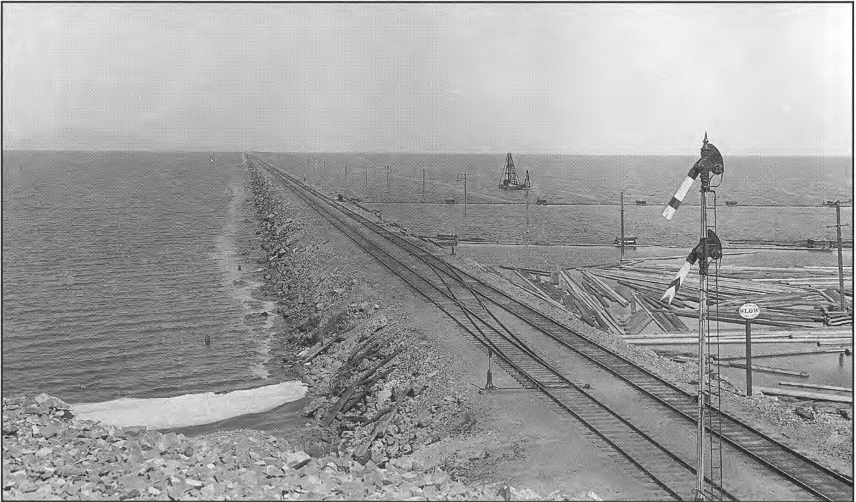
The finished roadway (looking east From Lakeside towards Promontory). The piling booms were kept on the south side of the fill to protect them from the harsh northerly winds.
