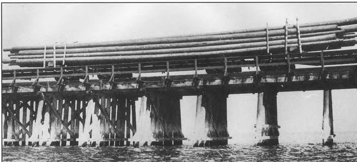
The 40 foot flat cars give scale to some of the pilings used in the deep water section of the Lucin cutoff. 38,000 piles were used in the construction of the Lucin cutoff, some of which were over 120 feet long. The cost of the Oregon pine logs was $60 each, a tidy sum considering a laborer on the project was paid $2 a day. Used by permission, Utah State Historical Society, all rights reserved Photo no. 558
