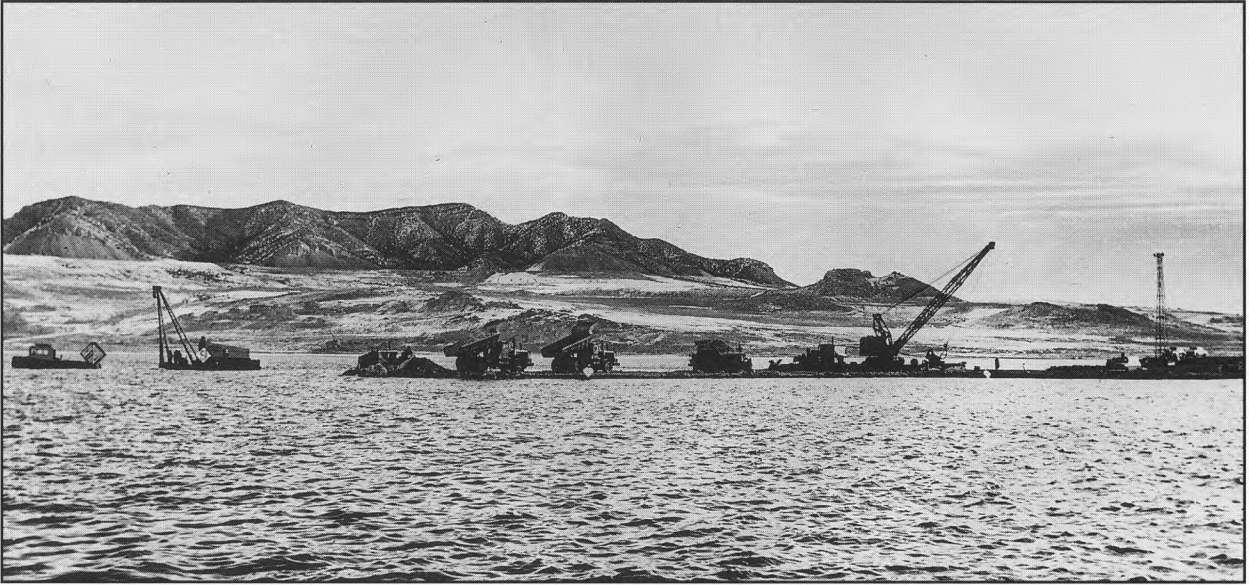
A variable army of workers and equipment worked from both ends while the barges and tugs raised the bottom of the lake between. In the background are the snow-flocked mountains of Promontory Peninsula. Used by permission, Utah State Historical Society, all rights reserved Photo no. 769
