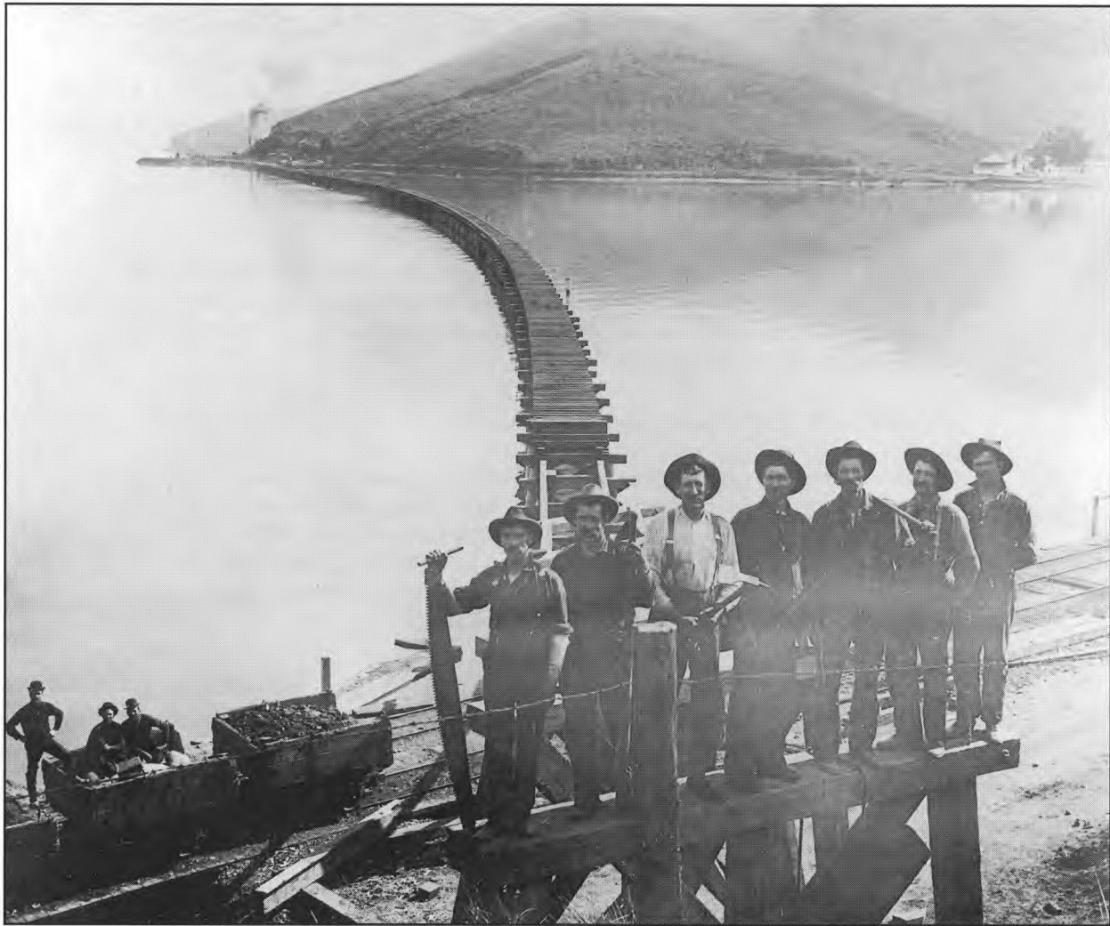
Western Pacific finally gave Salt Lake City its direct route to the coast when it built around the south end of the lake not long after the Lucin Cutoff was completed. Workers stand atop the temporary trestle that cuts across a section of the lake.
