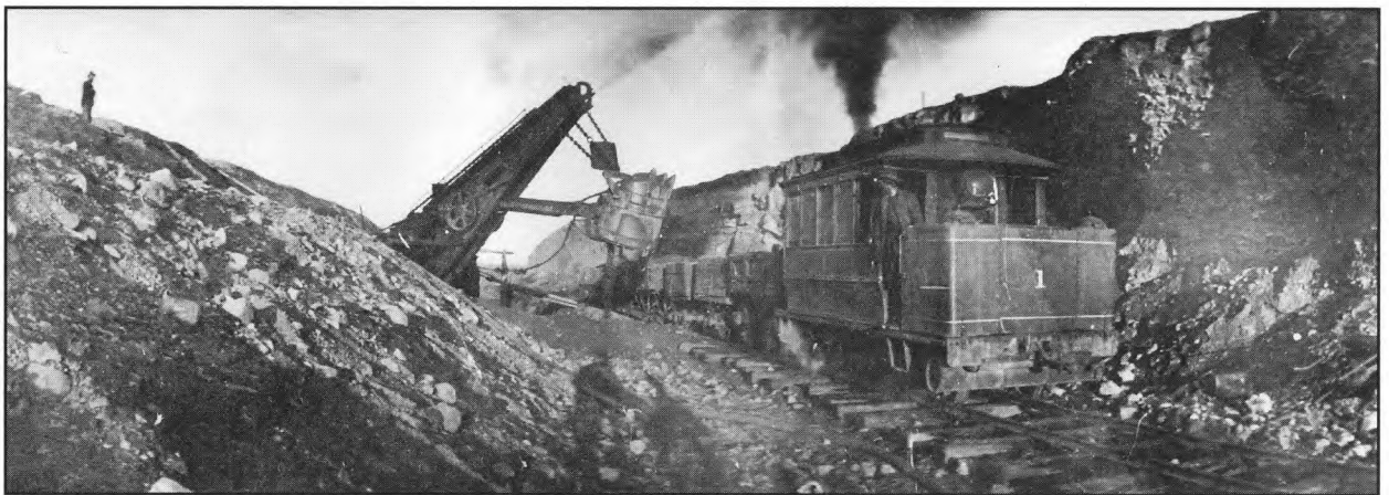
Excavating rock from Lakeside quarry on the west side of the lake. Steam shovels were provided by the Bucyrus Company at a cost of $10,000 each. California State Railroad Museum, Collection:387-253 No.16973
