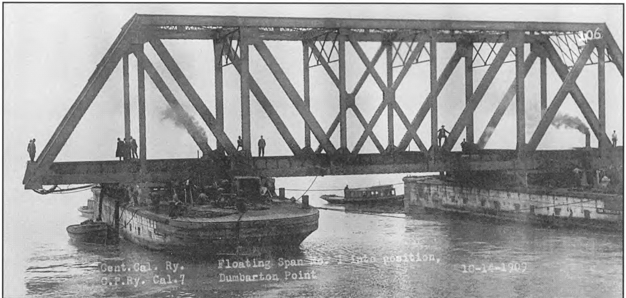
Two huge sailing ship hulls converted into barges serve as a means to transport the spans of the Dumbarton Draw Bridge. Near the center of the photo is the Risdon No. 3 . To the left is the Tiddley Addley , which was built or named to replace the Tiddley Addley which was probably left on the Great Salt Lake.
