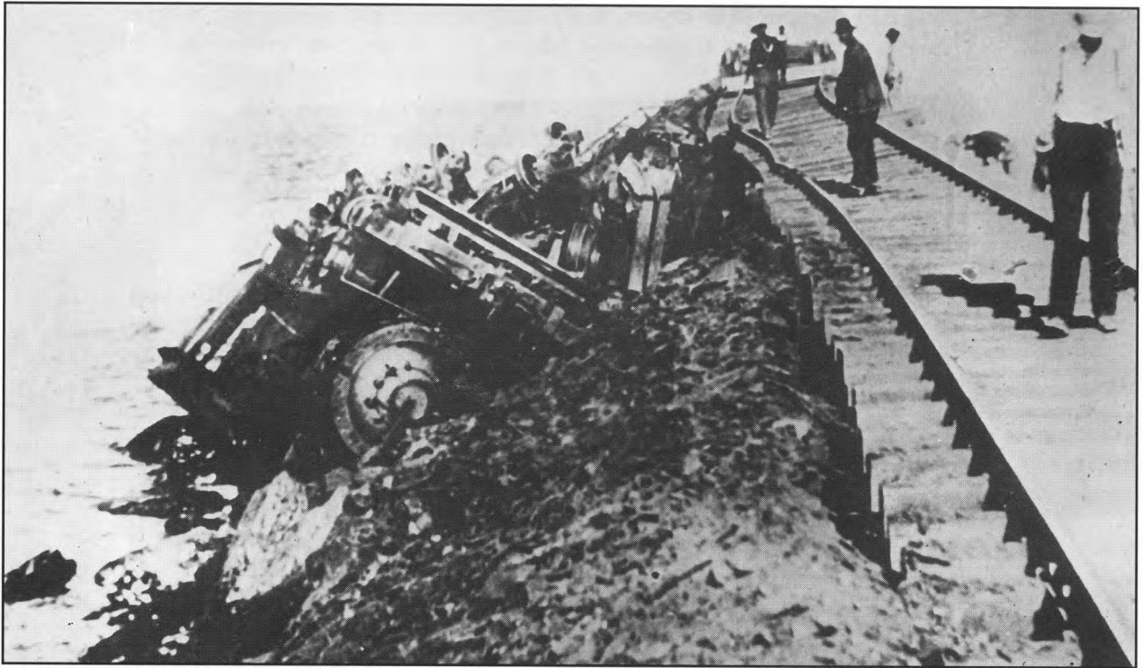
First work-related death, that of Robert W. Watson, occurred west of Promontory, near the approach of the permanent trestle, when engineer Jenken's east bound light engine derailed due to a section of grade settling during the night.
