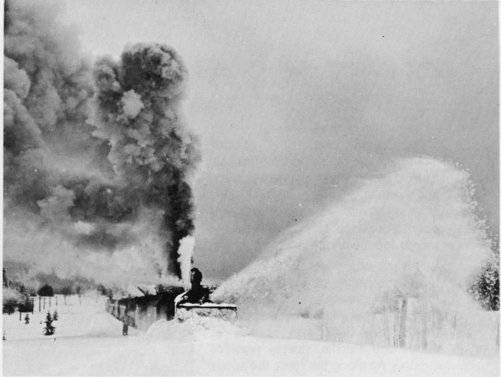
In later years a more modern, but nonetheless steam powered, rotary plow is seen at work. Few pieces of railroad maintenance equipment can match one of these machines when it comes to drama and spectacular action.
