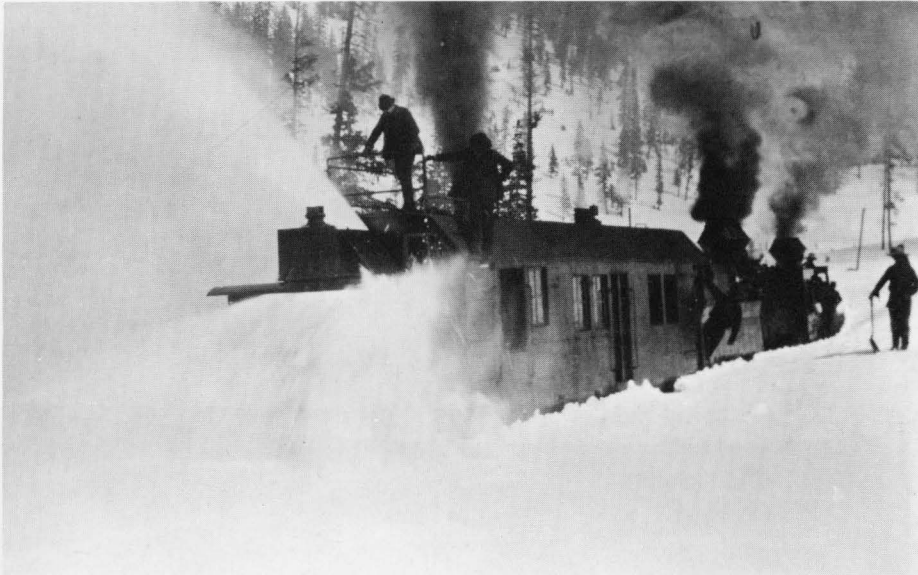
There had to be a better way of removing packed, drifted snow, and the Leslie brothers found it. In this shot from the UP archives
