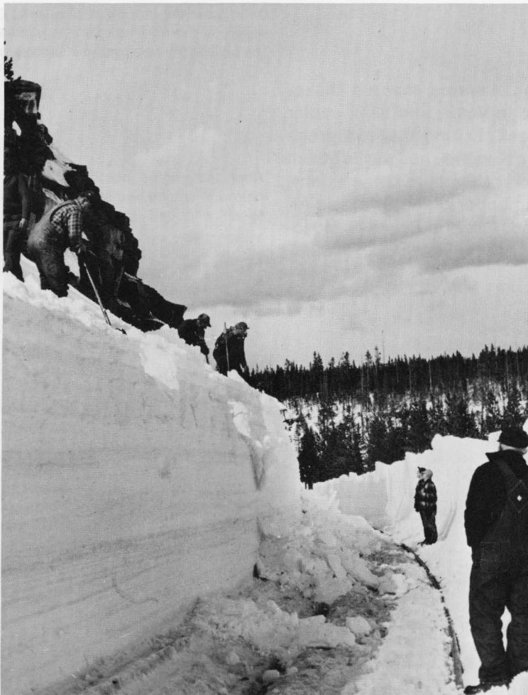
The rotary has been by, but strong arm work still needs to be done. Though the big plows move a lot of snow, they still can't replace good men armed with shovels.
