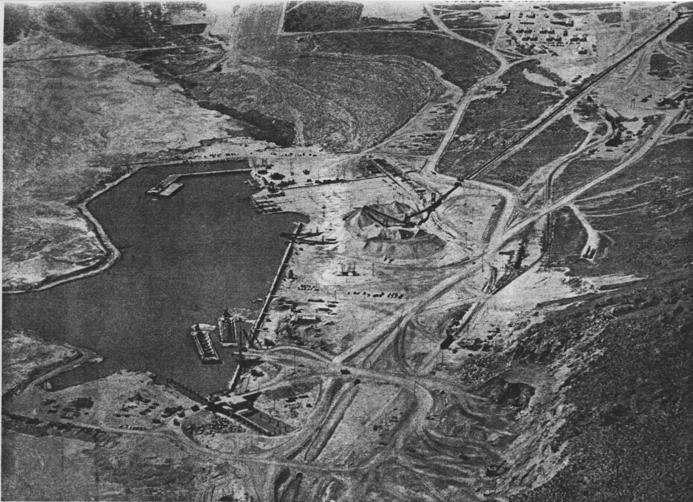
Harbor and material supply center for Great Salt Lake crossing are located on Promontory Point. Belt conveyor at upper right brings 4,200 tons per hour of sand and gravel to storage near waterfront. Barges secure rock from trucks loaded at principal quarry in foreground. Deck barges are loaded at dock at lower left. Ways where barges were assembled are at upper center, and pier for general service is on far side of basin.
