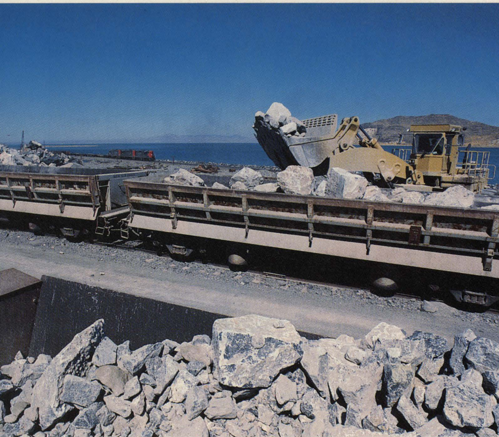
BOULDERS to armorplate the fill are loaded into 38-car train (above) as its motive power switches out piling for bridge construction at Lakeside. Once upon a time 2000 box cars, stripped of running gear, were sunk along the main fill to provide such protection from the lake's vagaries. The boulder-armored fill, in turn, protects the passage of the revenue traffic, such as a westbound CHOAT (Chicago-Oakland trailers) on September 7, 1986, west of Lakeside (below) on partially finished Strongknob fill.
