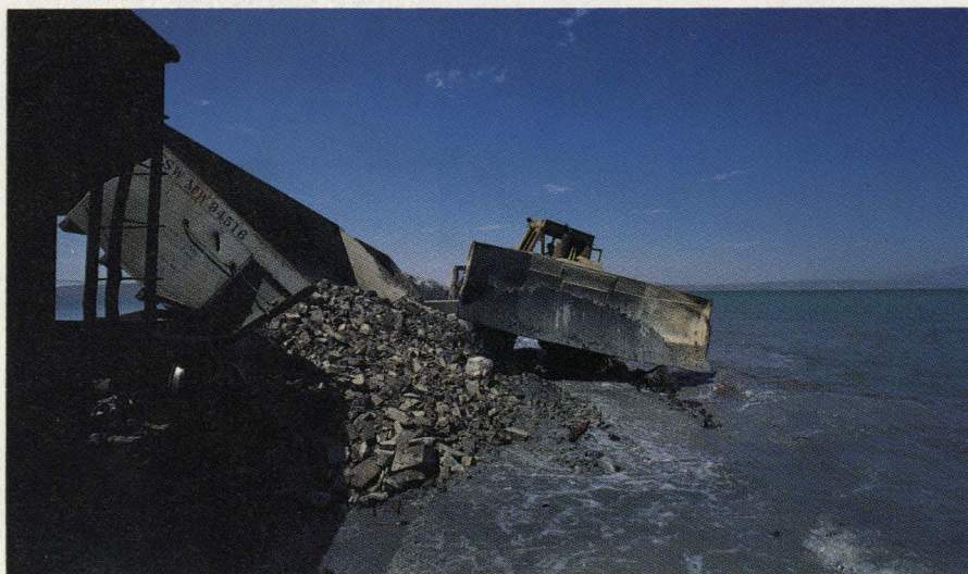
WIDE-BLADED BULLDOZER assists in spreading load of another 68-car work train into blue waters of Great Salt Lake. More than 2 million tons of rock and fill were needed to protect fill from latest lake onslaught. Building the fill originally in 1959 required the equivalent of material used in building three Grand Coulee Dams.
