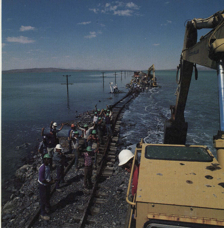
THE BIG DAY, August 4, 1986—and the Bear and his track foreman, Tony Martinez, standing under white Milepost 727, wave dozers, sidecasters, and backhoes in to close the last gap in Strongknob fill, ending isolation from the 727 miles' worth of Overland Route to the west. Rails will be joined August 11; the first mainline trains will roll August 23.
