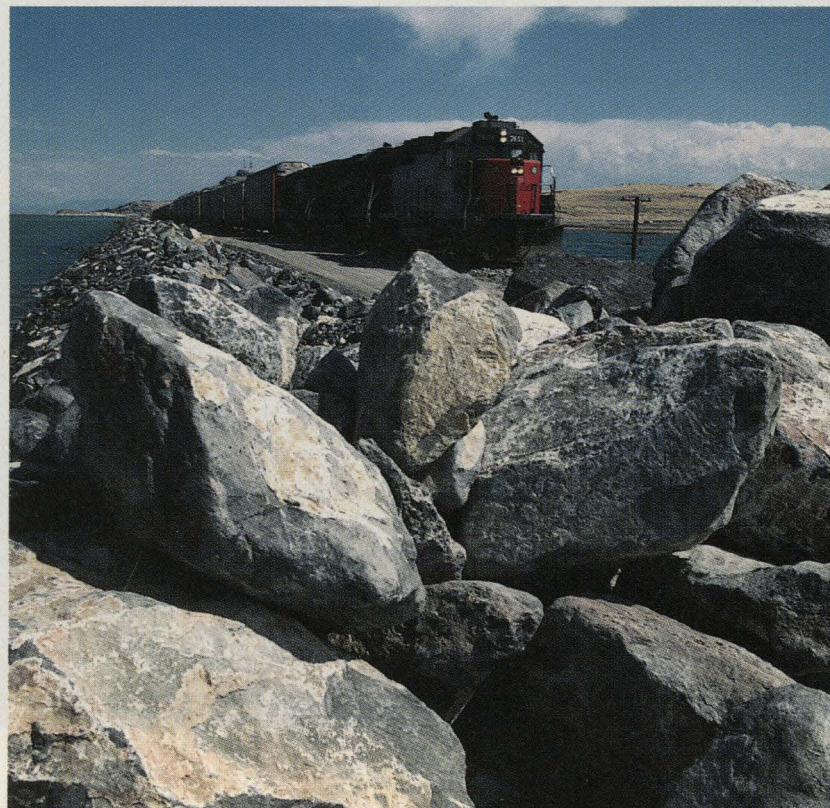
BOULDERS to armorplate the fill are loaded into 38-car train (above) as its motive power switches out piling for bridge construction at Lakeside. Once upon a time 2000 box cars, stripped of running gear, were sunk along the main fill to provide such protection from the lake's vagaries. The boulder-armored fill, in turn, protects the passage of the revenue traffic, such as a westbound CHOAT (Chicago-Oakland trailers) on September 7, 1986, west of Lakeside (below) on partially finished Strongknob fill.
