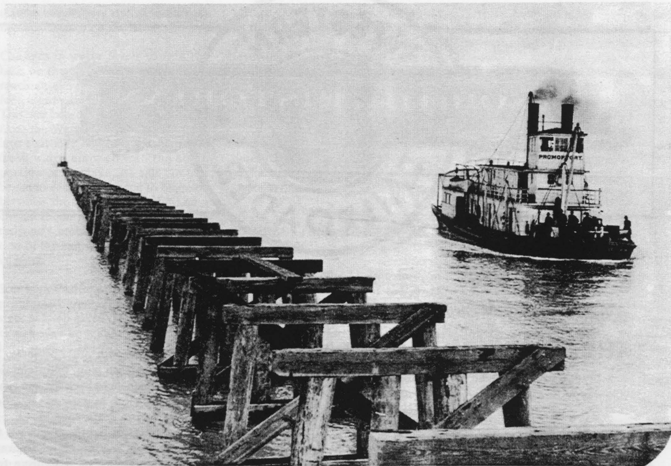
The sternwheeler Promontory , part of Southern Pacific's Great Salt Lake "fleet" steams alongside a temporary trestle during construction of the Lucien Cutoff. (California State Railroad Museum, Sacramento.)
