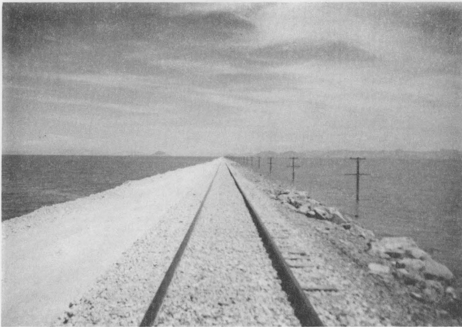
Restored fill between Hogup and Lakeside after storm of June 6, 1986.
