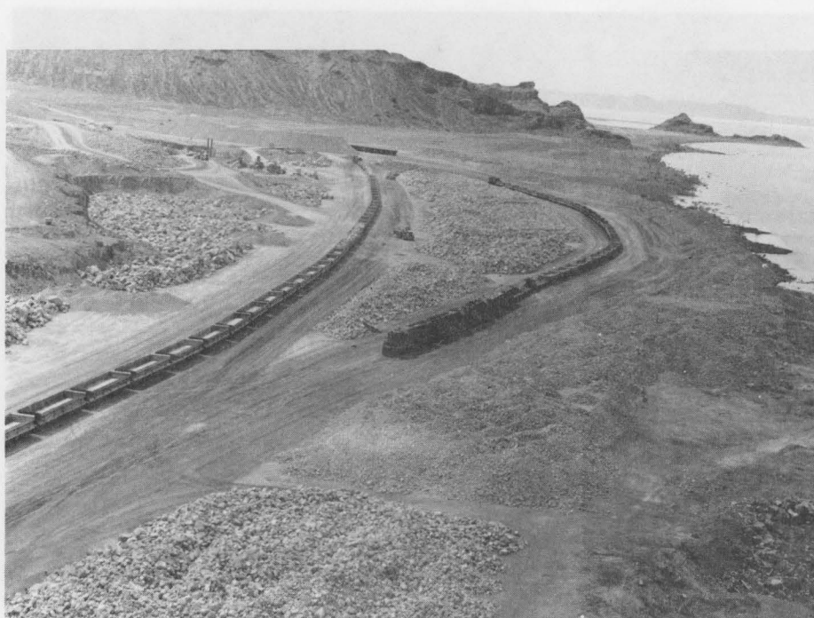
Work trains loading fill and riprap material at Lakeside Quarry.
