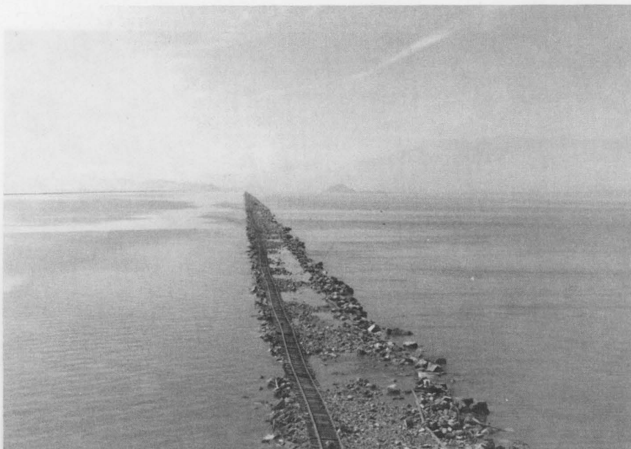
Typical damage as the result of the storm of March 28, 1987, on the Great Salt Lake Fill, looking west to Lakeside.
