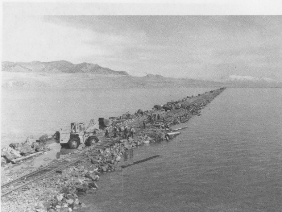
Track workers preparing track to allow passage of work train to dump ballast and fill after storm of March 28, 1987.
