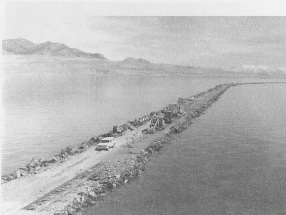
Surfacing gang working behind westward work train after storm of March 28, 1987.
