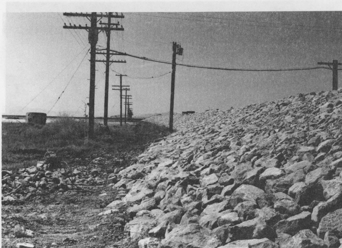
Finished slope protection in the vicinity of Groome in connection with the West Desert Project.
