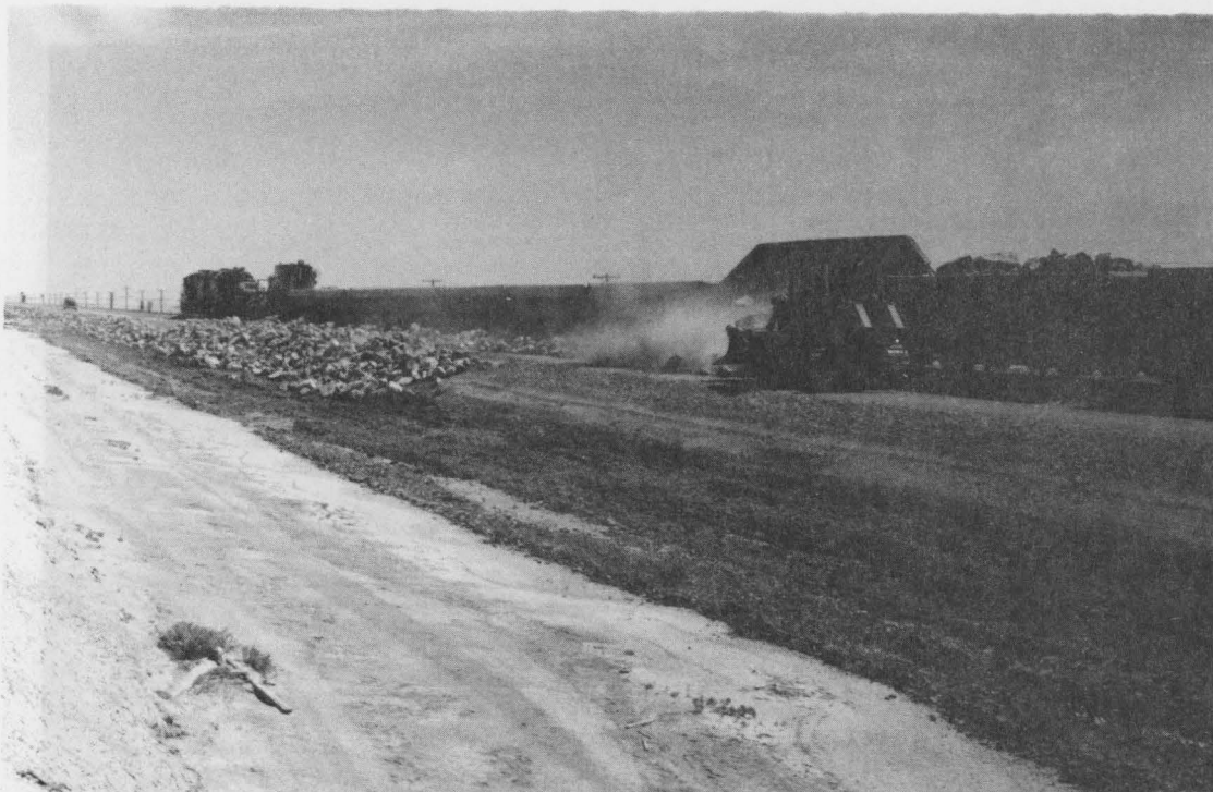
Work train unloading slope protection rock in the vicinity of Lemay in connection with the West Desert Pumping Project.
