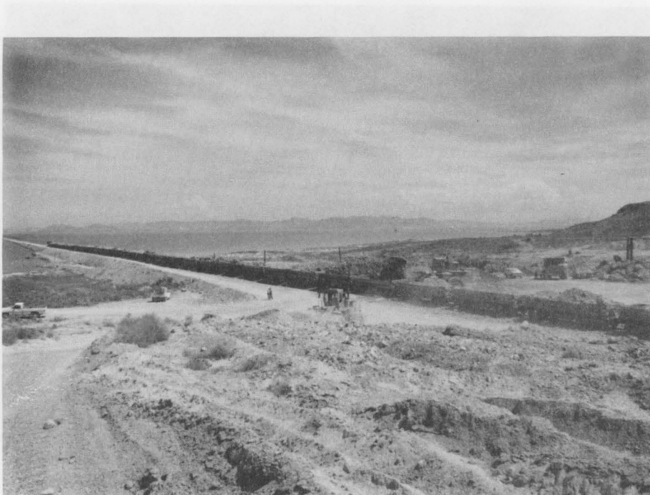
Eastward work train loading at Hogup with fill material for repair work after June 6, 1986, storm.
