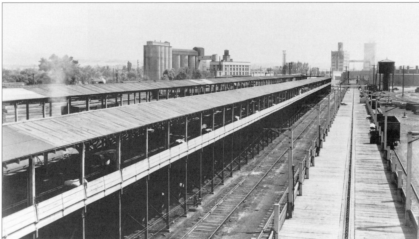
Shown here are the three ice docks of Pacific Fruit Express. The ice dock along the right side of the photo, shown without a roof, was used mainly for perishable traffic originating at Ogden, and was served by a stub-end track. In the distance are the Albers Brothers Milling Co. mill and the Sperry Flour Co.'s mill, both major rail customers. (Pacific Fruit Express, California State Railroad Museum Collection)
