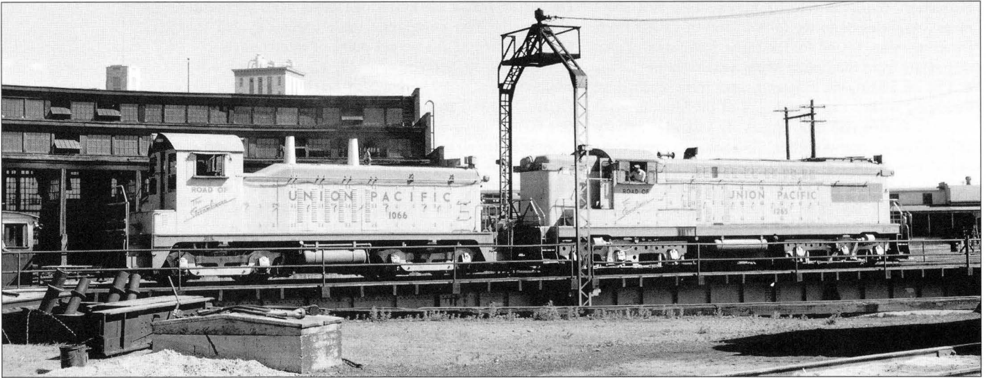
The 135-foot turntable at Ogden also accommodated two diesel locomotives with ease. Here, on June 20, 1959, UP 1066, and UP 1265 share the ride. The 1066 was one of 96 Electro-Motive model NW2s purchased by UP between 1940 and 1948, several of which worked in Ogden. The 1265 was one of six Baldwin model AS-616s purchased by UP in late 1951 for use as heavy switchers in the railroad's new hump yards, and for flat switching at Ogden. (Emil Albrecht, James W. Watson Collection)
