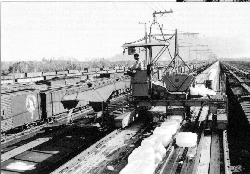
The 1954 completion of a new icing dock for Pacific Fruit Express at Riverdale Yard included three Preco automatic icing machines. These machines traveled the length of the ice dock on rails mounted to the outside edges of the dock. The Precos were able to swivel from one side to the other, allowing the re-icing of cars on either of the two 110-car tracks. (Union Pacific Museum Collection, Negative 38105)
