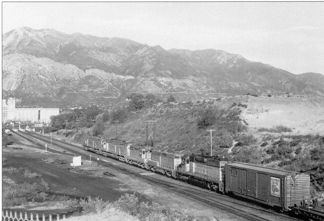
The completion of the Sand Ridge Cutoff in 1906 made Union Pacific's entrance into Ogden from the west much less complicated. In this view we can see the depth of the cut through the sand ridge, along with the bridges at Bridge Junction. There are actually four bridges, the three visible and a fourth bridge for the Shasta Track just to the left of the other three. The name Bridge Junction comes from the junction between the Oregon Short Line-owned cutoff and the OUR&D 30th Street Wye, completed at the same time. (Emil Albrecht, James W. Watson Collection)
