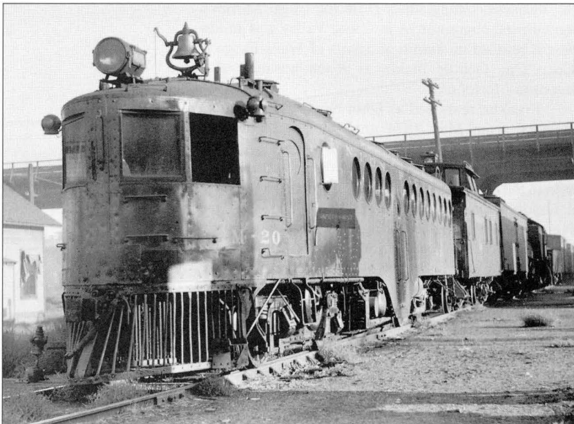
After being assigned to the Ogden-to-Brigham City local, UP McKeen car M-20 sits stored at Ogden on September 7, 1936, awaiting another assignment. McKeen cars were built by UP at its Omaha, Neb., shops from 1905 to 1908, when the McKeen Motor Car Co. was organized to manage the growing market for self-propelled cars and matching unpowered trailers. By 1920, the new Electro-Motive electric transmission cars were outselling McKeen's mechanical transmission cars, and the company was dissolved. M-20, shown here, was completed in 1908 and retired by UP in 1944. (Otto C. Perry, Western History Department, Denver Public Library, Negative OP-19470)
