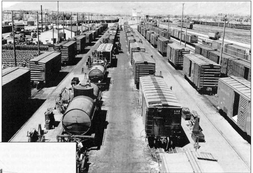
In 1954, UP completed a new four-track car repair facility as part of the expansion of Riverdale Yard. The new facility was equipped with the most modern features, including a work area fully paved with concrete, and a 50-ton traveling crane (from which this photograph, looking north, was taken), and plenty of space for material storage, with room for future expansion. (Union Pacific Museum Collection, Negative 43382)
