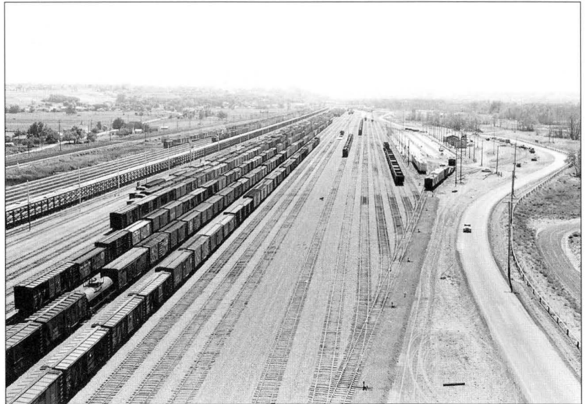
The new Pacific Fruit Express ice dock at Riverdale stretched almost the entire length of the yard. Shown here along the left center of this photo in September 1954, the ice dock was just recently completed. Also visible at right center is the new Union Pacific car repair track at Riverdale. (Union Pacific Museum Collection, Negative 37492)
