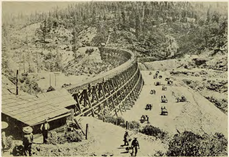
More than 12,000 Chinese workers were used to help build the Central Pacific. Pictured is 1,100-foot trestle over Secrettown Ravine, about 64 miles east of Sacramento, Calif.
