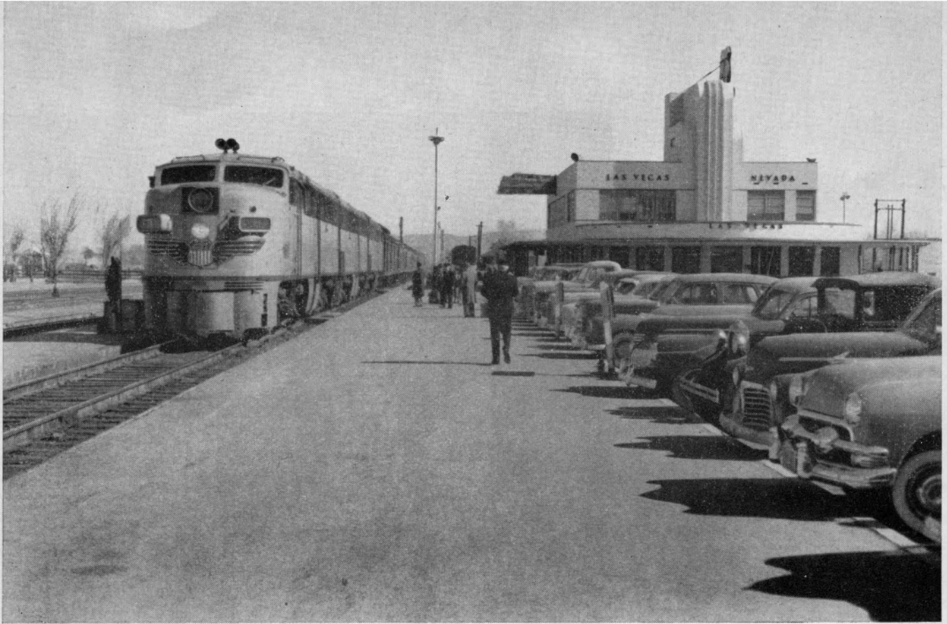
Las Vegas, the end of your trip. This is an early-morning scene of the Union Pacific's ultra-modern passenger station, with No. 3, the west-bound Uahn, arriving behind 6000-horsepower Alco-GE diesel No. 605. Las Vegas is the major terminal between Salt Lake City and Los Angeles.
