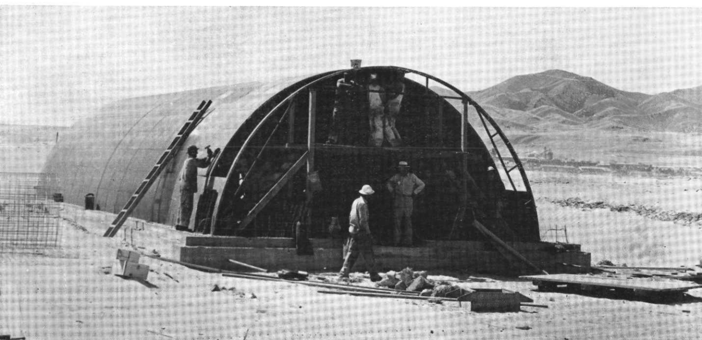
Storage igloo under construction.
