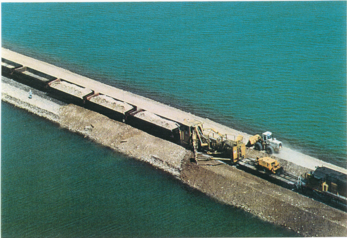
Two 40 car unit trains of 100 ton, 50 Cubic Yard Air Dump cars hauled material to the project site. The material was side dumped and initially pushed away from the tracks with a Jordan Spreader.
