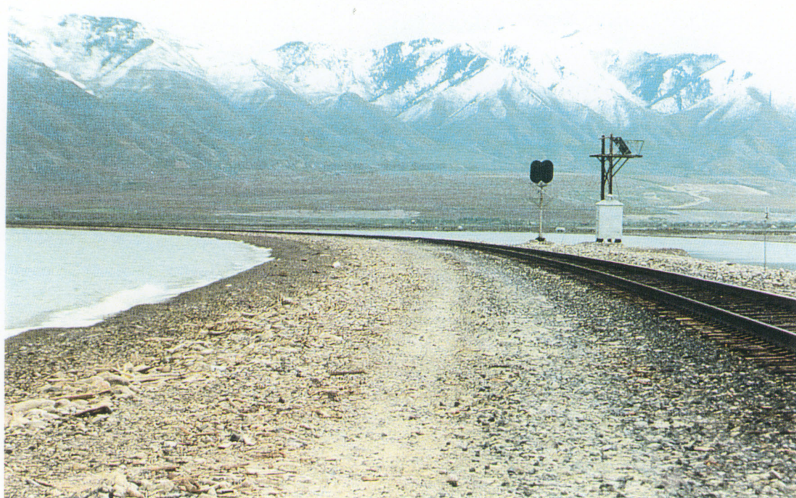
View easterly of beach after all of the material has been pulled out into the lake by wave action to 6:1 slope.
