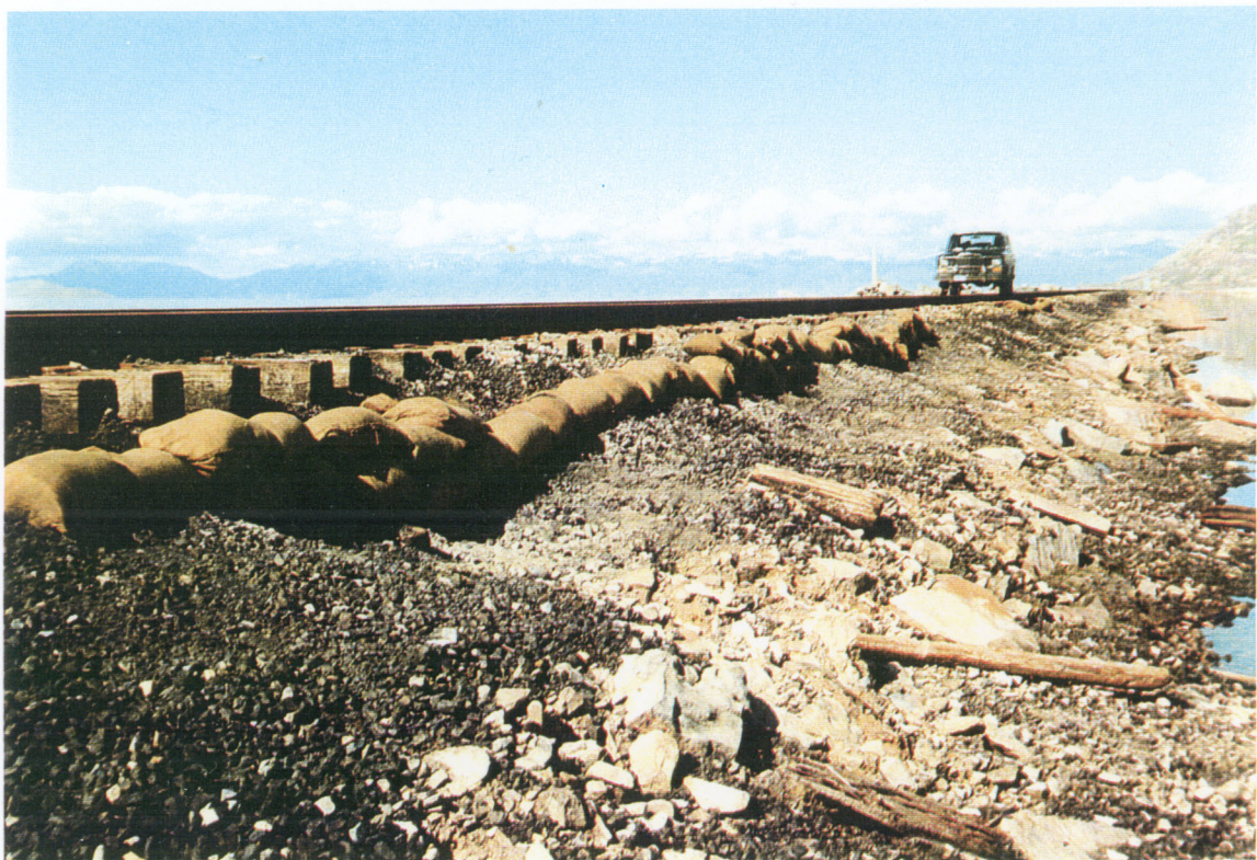
Taken prior to the beach project, this photo shows an example of sandbagging in an attempt to stem severe erosion caused by wave action.
