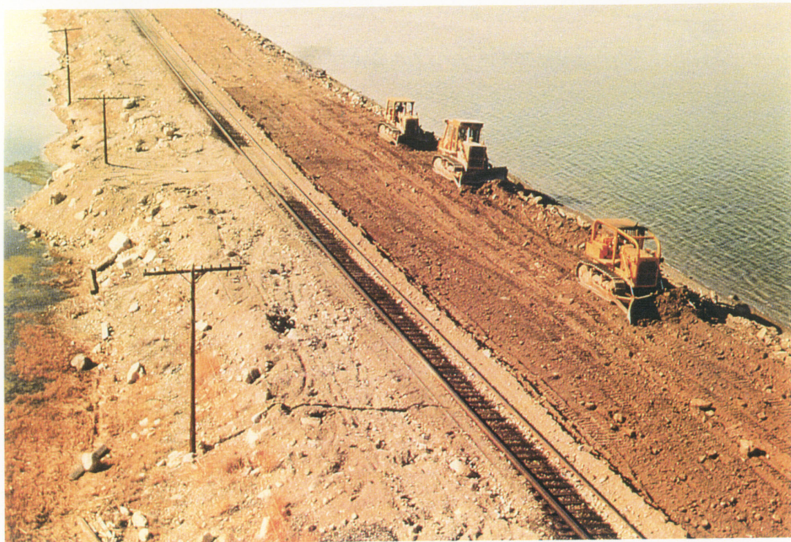
Bulldozers were used to widen the embankment and extend the beach into the lake.
