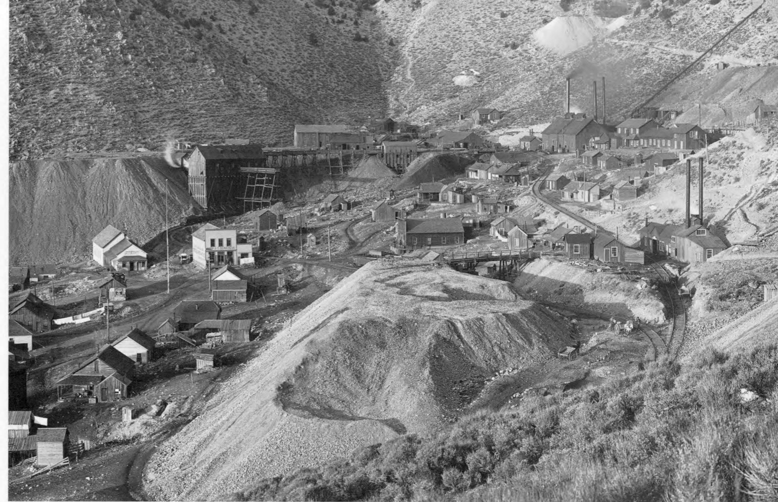
Visible in this 1905 view of the Mammoth Mine is the New East Tintic's upper line and spur to the Mammoth's ore bins at the left. In the center distance, at the upper end of the line is the New East Tintic's engine house, right up against the hill side. - Shipler Photo, Utah State Historical Society Collection
