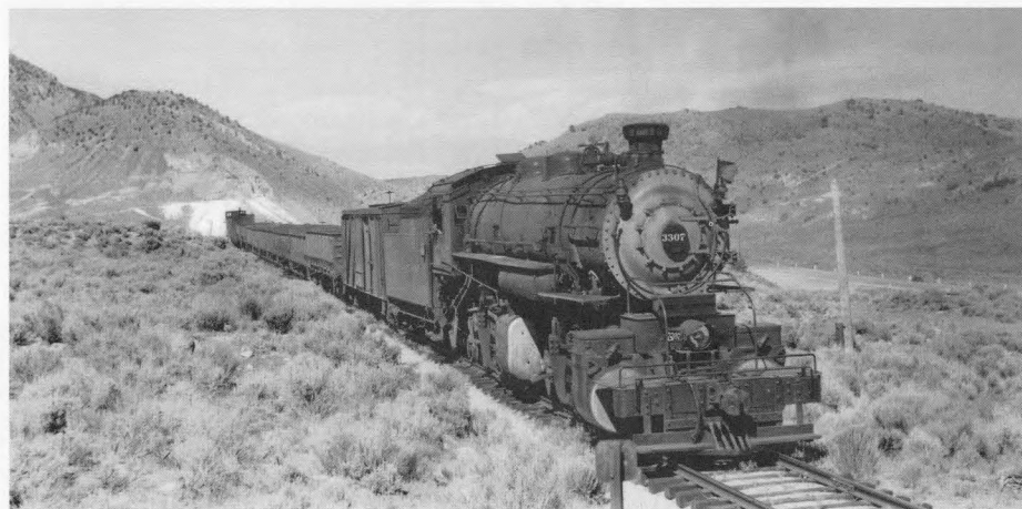
The Tintic Range Railway became D&RG's Tintic Branch as part of a system wide reorganization, on July 31, 1908. By the early 1940s, D&RGW operated into the Tintic district on a three-days-per-week basis, returning to Provo on the other three days. Here, D&RGW 2-6-2 3307 arrives at Eureka on July 5, 1940, having just come up Pinyon Canyon by way of the new line that replaced the branch's famous "Double Circle" but with a steeper grade that required larger motive power. - R. H. Kindig Photo, Don Strack Collection
