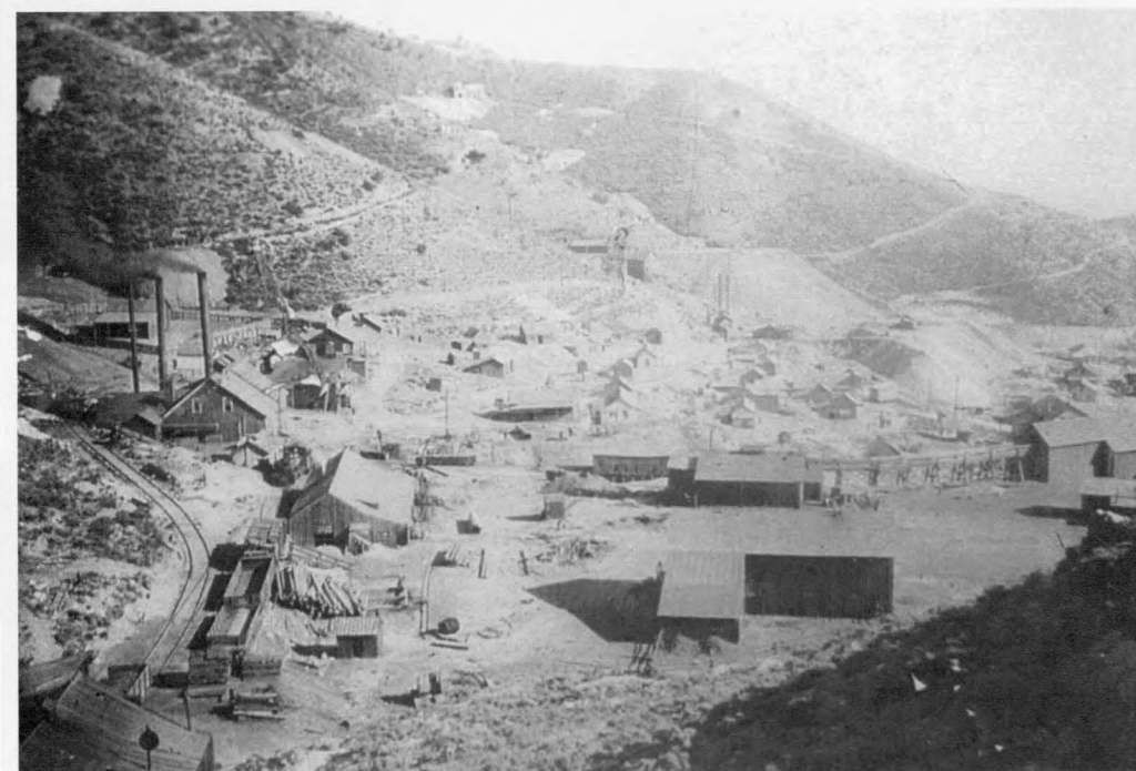
In this view of the Mammoth mine, the ore bins are seen to the right. The New East Tintic's engine house is visible at lower left, and the road's Shay can be seen adjacent to the mine's power house. - Tintic Historical Society Collection
