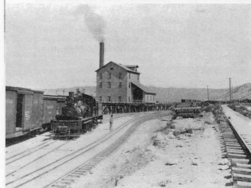
Dual-gauge Eureka Hill trackage is also visible in this 1908 view of the Tintic Smelting Co. where a Eureka Hill narrow gauge Shay is at work. - Sam Bass Collection
