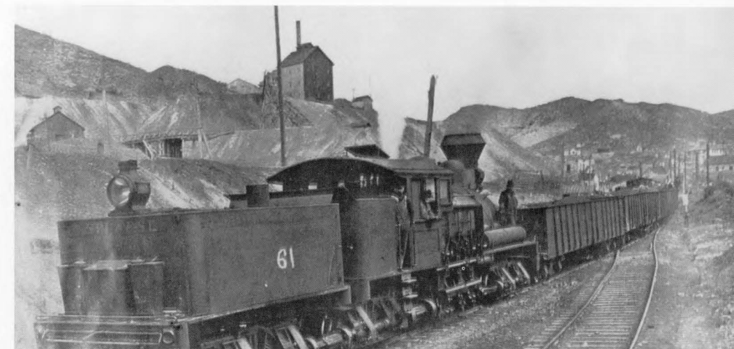
By 1907, the San Pedro, Los Angeles & Salt Lake had bought a third Shay locomotive to operate the Tintic branches. This large 80-ton locomotive was put to work immediately, and is seen here in 1909 easing a cut of loaded cars past the Bullion Beck mill in Eureka, down to the Eureka Branch's mainline connection at Tintic, three miles to the west. - Palmer Photo, Don Strack Collection
