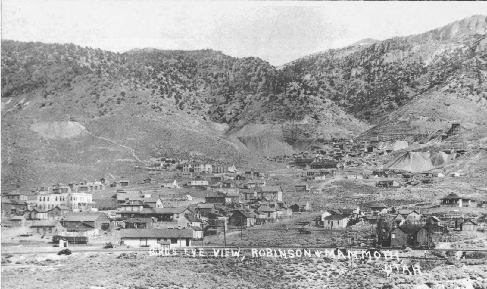
The Mammoth depot is seen in this view just above the word "Bird's" in the inscription. The Mammoth mine and its large waste dumps can be seen high on the mountain side, and a bit to the right, above the depot. The New East Tintic Railway connected the Mammoth mine and the joint station at Mammoth. - Tintic Historical Society Collection
