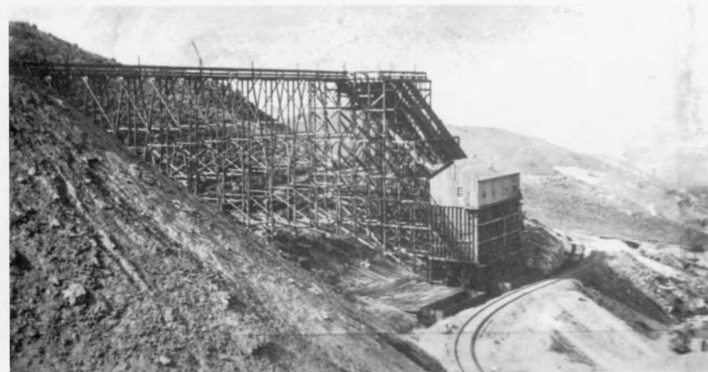
The Gold Chain mine was originally known as the Sioux-Ajax, and in about 1901, the New East Tintic built a spur to serve the mine's new ore bins, which were built right adjacent to the road's mainline. The Robinson mill is visible to the west in the background. - Tintic Historical Society Collection
