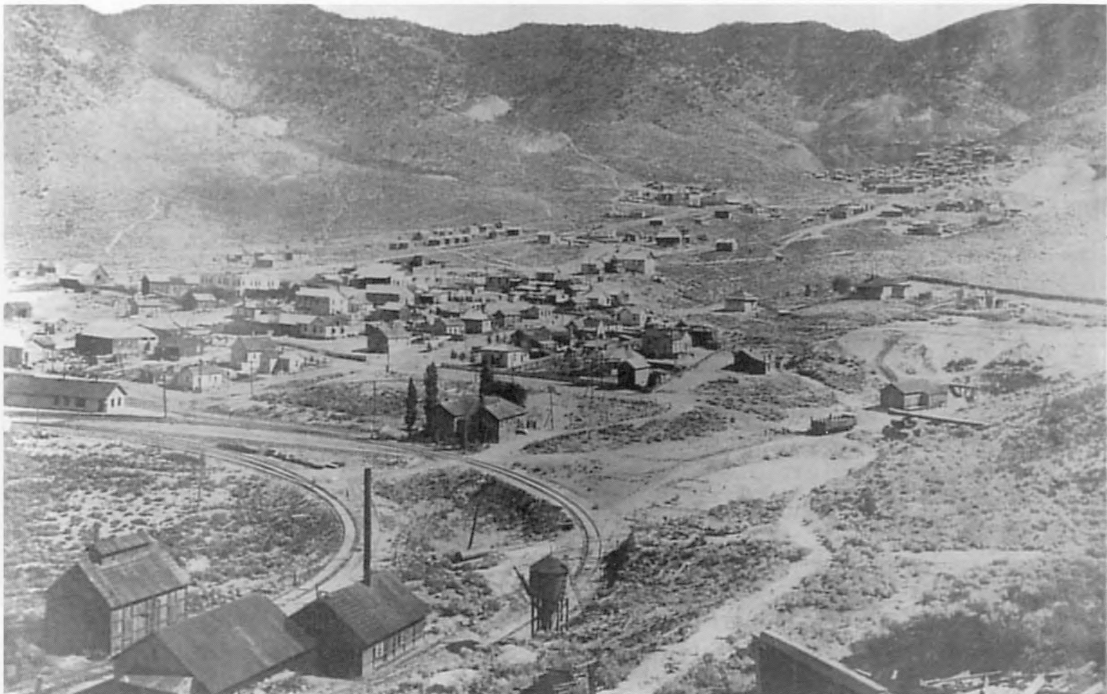
From the Robinson mill, this view shows the joint Mammoth depot at left middle. The New East Tintic's lower line curved away from the depot and began its 6 percent climb to the Mammoth mine seen in the distance at upper right. The Farrel mill is just out of the photo to the right. - Utah State Historical Society Collection
