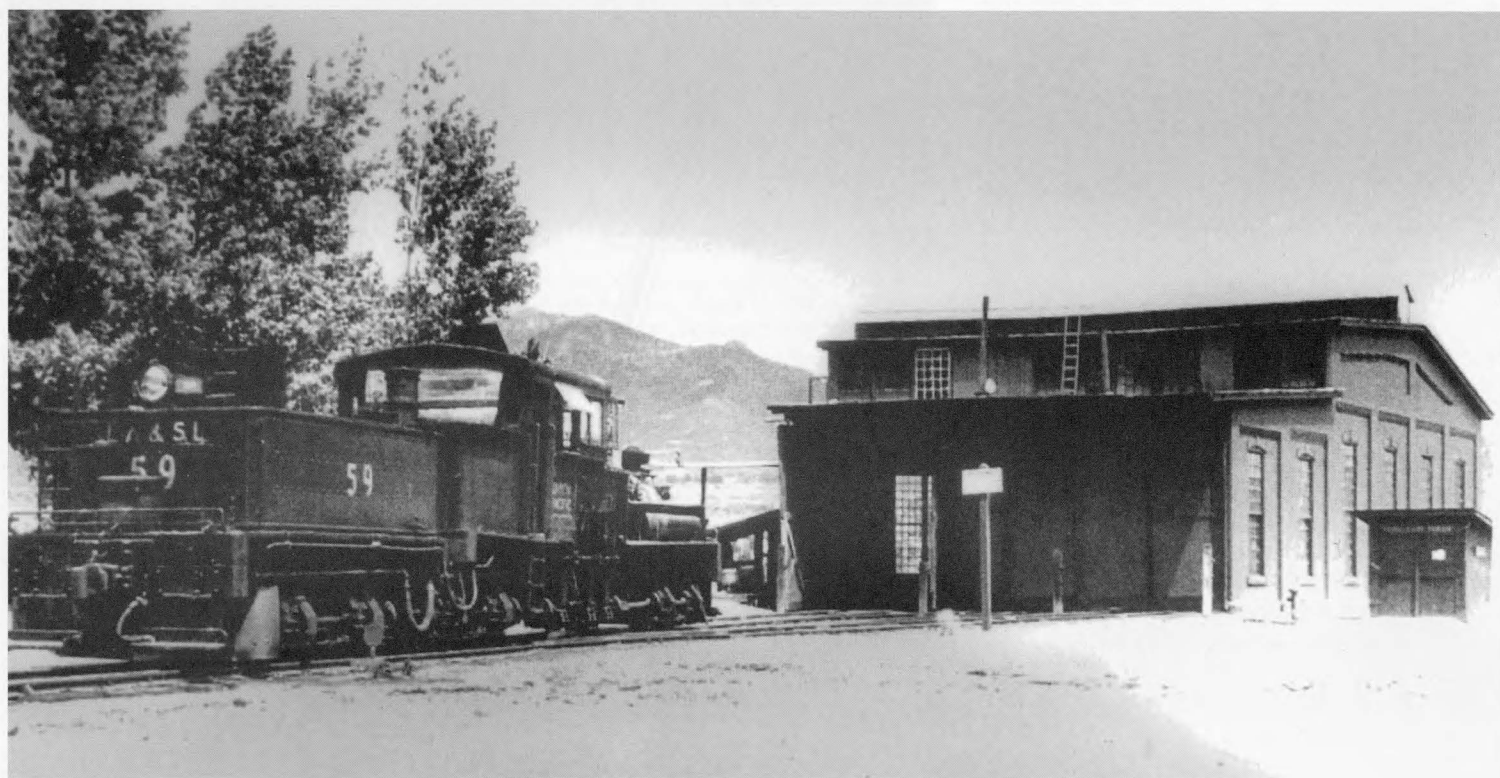
Below: The brick engine house at Tintic was completed in about 1903, and replaced an earlier structure located at the Mammoth mine. The engine house's design matched similar, but larger, roundhouses built at the same time at Salt Lake City, Lynndyl, and Milford. No information has surfaced as to when the Tintic engine house was torn down. - Tintic Historical Society Collection
