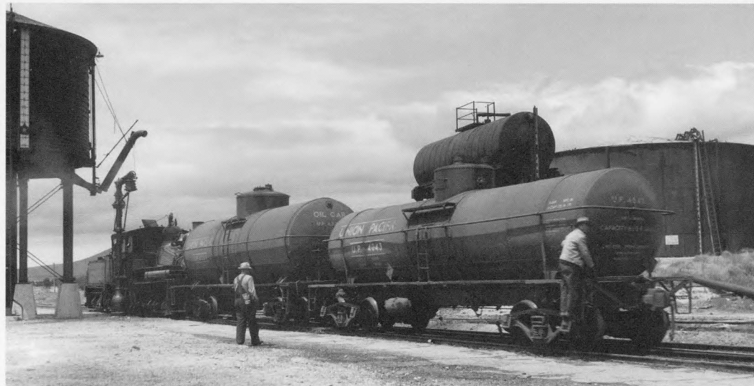
LA&SL 59 switching at Tintic on June 21, 1947. The LA&SL Shay locomotives assigned to the Tintic branches were oil fired. On a regular basis, oil arrived and had to be switched to the oil loading spur to fill the storage tank in the background. Another oil stand at Tintic also served to top off mainline trains. - Two photos, F. J. Peterson Photo, Donald Duke Collection
