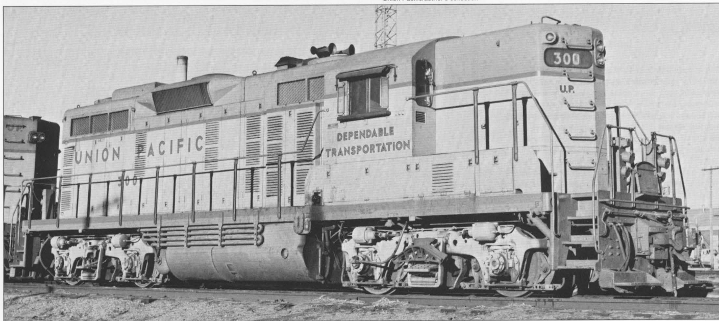
UP 300 as it appeared with the EMD turbocharger installation done by EMD. The second group of six units that were sent to LaGrange to be rebuilt with the EMD design did not acquire the same regular GP20 features as the first three. They can be identified by the same arrangement of the louvers on the carbody doors in the center of the carbody, under the dynamic braking bulge and grille, along with the addition of a three-foot radiator fan and small winterization hatch, a feature that all nine LaGrange-modified units received. The units modified by UP at Omaha did not gain the extra louvers, which were the same on both sides. Laramie, Wyo., October 29, 1968.
