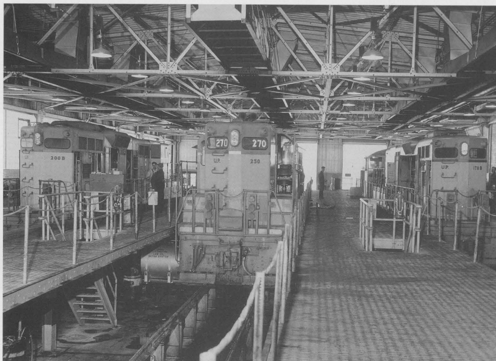
Tracks 1, 2, and 3 in the Salt Lake Shop were assigned to running repairs on the railroad's locomotive fleet. These are repairs that can be completed in eight hours or less. In this view looking out the north end, GP9 number 250 is being worked after recently arriving at the head of Train 270, the daily time freight between Pocatello and Salt Lake. Just visible above number 250's coupler is its road number in red 3-inch numerals. Note also the overhead exhaust ventilators. Union Pacific Museum collection 38050
