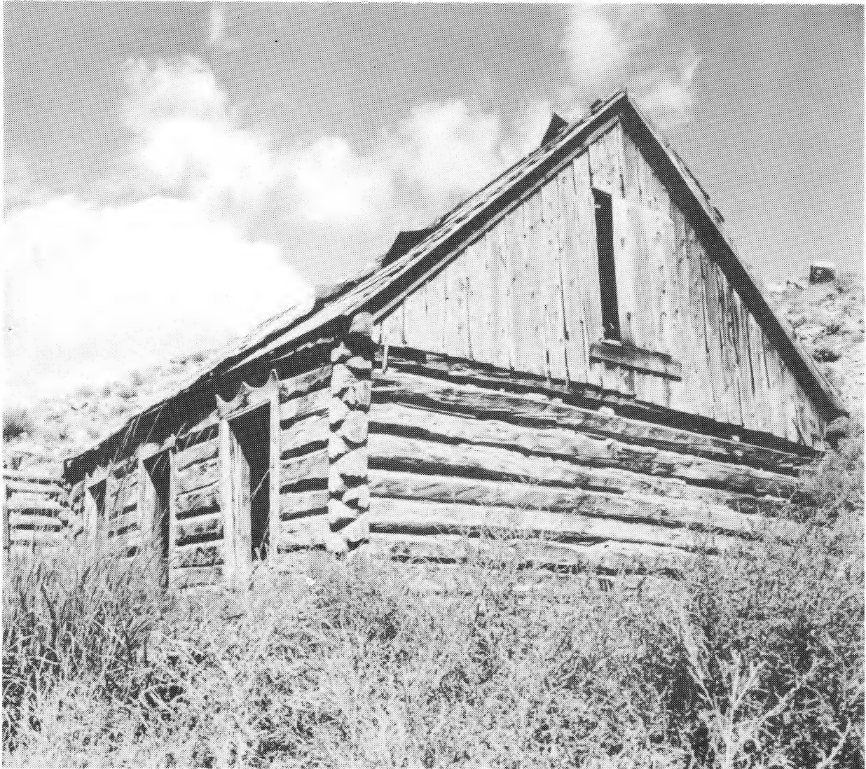
The old post office at Harper yielded a treasure in old stamps a few years ago. The post office, hotel, livery barn and a couple other buildings are all that remain of the old town in Nine Mile Canyon.
