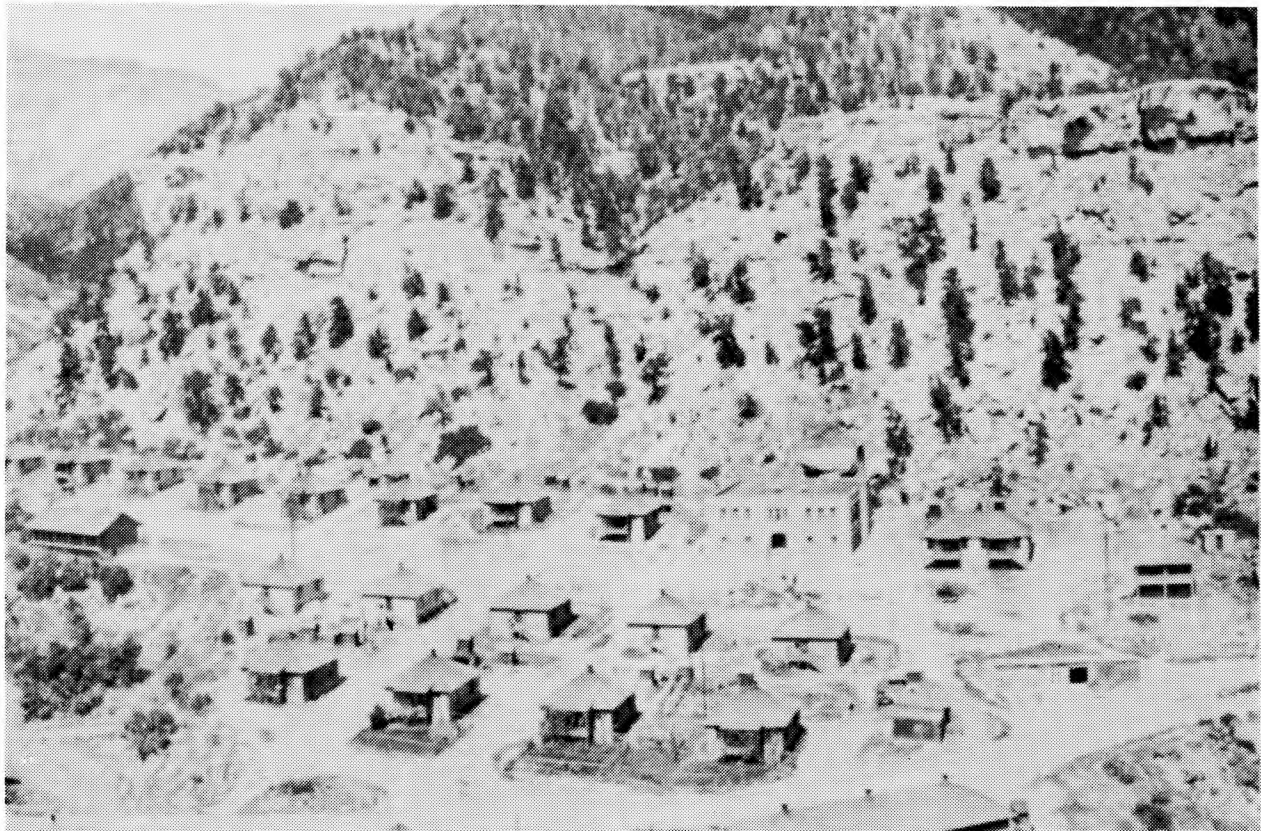
the picture was taken prior to 1945 when indoor plumbing became the vogue.
