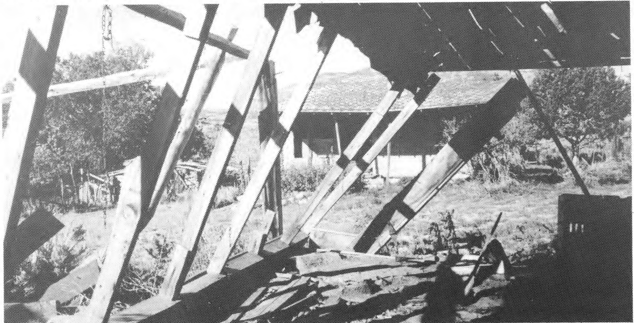
Most of the homes are gone now, but some still stand at Coal City. The wood frame homes are in various stages of collapse
