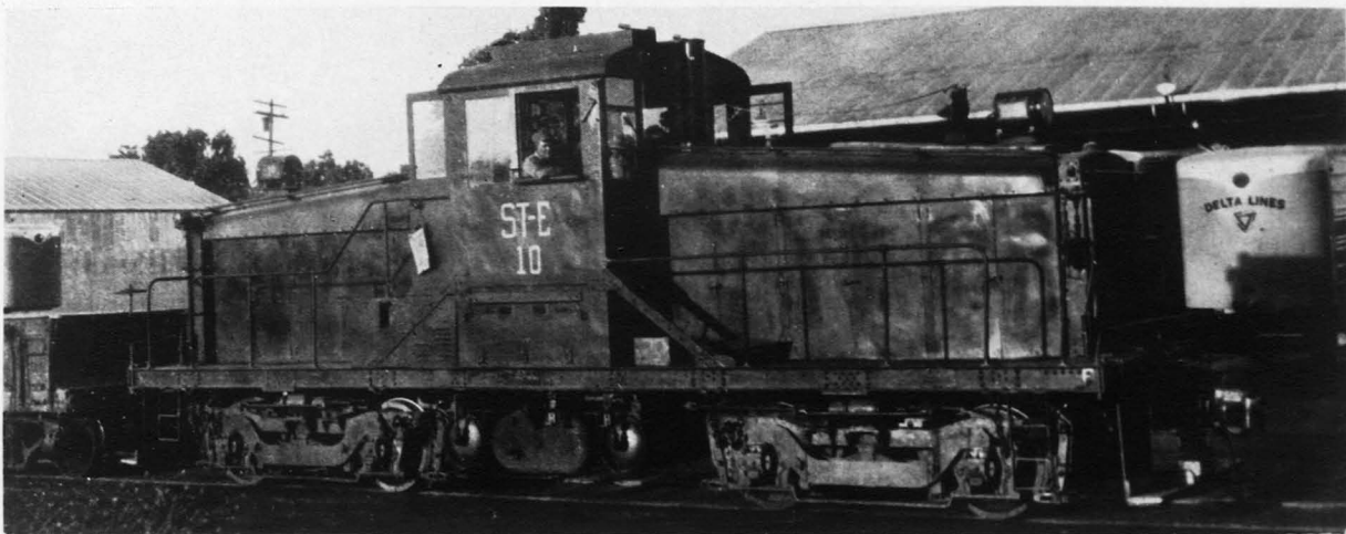
A war-time steeple-cab 450 b.h.p. 58-ton Bo-Bo switcher built by Mid-West Locomotive Works, and purchased as war surplus by the Stockton Terminal & Eastern, California
