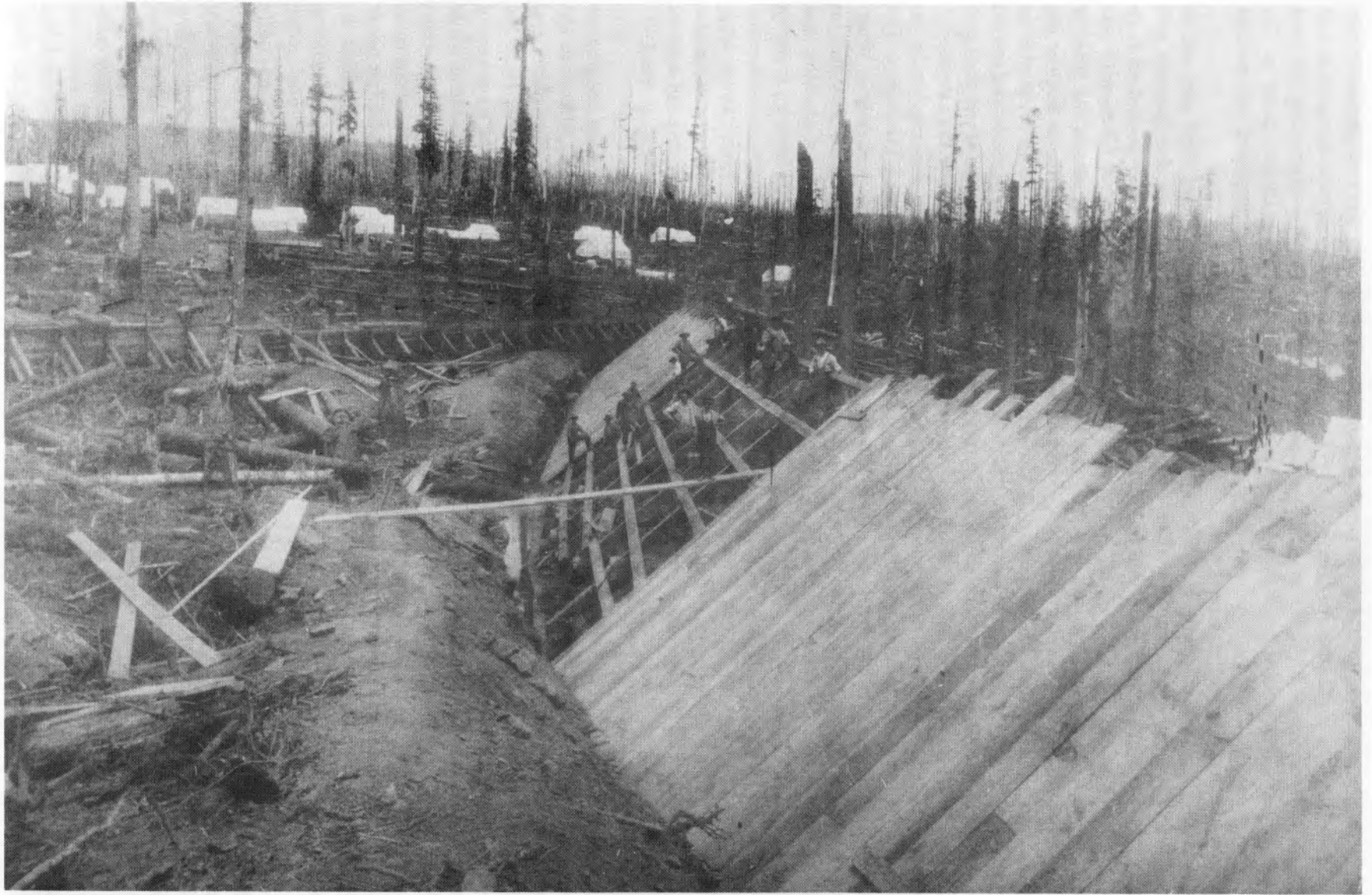
Building a log pond at Mill A or Chenowith, Washington. Constructing a retaining wall on a framework of logs with lumber was easier than trying to move dirt. Judging from the size of the workmen, the timber in the center of the picture may be 40 feet in length. In 1985 an abandoned dam of identical construction was found just south of the Dee millsite. Flume in the background will supply water to the pond and may be used to transport logs since it is rectangular in shape. Lumber flumes of the period were triangular; log flumes square or rectangular. (Courtesy of Clyde Norby.)
