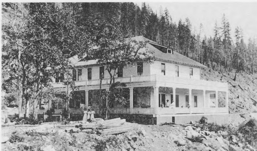
The Dee Hotel was a fixture of the community for many years. It served as a boarding house for company employees and as a guest house for visiting officers of the company. The mainline track of the Mount Hood was located so close to the east side of the hotel guests could almost step off the cars onto the open porch. (Courtesy of Russ Curtis.)
