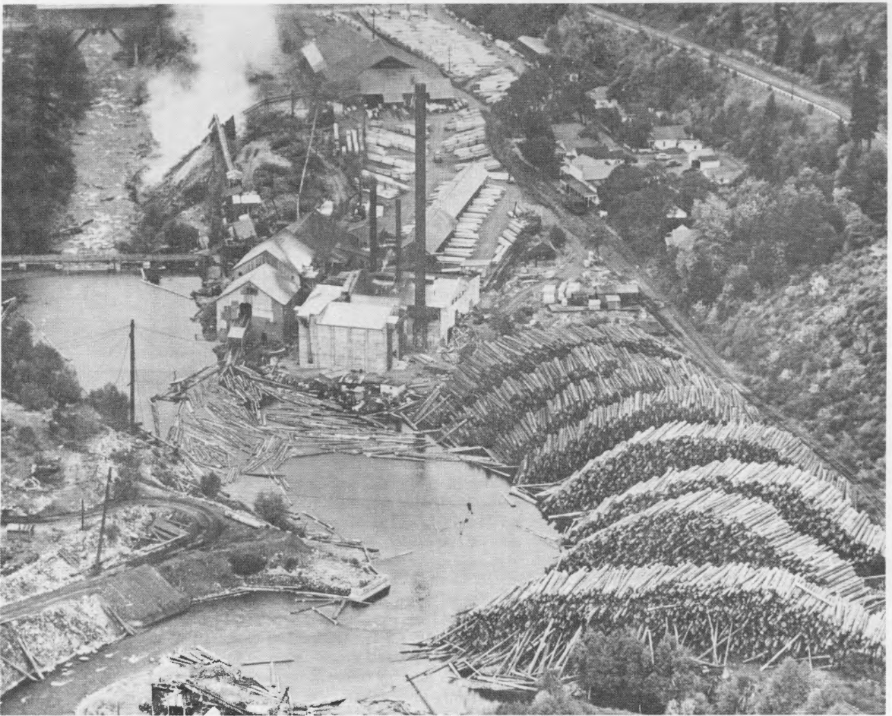
The Dee sawmill about 1950. The logging railroad has been abandoned and the new truck dump is in the lower left. Logs have been decked for the coming winter and the mill was now sawing every month of the year. Using a cable system it was possible to deck logs over 50 feet if desired. In 1941 a similar deck of logs went up in smoke. While making more room for another deck a blasting fuse smouldered, later ignited the dry duff and the blaze reduced 4½ million board feet of logs to cinders. Fortunately the fire was contained and did not spread to the buildings or the extensive lumber inventory. Note the open burn pile. (OHS Neg. 64984.)
