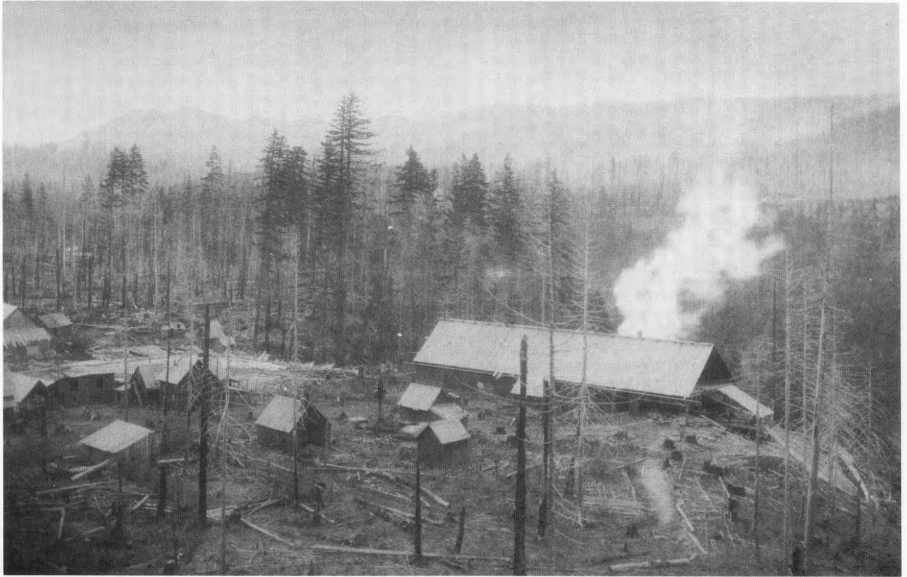
Mill A sawmill in Washington sometime before 1900. Log pond and the wooden dam can be seen in lower left. Rough lumber dropped out of the rear of the mill into a flume that floated the boards and railroad ties to the Columbia River. Mill A Flats are still shown on modern maps. The burned forest around the mill is typical of the period. Most of the timber in the Columbia River Gorge was destroyed by fires caused by settlers, railroads and loggers. No attempt was made to control the frequent blazes. (Courtesy of Clyde Norby.)
