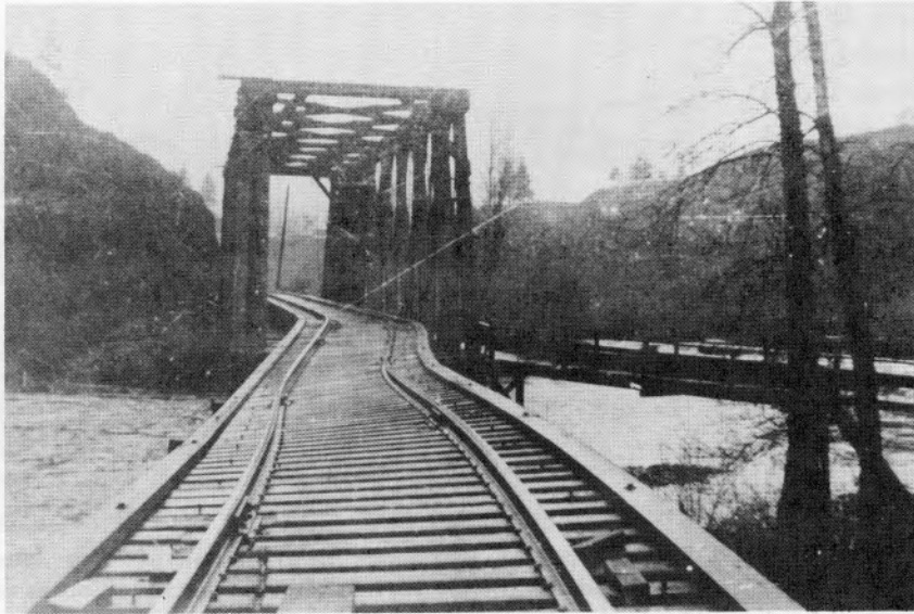
Rampaging waters of Hood River have caused problems for the little railroad on numerous occasions. This particular shift in alignment occurred while the old wooden span was still in use and happened during the same storm that took out track at Collins Creek. (Leland Flint photo.)
