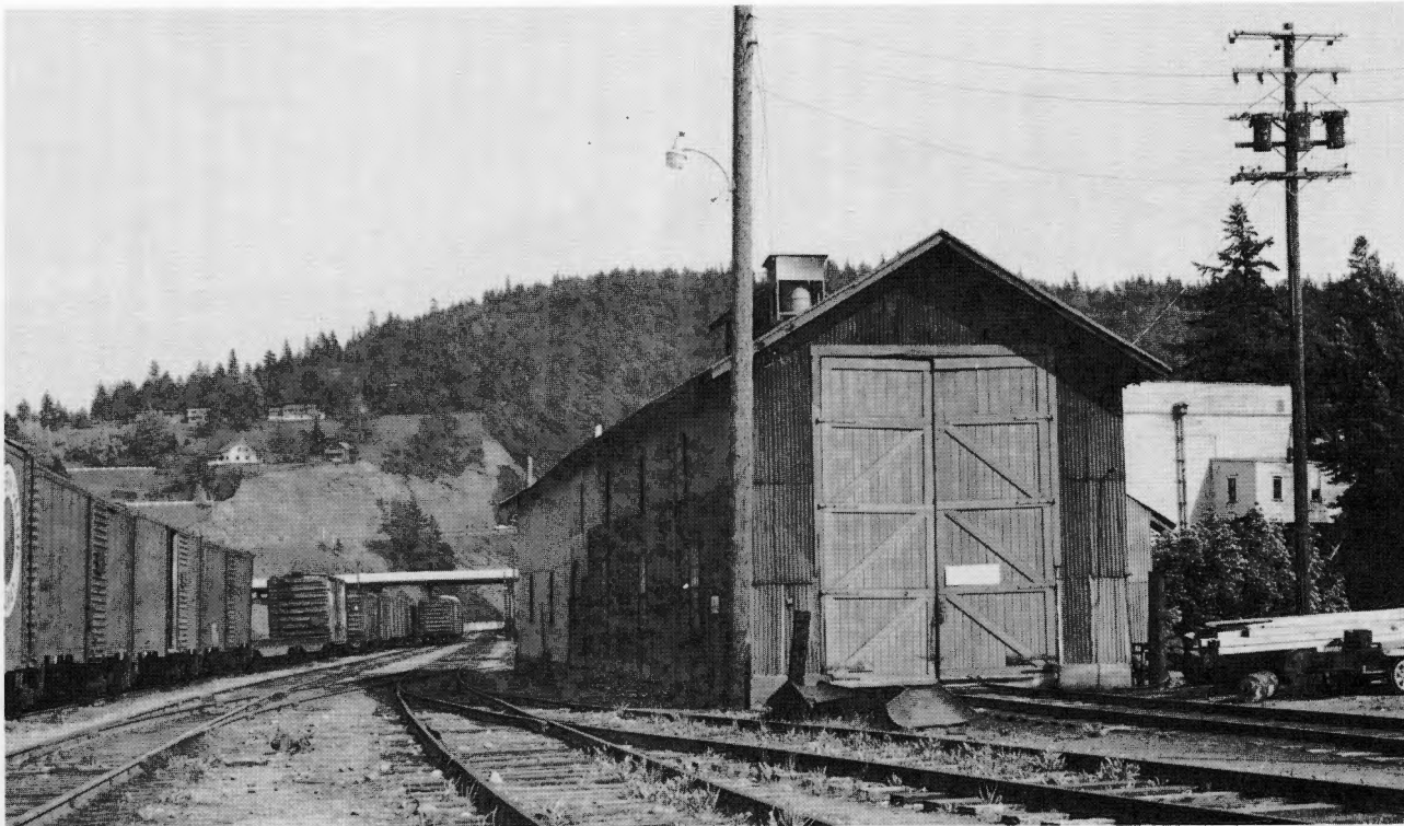
Hood River engine house in the late 1950's or early 1960's. View is east toward Hood River, white overpass is the Highway 35 bridge over the yard tracks and the river. (Courtesy of Donald C. Dietrich.)
