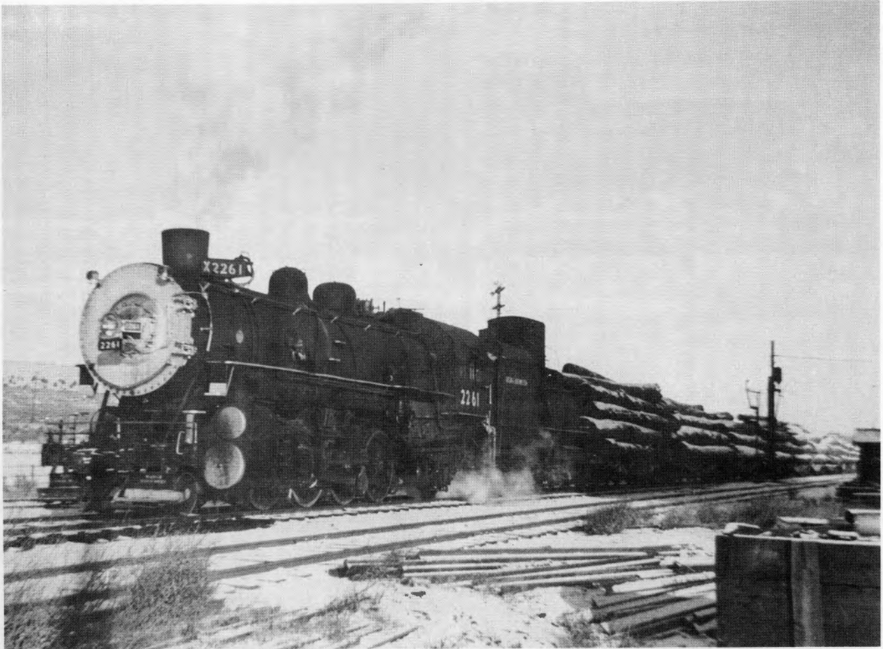
A sister to the ill-fated Mount Hood Number 36. Number 2261 was one of two former Union Pacific 2-8-2's purchased by the Edward Hines Lumber Company for its Oregon and Northwestern Railroad. Although the O&NE was a common carrier its main purpose was to haul logs from the company logging operations at Seneca, Oregon some 60 miles north of Hines. These locomotives were well suited for this purpose and at the rumored price of $10,000 each, a real bargain. (Photo by author.)
