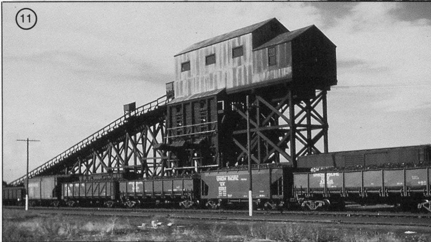
*Photo 2 — Circa 1949: A view of the 230-ton coal trestle from the north, with a feed mill in the background. The coal trestle had two tracks leading up to it, one for loaded cars and one for empty cars, and a hoist pulled the cars up the incline. The trestle could load locomotive tenders spotted on both sides of the structure. One of the feed mills can be seen towering over the loaded coal cars.*
