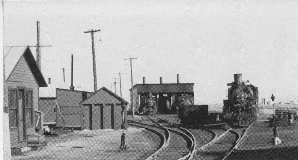
*Photo 7 — Circa 1948: The three-stall enginehouse with what are, likely, four Harriman-standard 2-8-0 locomotives, each with a vanderbuilt tender. The wood gondola is sitting beside the cinder pit.*
